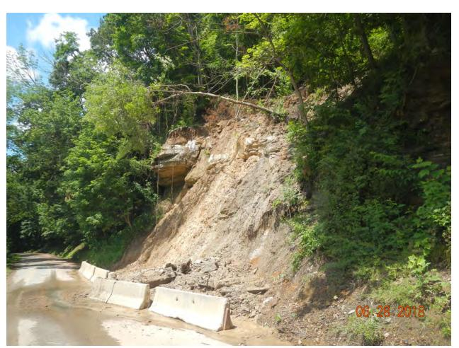
Photo: Landslide pushing into a roadway in Maryland.
