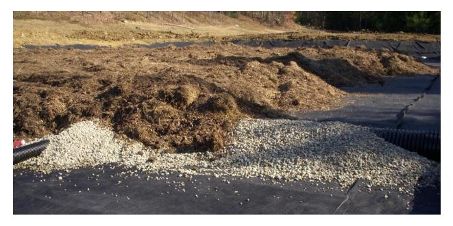
Figure 7: Close up image of effluent collection pipe embedded in rock shown in Figure 5. Image shows spur pipes (bottom left) connecting into the trunk (header) pipe (bottom right).
