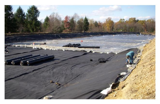
Figure 26: Non-woven geotextile being placed on top of a synthetic liner during the construction of a Bioreactor.
