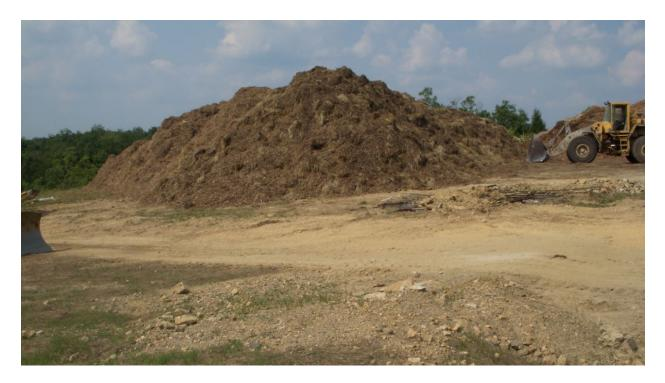
Figure 5: Large pile of Bio Mix (manure, compost, hay, woodchips, limestone) in preparation to be placed in Bioreactor.
