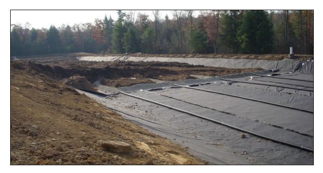
Figure 10: Alternative piping network design. Spur pipes are aligned parallel to the longest dimension of the Bioreactor and the trunk (header) pipe is positioned across the width of the bioreactor. The piping network is embedded in stone to protect the perforations from the overlain Bio Mix layer.
