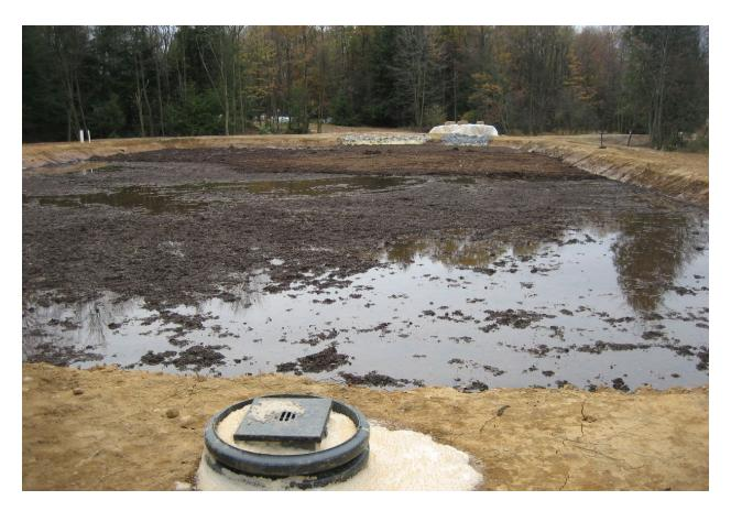
Figure 18: Newly constructed Bioreactor being filled with mine drainage in preparation for a two-week incubation period.
