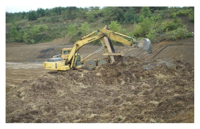
Figure 12: Truck end-dumping the Bio Mix material and excavator trying to carefully smooth out the surface to obtain a uniform thickness to promote a uniform flow pattern. Extreme caution must be used to prevent compaction of the Bio Mix material, which is irreversible.
