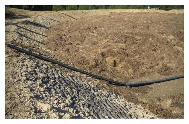
Figure 9: Bioreactor under construction showing effluent collection pipe embedded in rock (bottom right) to be covered by Bio Mix layer. Pipe cleanouts were installed along the side slopes to remove debris if collection piping becomes clogged. Once a common practice, cleanout pipes are now sparingly used because of short circuiting issues experienced by flow along the sides of the clean out pipes.
