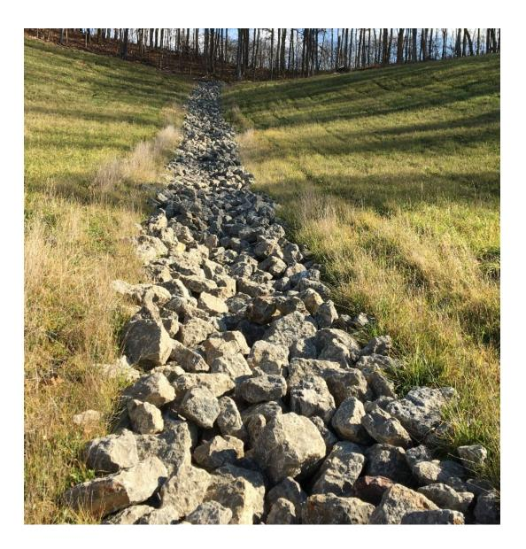
Figure 4: Photograph of Aggregate-lined ditch.
