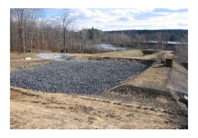
Figure 6: Newly constructed Limestone bed before being filled with mine drainage.
