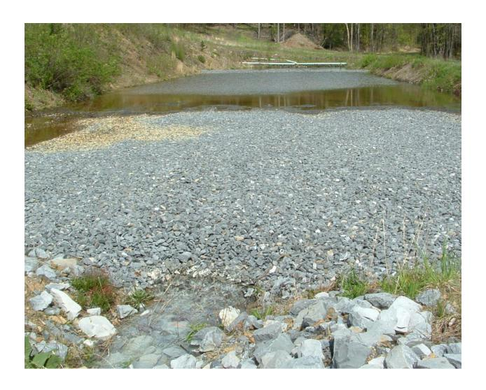
Figure 7: A limestone bed constructed with a focus on easy maintenance and not using a piping network to continuously flush the system to remove precipitates. Water flows into the system from the piping manifold seen in the background and water exits in the foreground.
