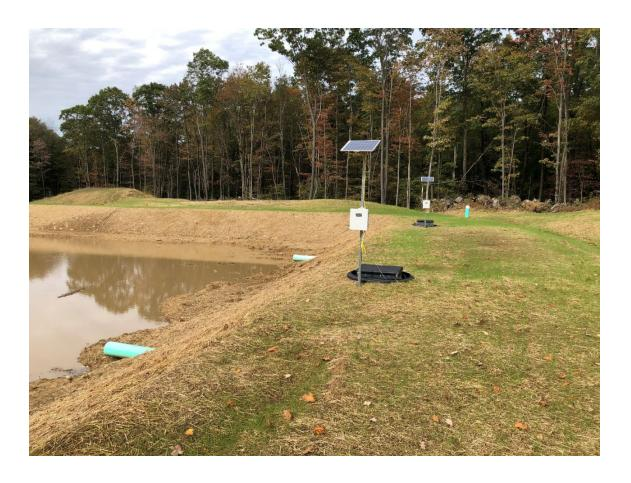
Figure 9: An "Agri Drain Smart" water control structure is shown enclosed by the black corrugated pipe. The solar-powered system can be set using the programmable logic controller (PLC) contained within the white box on the post to drain the limestone bed once a week and for a specified duration. The control box powers an actuator that opens and closes a gate valve to drain (flush) the system contained within the water level control structure in the embankment.
