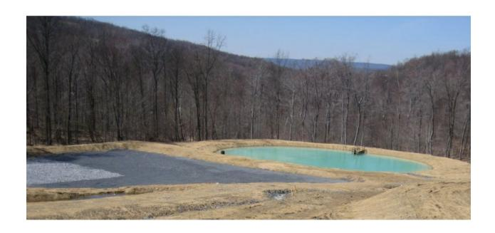
Figure 8: A newly constructed limestone bed (left) constructed with a dosing siphon. The system acts as a batch reactor that fills with mine drainage until a pre-determined elevation is achieved that triggers the dosing siphon to drain the system to a settling pond. The aquamarine color of the settling pond is caused by suspended aluminum flushing to the pond.
