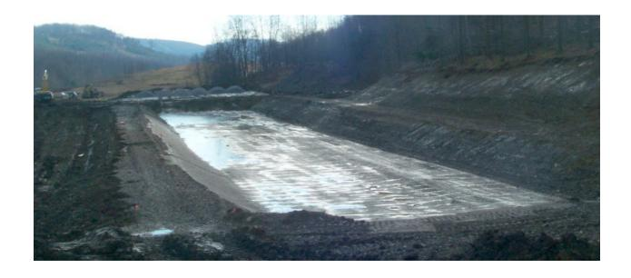
Figure 5: Graded footprint of limestone bed. Piles of limestone seen in the background.
