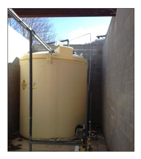
Figure 5. Photo of a HDPE Double-Walled dose tank.
