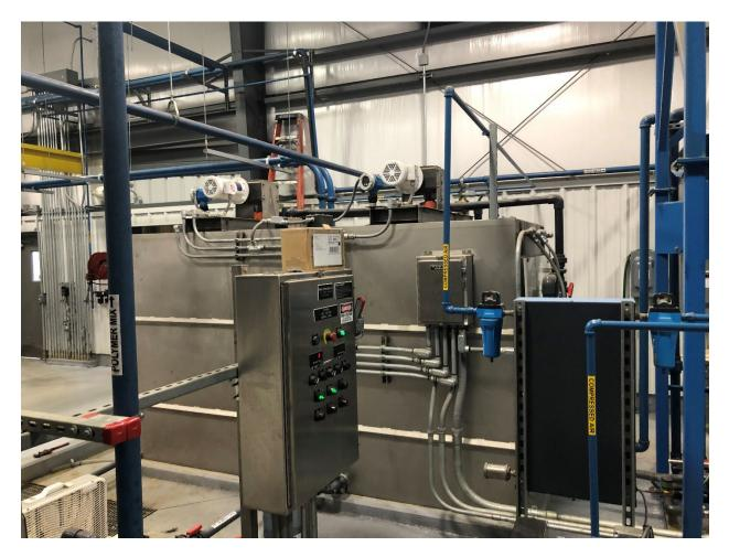
Figure 5. Stainless steel blending/aging tank for made down dry polymer solution with mixers mounted over the tanks.
