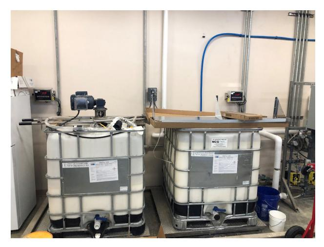
Figure 2. Emulsion polymer totes (275-gallon) for use at a mine drainage treatment facility in Pennsylvania.
