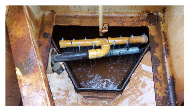
Figure 8. Application point of polymer into the mine drainage at a treatment facility.
