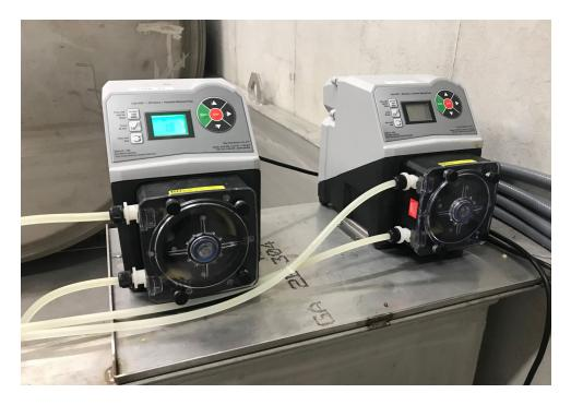
Figure 7. Photo of two pumps as part of the dosing skid component of a dry polymer automatic system.
