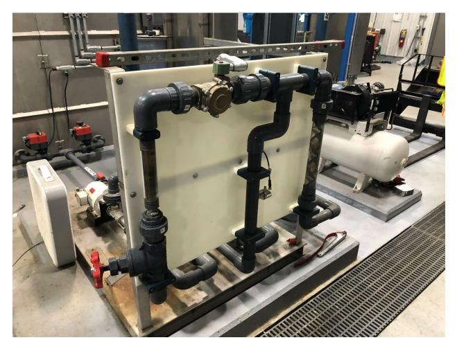
Figure 6. Pumps and inline static mixers for mixing the made down polymer solution with push (dilution) water prior to addition to the mine drainage source.
