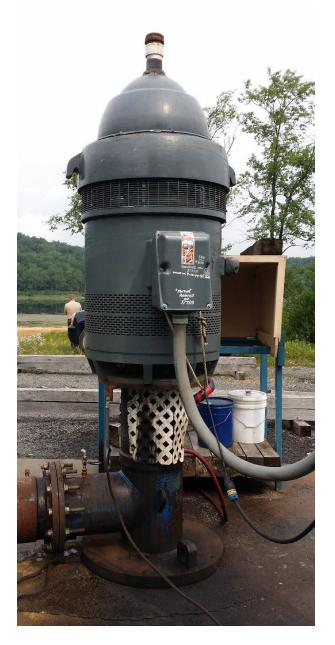
Figure 1. Vertical Turbine Pump at a mine site in West Virginia used to pump water from an underground mine pool to the surface for treatment at an active chemical treatment facility.
