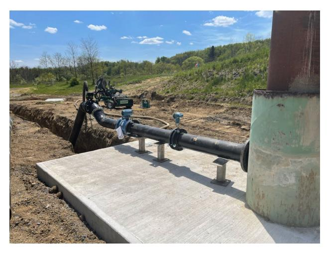
Figure 3. New installation for a Vertical Turbine Pump showing concrete pad, surface borehole casing, inner borehole casing and conveyance piping connection fittings at a mine site in Pennsylvania used to pump water from an underground mine pool to the surface for treatment at an active chemical treatment facility.
