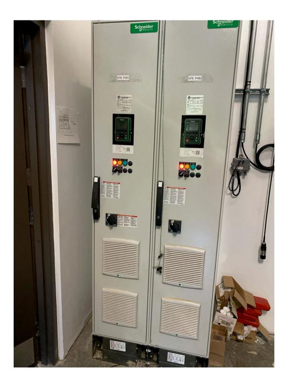
Figure 4. Soft Start/VFD units (2) for two 150 HP submersible mine water withdraw pumps at a mine site in Pennsylvania used to pump water from an underground mine pool to the surface for treatment at an active chemical treatment facility.
