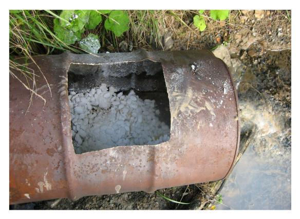
Figure 1: 55-gallon barrel with hole cut into it containing soda ash briquettes, with mine drainage flowing through each end of the barrel to allow dissolution of soda ash.
