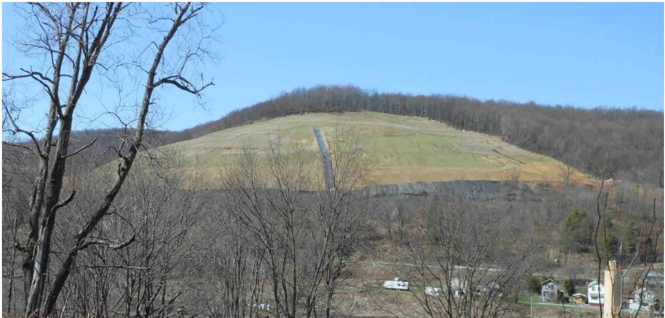
Ehrenfeld Coal Refuse Pile Reclamation Project Photo Credit: Pennsylvania Department of Environmental Protection
