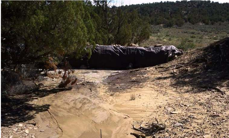
Figure 8. View downstream to the N7 temporary sediment dam after the first sediment event.
