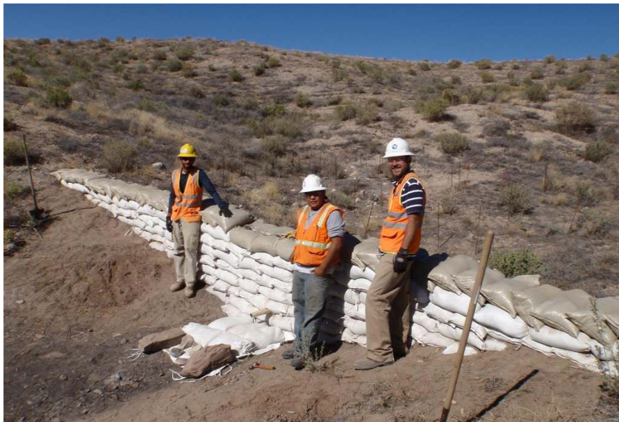
Figure 4. WV3 study site after construction of temporary sediment dam.
