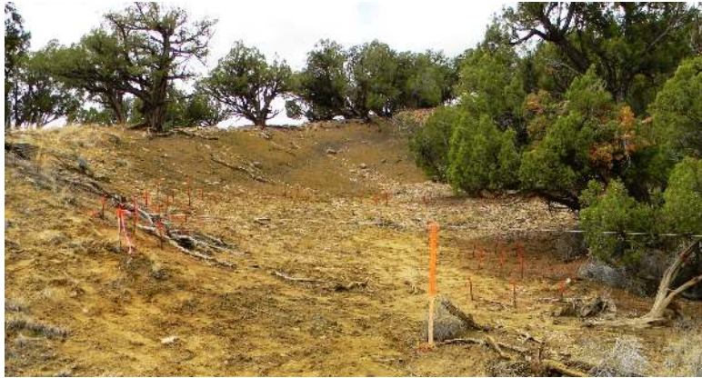
Figure 3. N7 sediment dam site with survey in progress and sediment pins installed.
