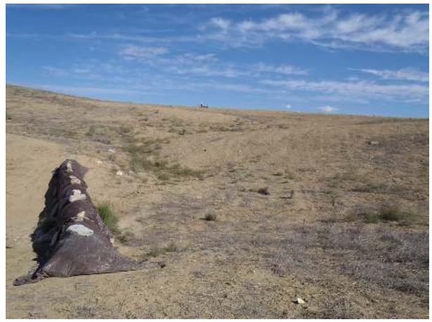
Figure 6. MV5 GeoFluv design with topdressing and poor to moderate vegetation establishment.
