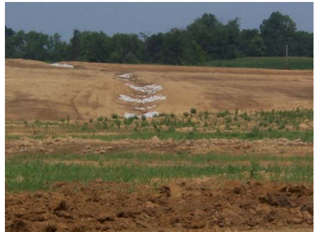
Water control structures on recently reclaimed land. These include grass waterways (top right), WASCOBs (lower left and right).
