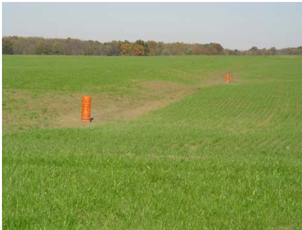
Water control structures on recently reclaimed land. These include grass waterways (top right), WASCOBs (lower left and right).
