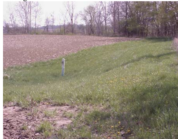
WASCOB embankment (right) and riser for drainage
