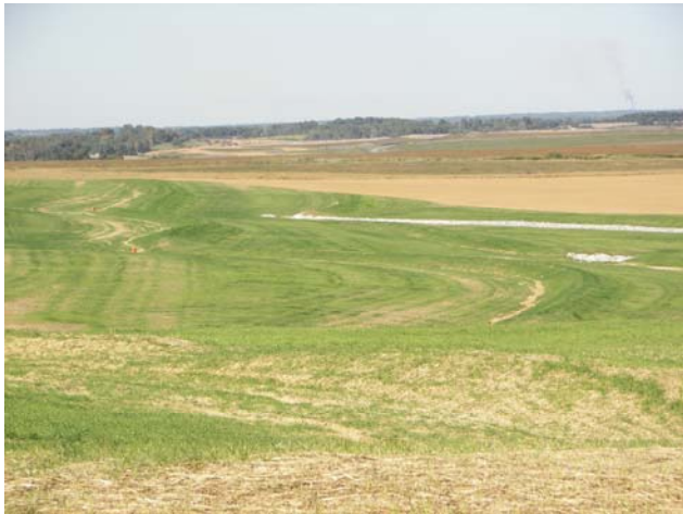
Contours used to control water on reclaimed land.
