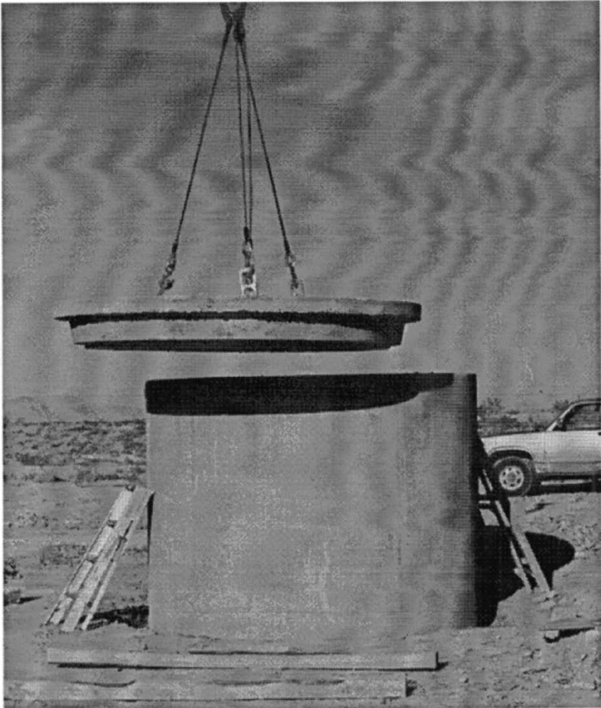
FIGURE 2. EXPENDABLE CONTAINMENT STRUCTURE
