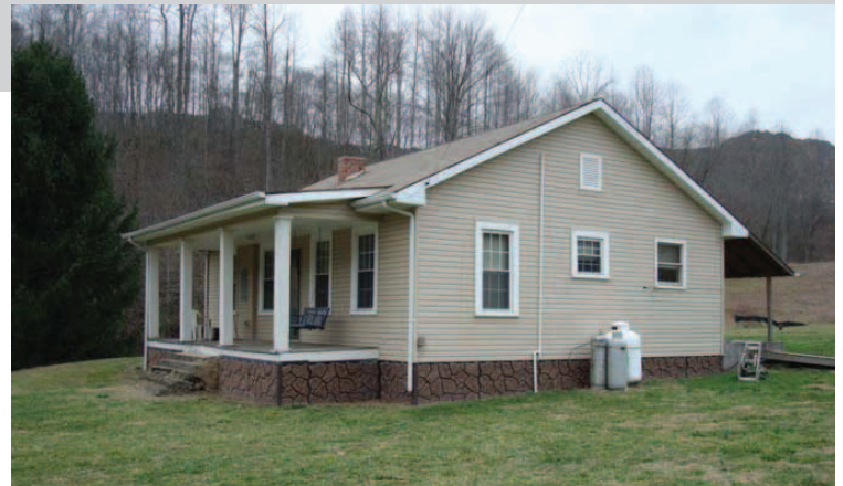
ABOVE PHOTO: Typical house in West Virginia near a surface coal mining operation. This particular house was instrumented for this project.
