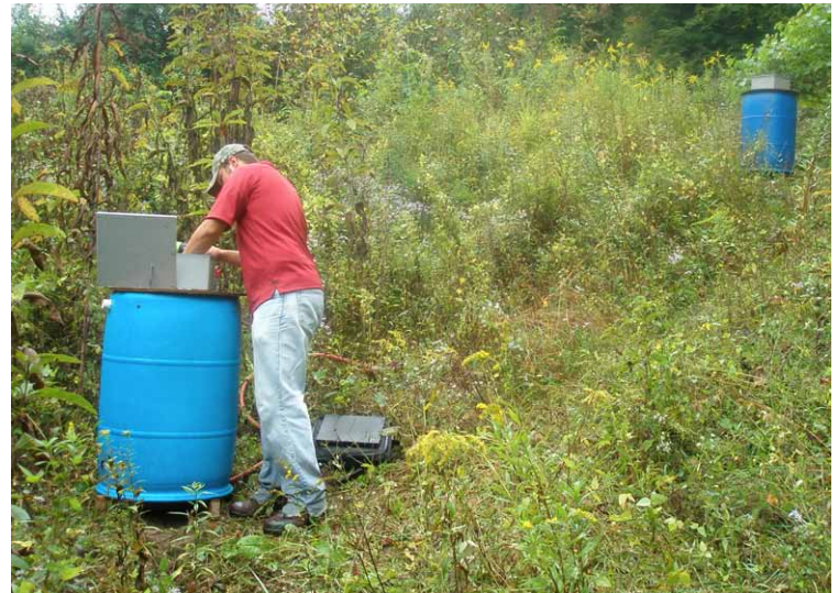
ABOVE PHOTO: Field installation of Apatite II treatment apparatus.
