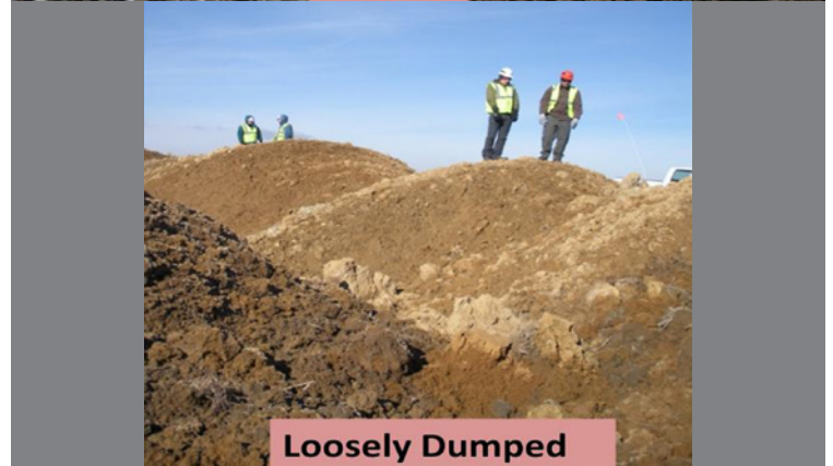
ABOVE PHOTOS: Conventional Graded Soil Replacement (Top). Loosely Dumped Soil Replacement (Bottom).
