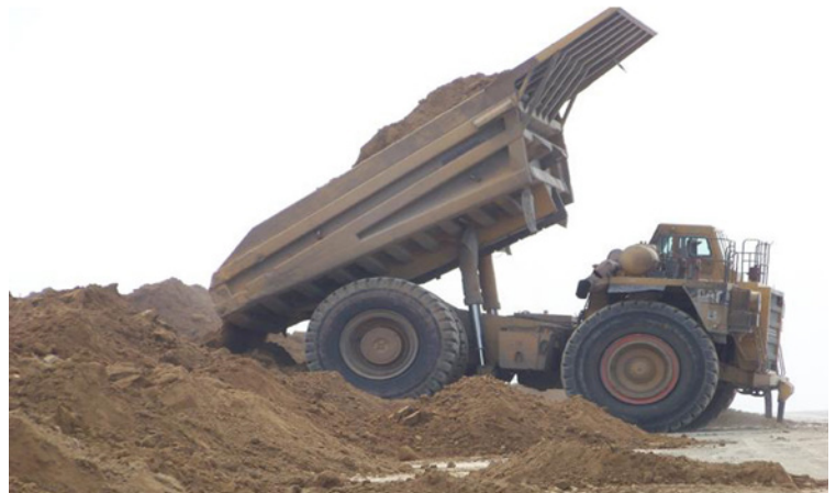
ABOVE PHOTOS: Ponding on Loosely Dumped Soil (Top). Placement of Loosely Dumped Soil (Bottom).
