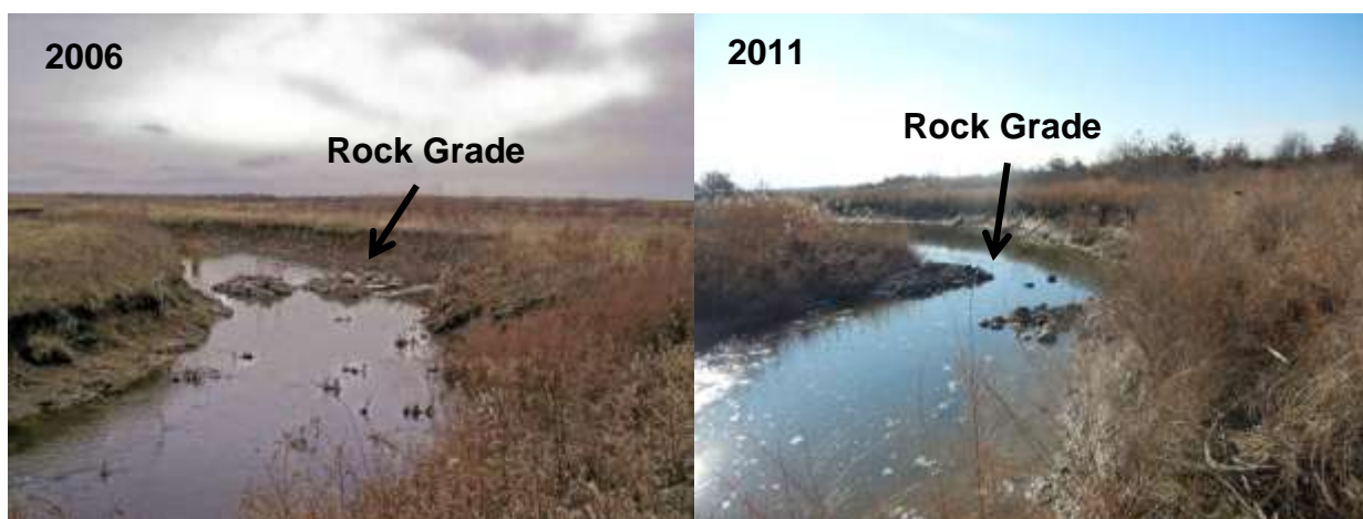
Figure 18. Bonnie Creek rock structures between cross sections 11662 and 12860 and location between cumulative channel length 2,500 and 2,900 m. Top photo is looking upstream at both structures (2005 flight), the middle photo is looking downstream at the structure at cross section 12860 (2005 flight), and the bottom photos are looking downstream at the structure at 12860 (2006 and 2011).
