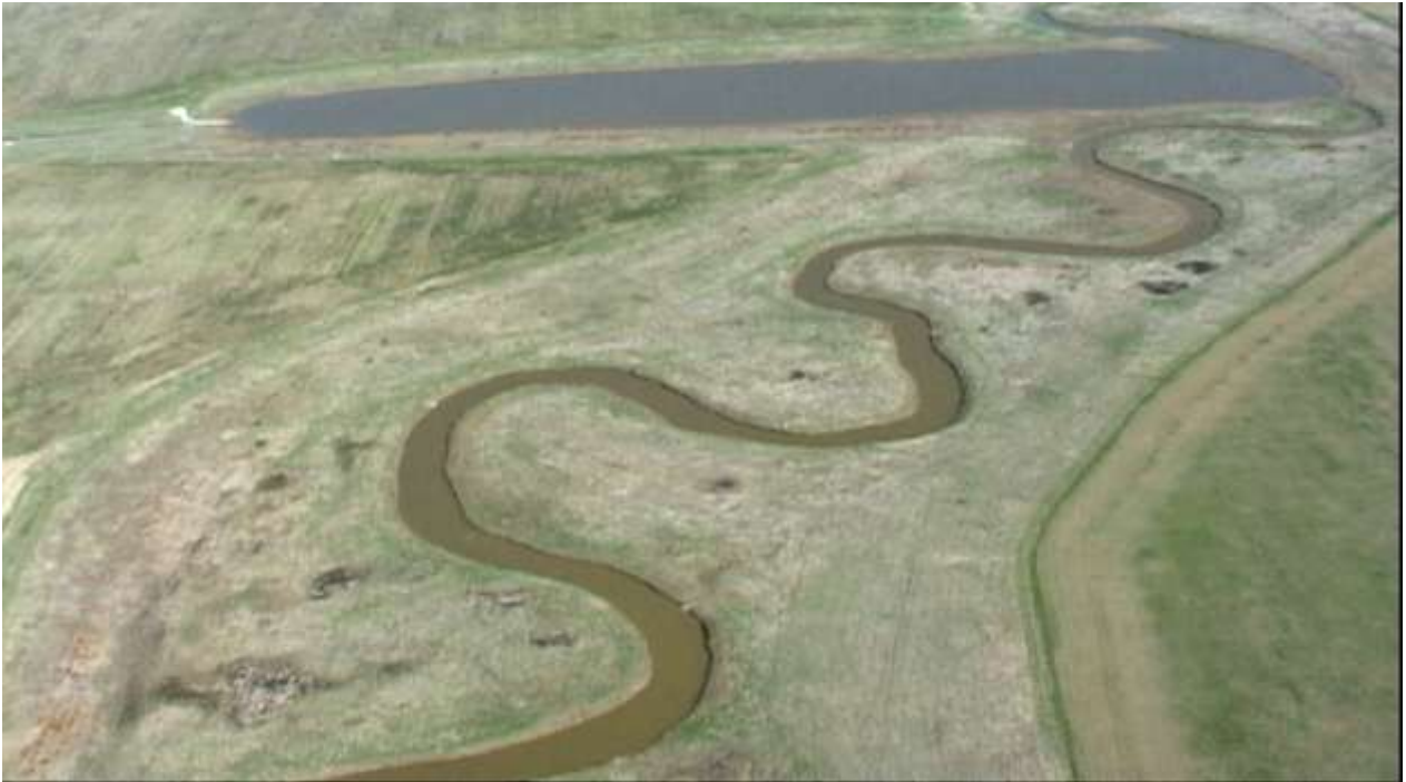
Restored reach downstream of incline pit
