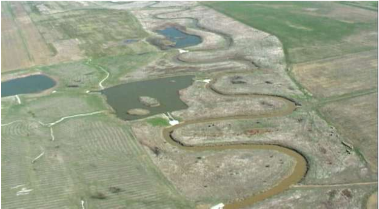
Restored reach downstream of incline pit
