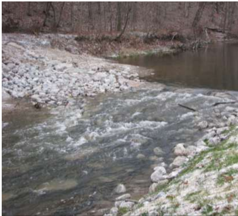
Figure 31. Example of a rock riffle that is keyed into the bank to help prevent the flow from flanking the structure. Top photo is looking across the channel and bottom photo is taken from the opposite bank looking upstream.
