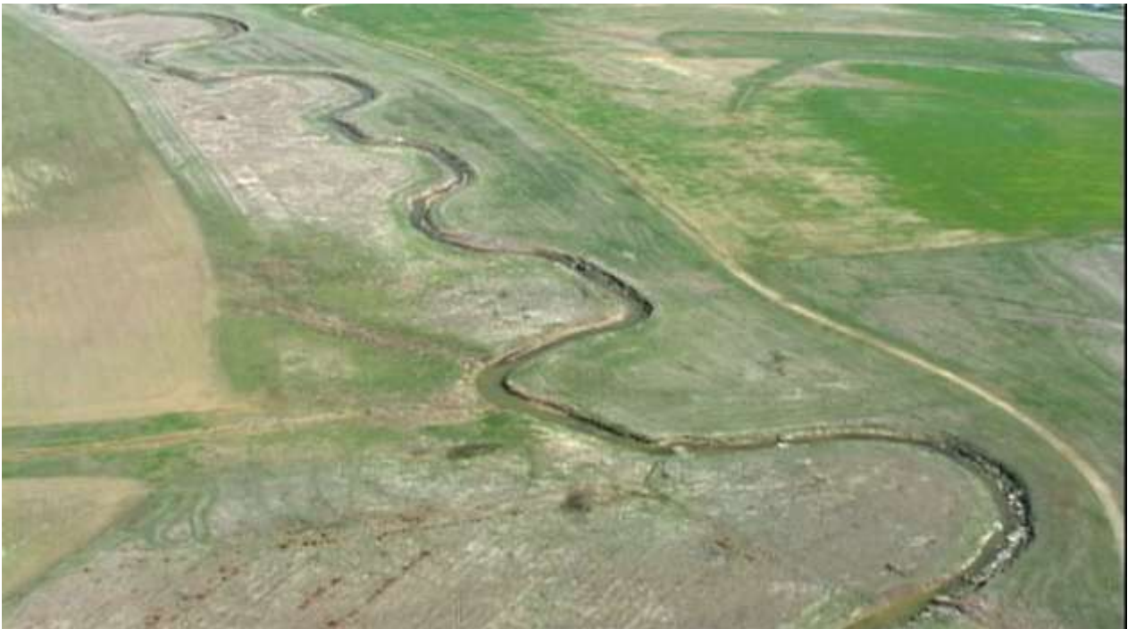
Restored reach downstream of Rte 154
