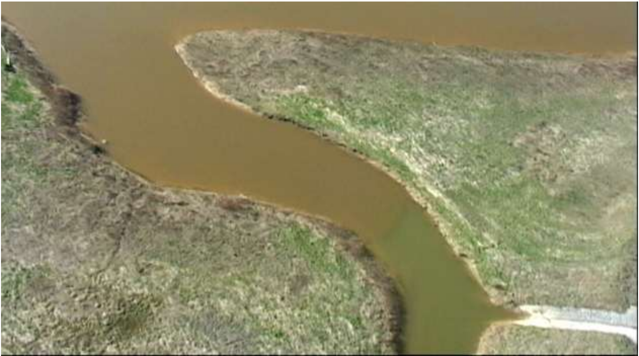
Twentieth bank below Rte 154 and directly upstream of the incline pit inlet
