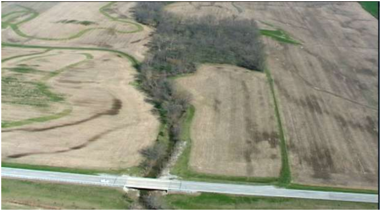
Agricultural ditch upstream of Rte 154
