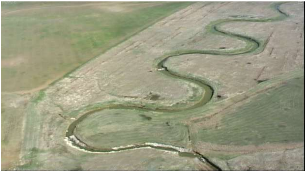
Restored reach downstream of Rte 154
