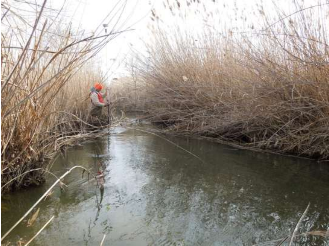
Figure 30. Pipestone Creek rock structure in 2011 (looking upstream) at cross section 793 and location cumulative channel length 241 m.
