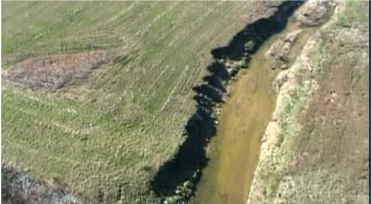
First bank downstream of Rte 154
