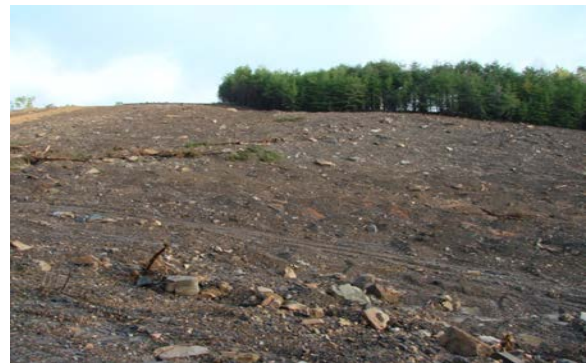
A photo taken the morning after 4.2 inches of rain from Hurricane Irma fell on the site with no observable erosion.
