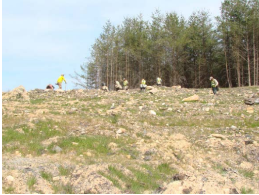
Williams Forestry planting the tree seedlings in the un-compacted backfill of Mine #43 with sparse vegetation to allow for tree growth.
