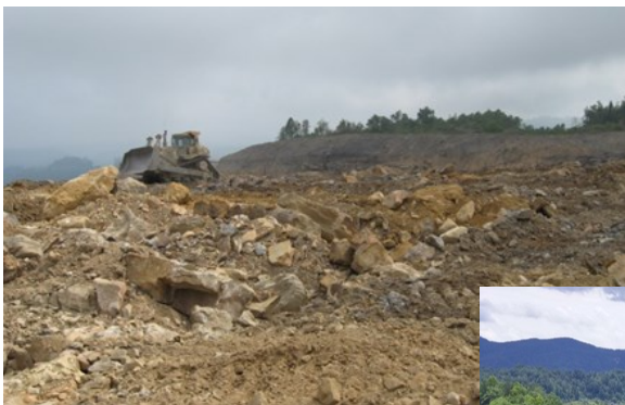
Above: A small reclamation dozer striking off the tops of end-dumps.
