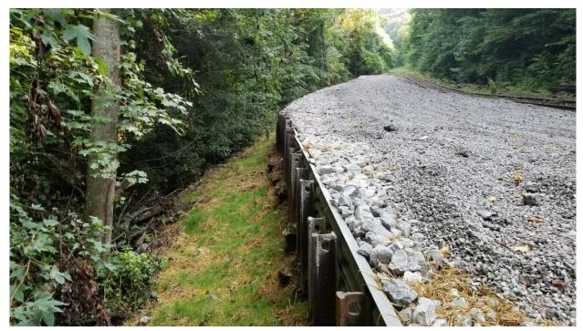
Rail Steel Installation as Part of the Big South Fork Scenic Railway Slide Repair
