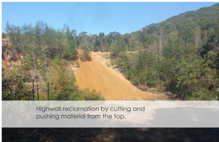
Highwall reclamation by cutting and pushing material from the top.
