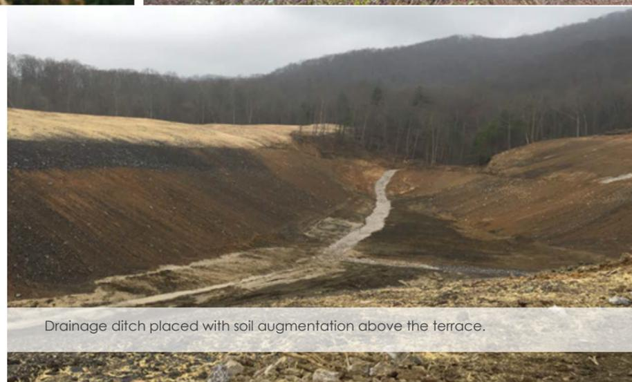
Drainage ditch placed with soil augmentation above the terrace.
