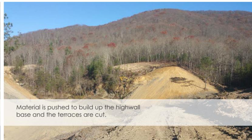
Material is pushed to build up the highwall base and the terraces are cut.
