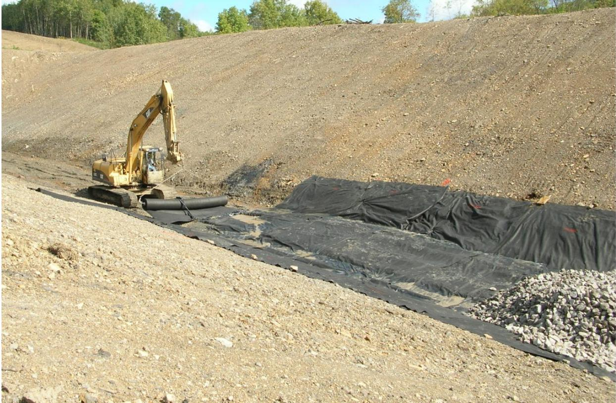
Figure 4: Excavator unrolling Non-woven Geotextile to act as a protective barrier between soil and synthetic liner as part of constructing an ALD.
