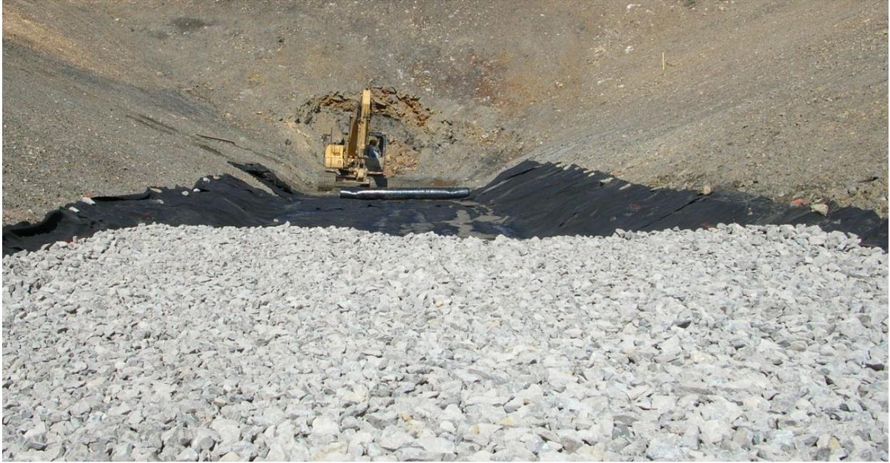
Figure 5: Excavator unrolling synthetic liner ovetop of a layer of non-woven Geotextile.
