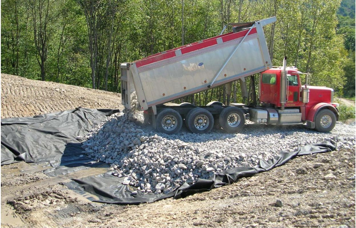
Figure 6: Triaxle truck dumping limestone on top of synthetic liner during ALD construction.
