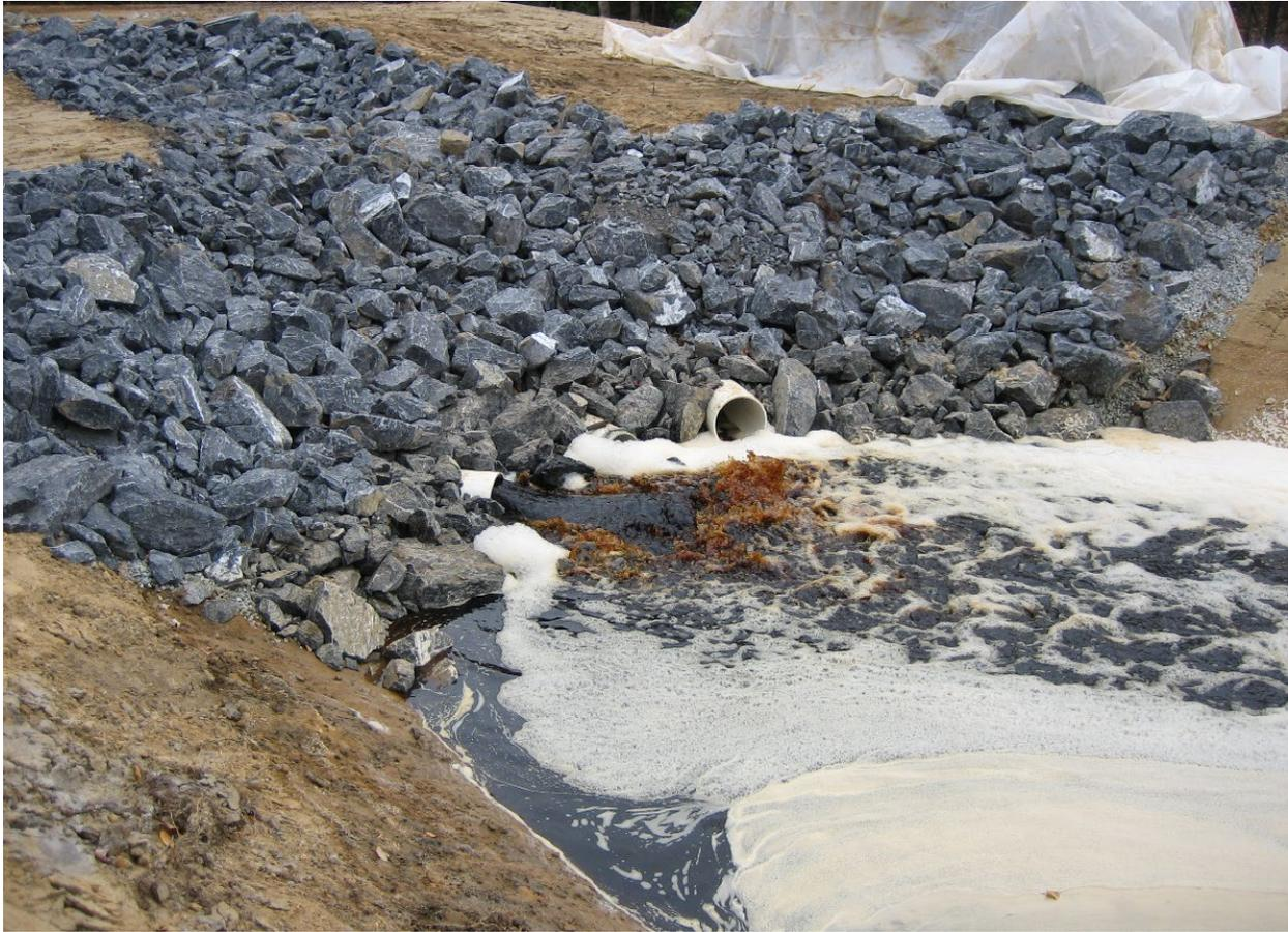
Figure 19: First discharge of a newly constructed Bioreactor after the incubation period. The organic-rich water with elevated BOD & COD is an environmental concern if not appropriately treated in the subsequent ponds.
