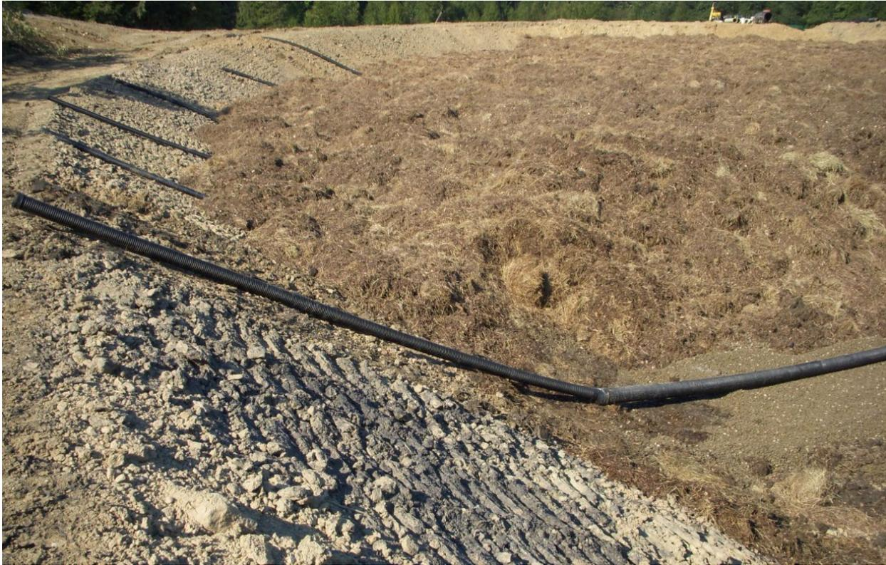
Figure 9: Bioreactor under construction showing effluent collection pipe embedded in rock (bottom right) to be covered by Bio Mix layer. Pipe cleanouts were installed along the side slopes to remove debris if collection piping becomes clogged. Once a common practice, cleanout pipes are now sparingly used because of short circuiting issues experienced by flow along the sides of the clean out pipes.
