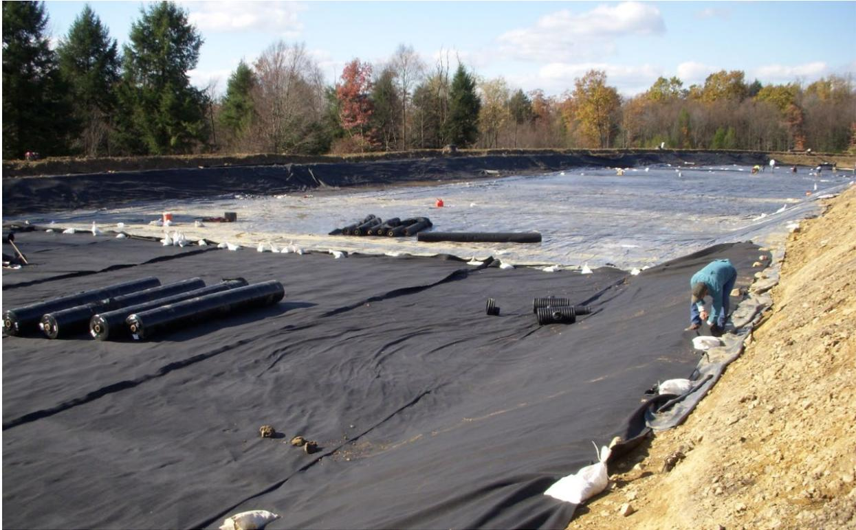
Figure 26: Non-woven geotextile being placed on top of a synthetic liner during the construction of a Bioreactor.
