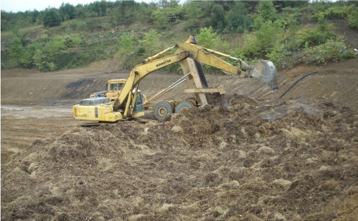
Figure 12: Truck end-dumping the Bio Mix material and excavator trying to carefully smooth out the surface to obtain a uniform thickness to promote a uniform flow pattern. Extreme caution must be used to prevent compaction of the Bio Mix material, which is irreversible.
