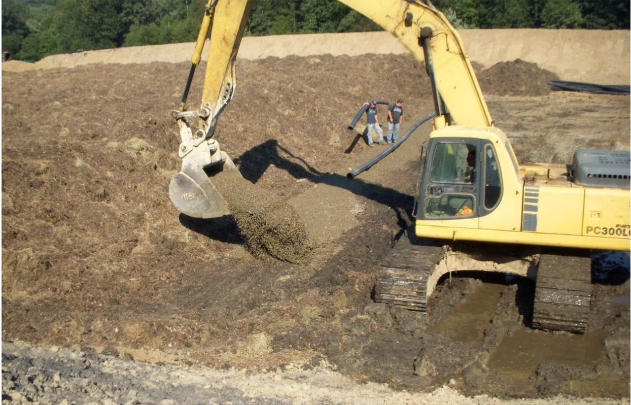
Figure 8. Excavator installing rock bedding for piping network.
