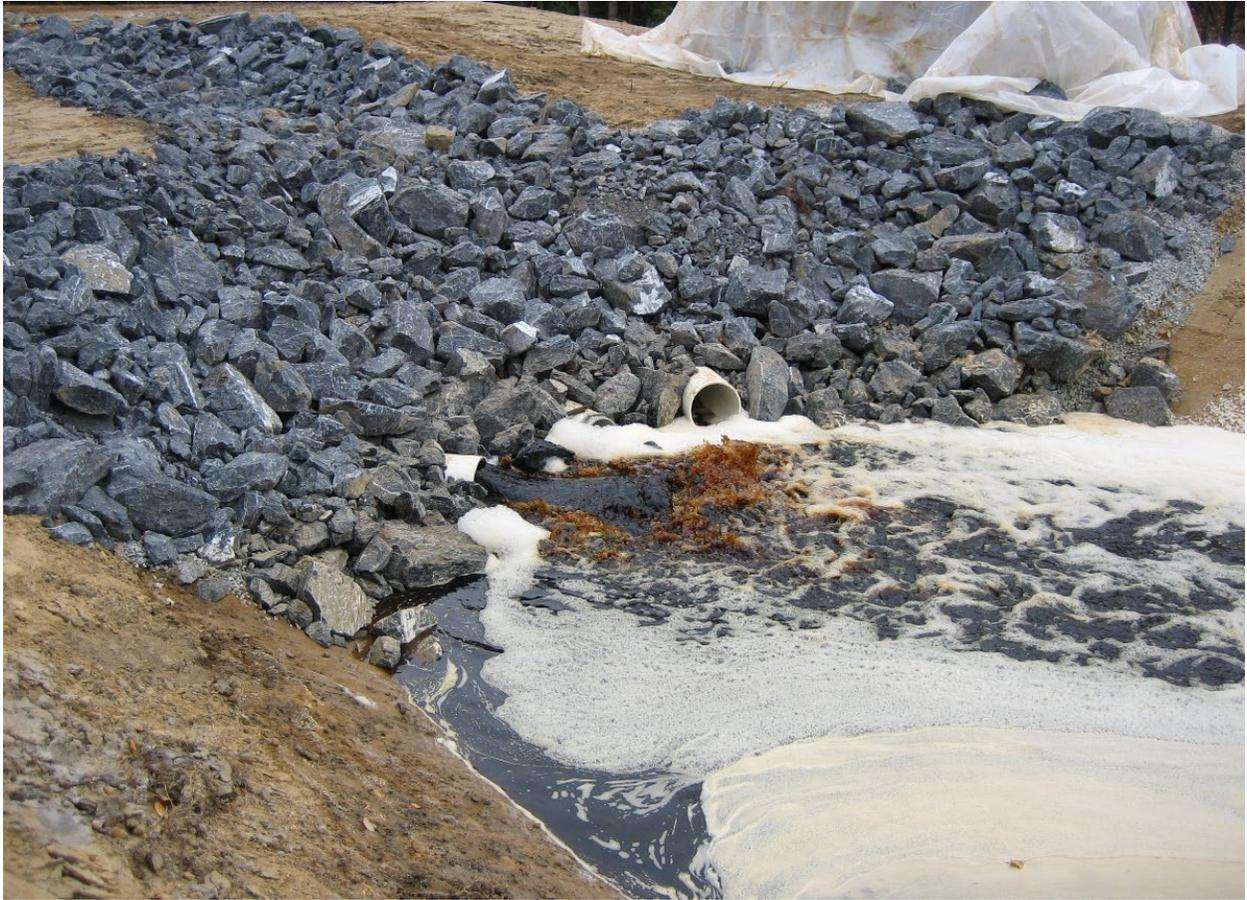
Figure 19: First discharge of a newly constructed Bioreactor after the incubation period. The organic-rich water with elevated BOD & COD is an environmental concern if not appropriately treated in the subsequent ponds.
