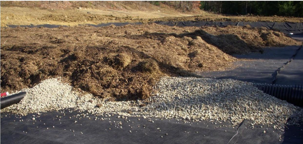
Figure 7: Close up image of effluent collection pipe embedded in rock shown in Figure 5. Image shows spur pipes (bottom left) connecting into the trunk (header) pipe (bottom right).
