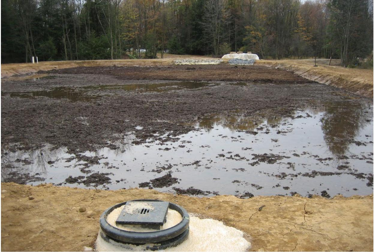
Figure 18: Newly constructed Bioreactor being filled with mine drainage in preparation for a two-week incubation period.
