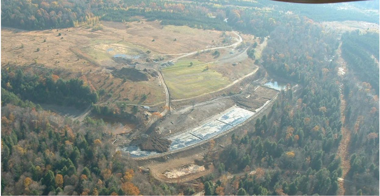
Figure 13: Bio Mix being spread over top of a non-woven geotextile and synthetic liner system during the construction of a 2.0 acre Bioreactor.
