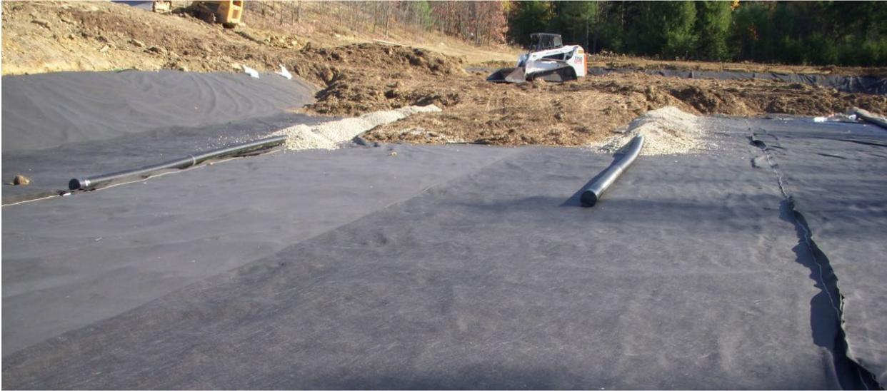
Figure 6: Lateral piping network placed overtop of non-woven geotextile and synthetic liner. Note the pipes placed in rock bedding to protect perforated openings.
