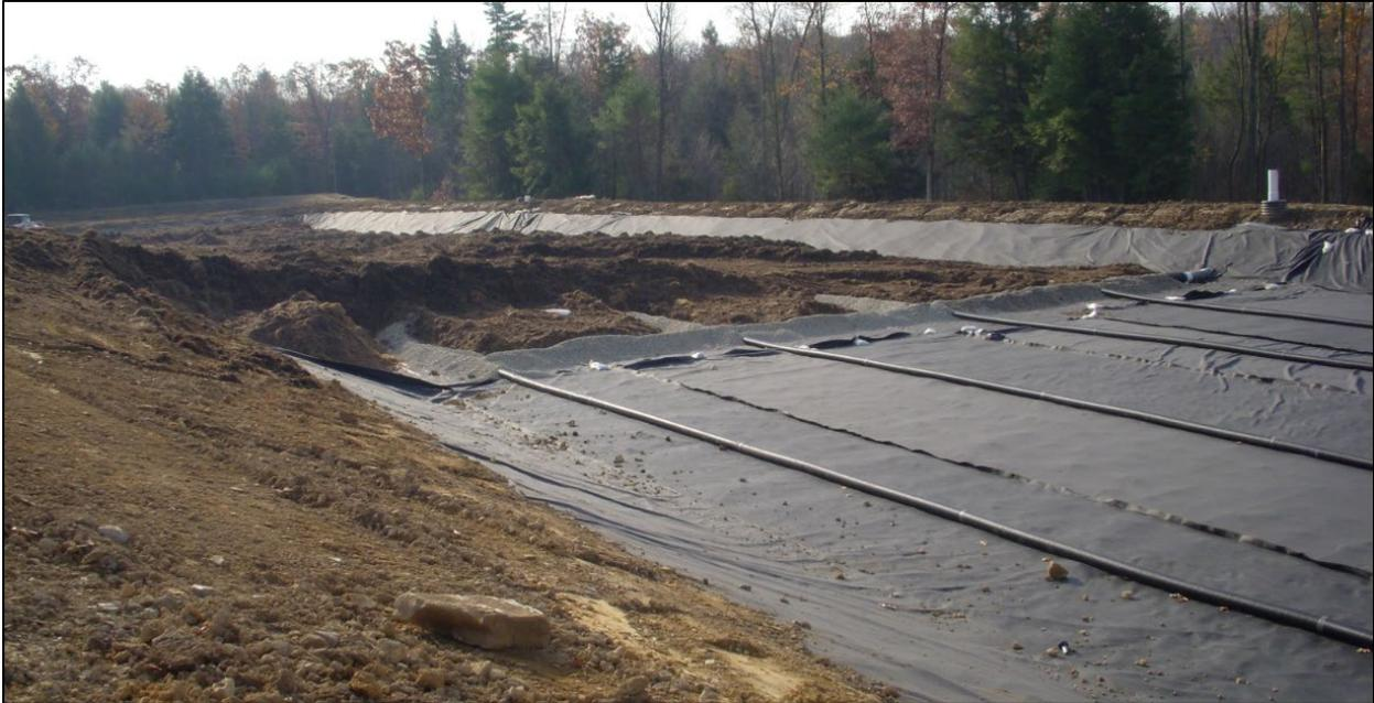
Figure 10: Alternative piping network design. Spur pipes are aligned parallel to the longest dimension of the Bioreactor and the trunk (header) pipe is positioned across the width of the bioreactor. The piping network is embedded in stone to protect the perforations from the overlain Bio Mix layer.
