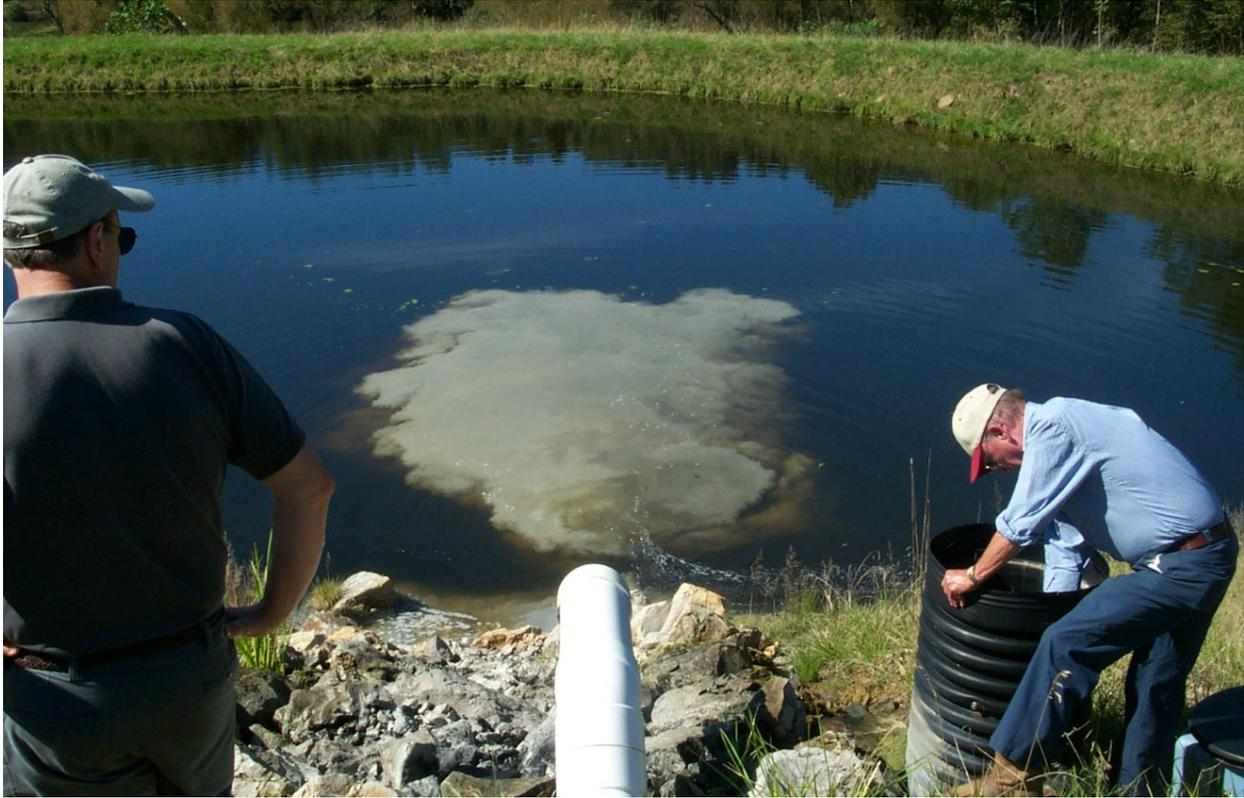
Figure 11: Short term flush of a Bioreactor effluent pipe to prevent build up of precipitates. Whitish elemental sulfur flushed into a subsequent pond filled with ferrous monosulfide. FeS particulates constantly discharge from this bioreactor to the settling pond due to an insufficiently sized Bio Mix layer.
