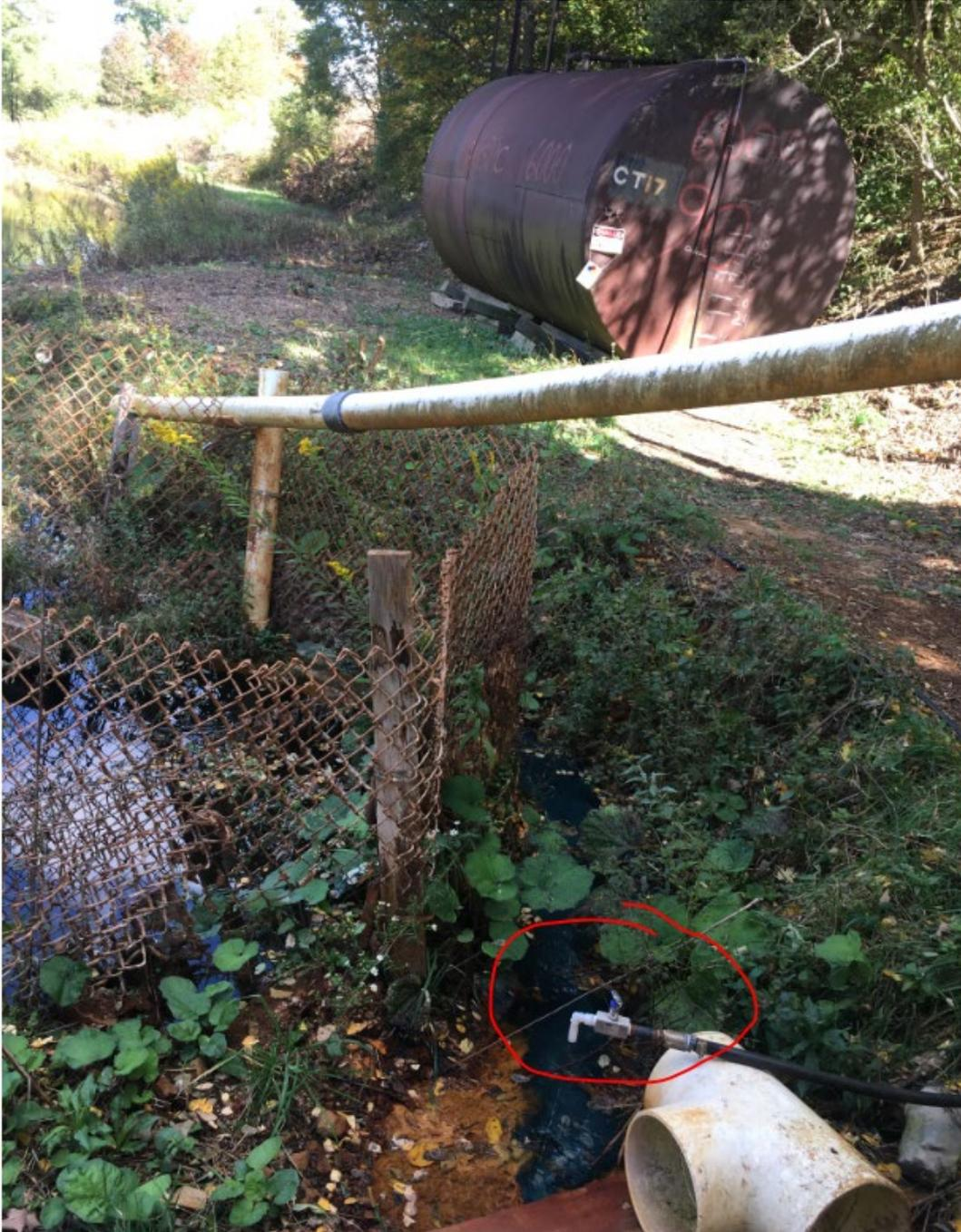
Figure 8: Photo of a “typical” manually operated steel tank Caustic Soda treatment system. A 6,000-gallon steel tank is set on wooden cribbing to prevent contact between ground moisture and the tank. A red circle highlights the poly feeder line and manually adjusted valve that doses the mine drainage below.
