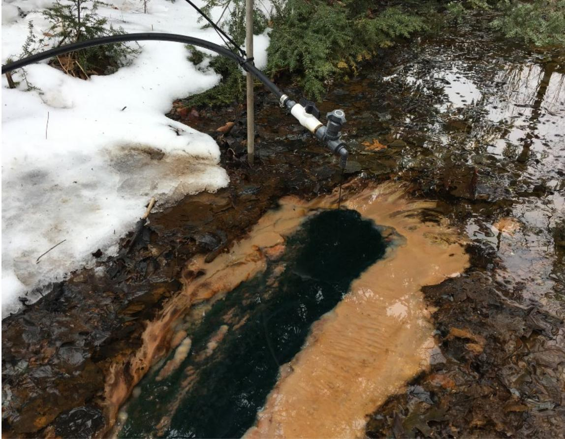
Figure 12: Grey needle valve used to control Caustic Soda dose into mine drainage. Notice a ball valve is located before the needle valve to prevent pressured flow to the needle valve to provide better control when a low dose is required.
