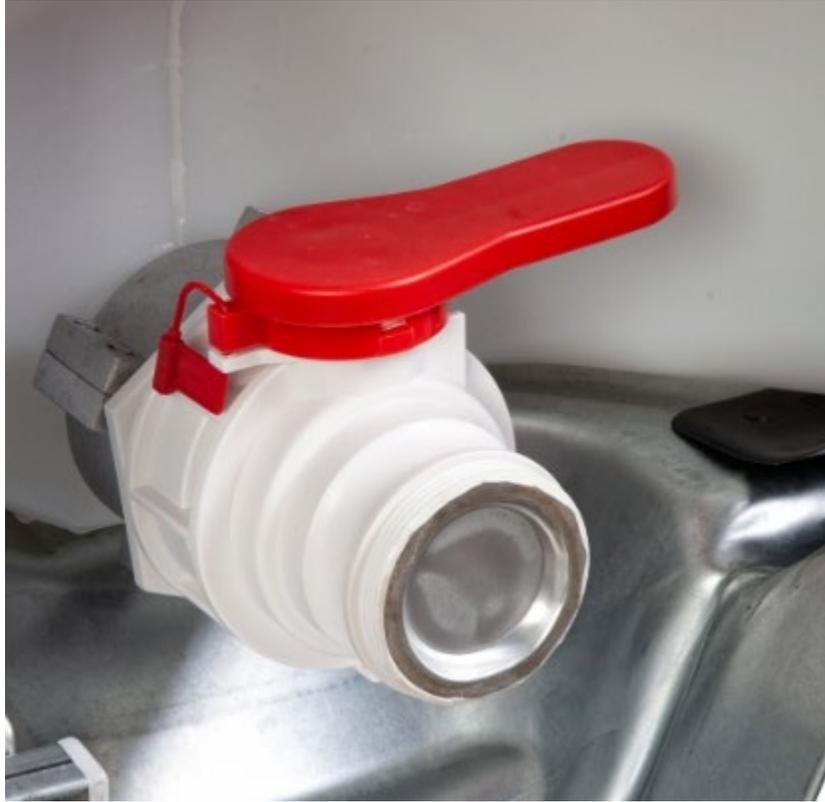
Figure 4: Picture of the 2-inch camlock valve assembly for connecting hoses and lines to Caustic Soda totes. The camlock is used for quick connects to hoses while the NPT threaded connection is used for connecting to poly feeder line.
