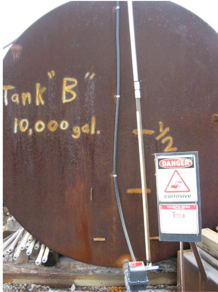
Figure 11: Photo of a 10,000-gallon steel Caustic Soda storage tank with caustic level sight tubing
