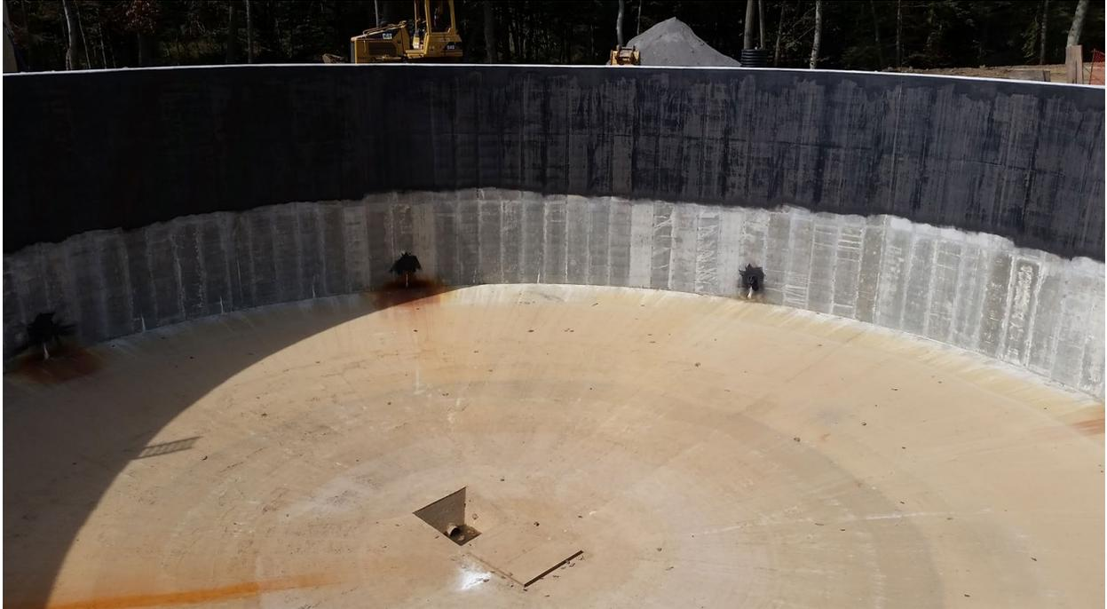
Figure 11: A newly constructed concrete clarifier showing the sloped floor and the sludge sump and sludge pump line extending under the floor.
