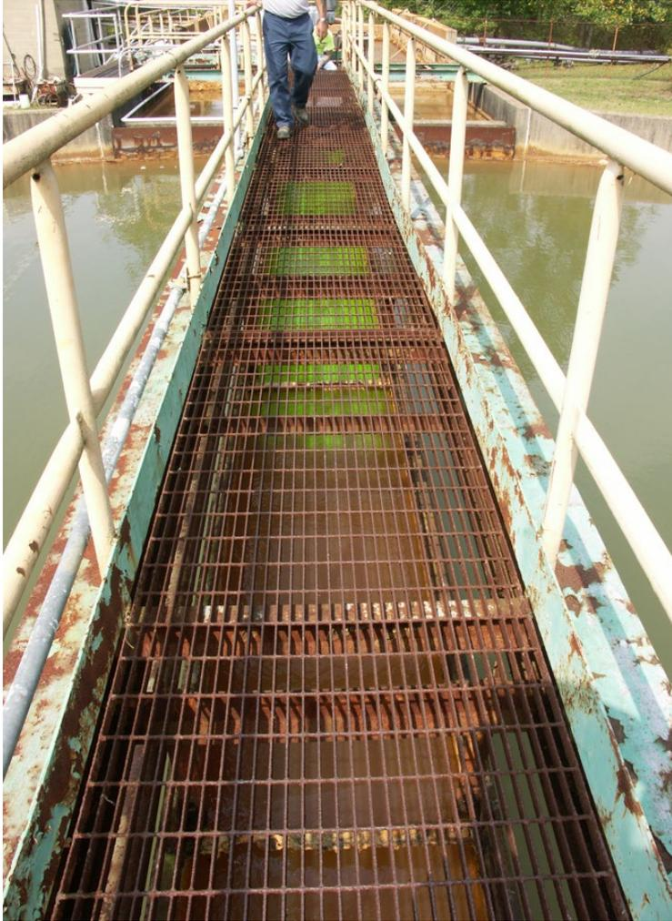
Figure 14: Bright green dye introduced into conveyance trough that connects the reaction tank to the center well of the clarifier. The open conveyance trough is located under the catwalk to the center well. Also, note the corrosion of the steel catwalk and handrailing extending to the center well.
