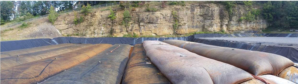
Figure 47: Additional photo of geotubes show in in Figure 46. The geotubes will be buried in place as part of a reclamation plan to reclaim the highwall in shown in the photo. Soil will be placed over the final elevation of the geotubes and vegetated as part of the plan.
