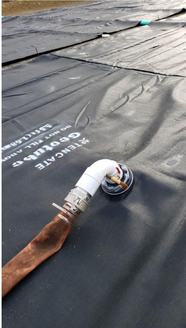
Figure 49: Sludge is pumped through the red hose and into the geotube where the polymer flocculated particles are larger than pores in the geotube, which causes the solids to be retained in the bag while the water seeps through the fabric, dewatering the solids.
