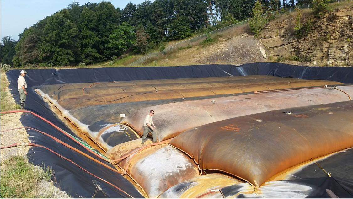
Figure 46: Large geotubes receiving sludge pumped from a clarifier. Eventually, the geotubes will be buried in place for final disposal.
