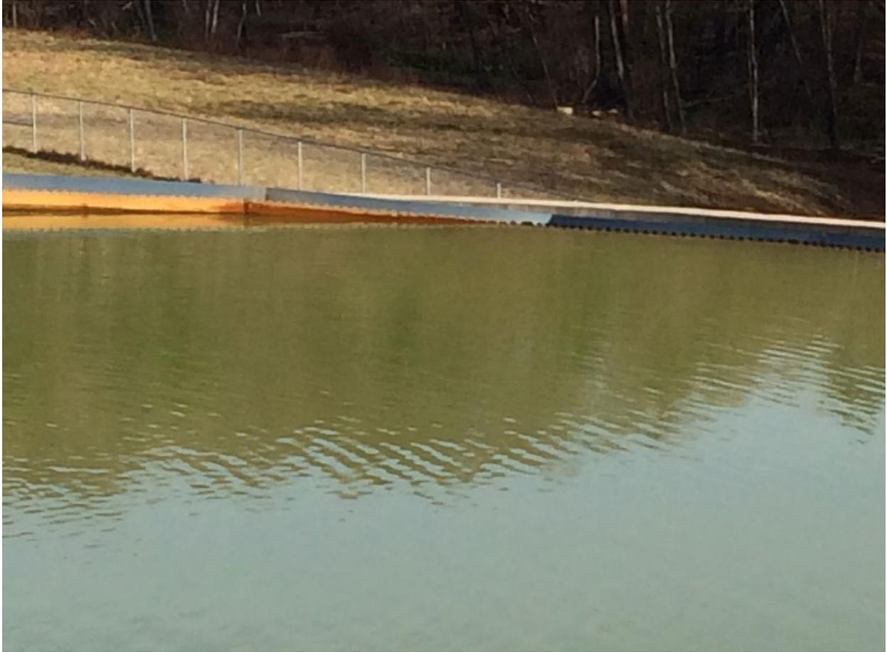
Figure 39: Photo showing a portion of the yellow saw-toothed weir fell into the clarifier because corrosion from the mine drainage caused the fasteners to fail.
