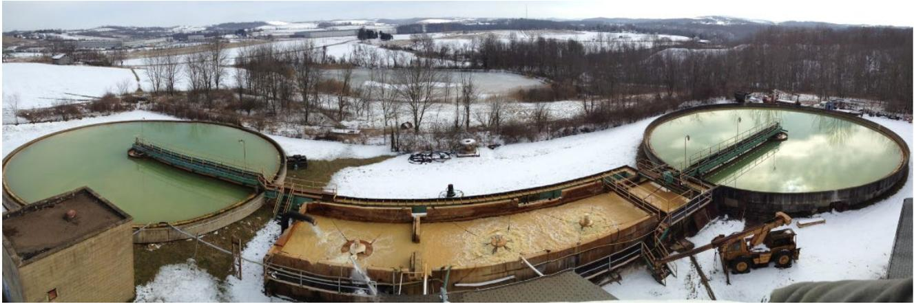
Figure 5: Hydrated Lime mine drainage treatment plant using two conventional clarifiers operating in parallel.
