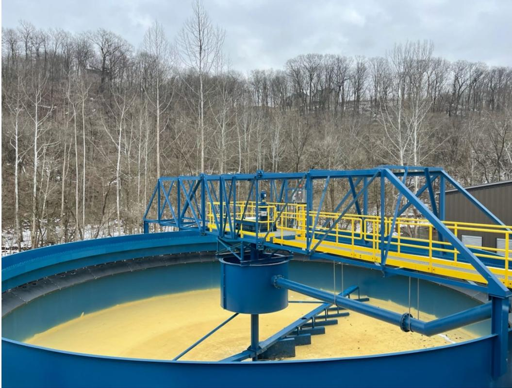
Figure 31: A newly constructed welded steel conventional clarifier with a concrete floor. Note the greyish density curtain baffle extending the perimeter of the inside wall under the laundering weir.
