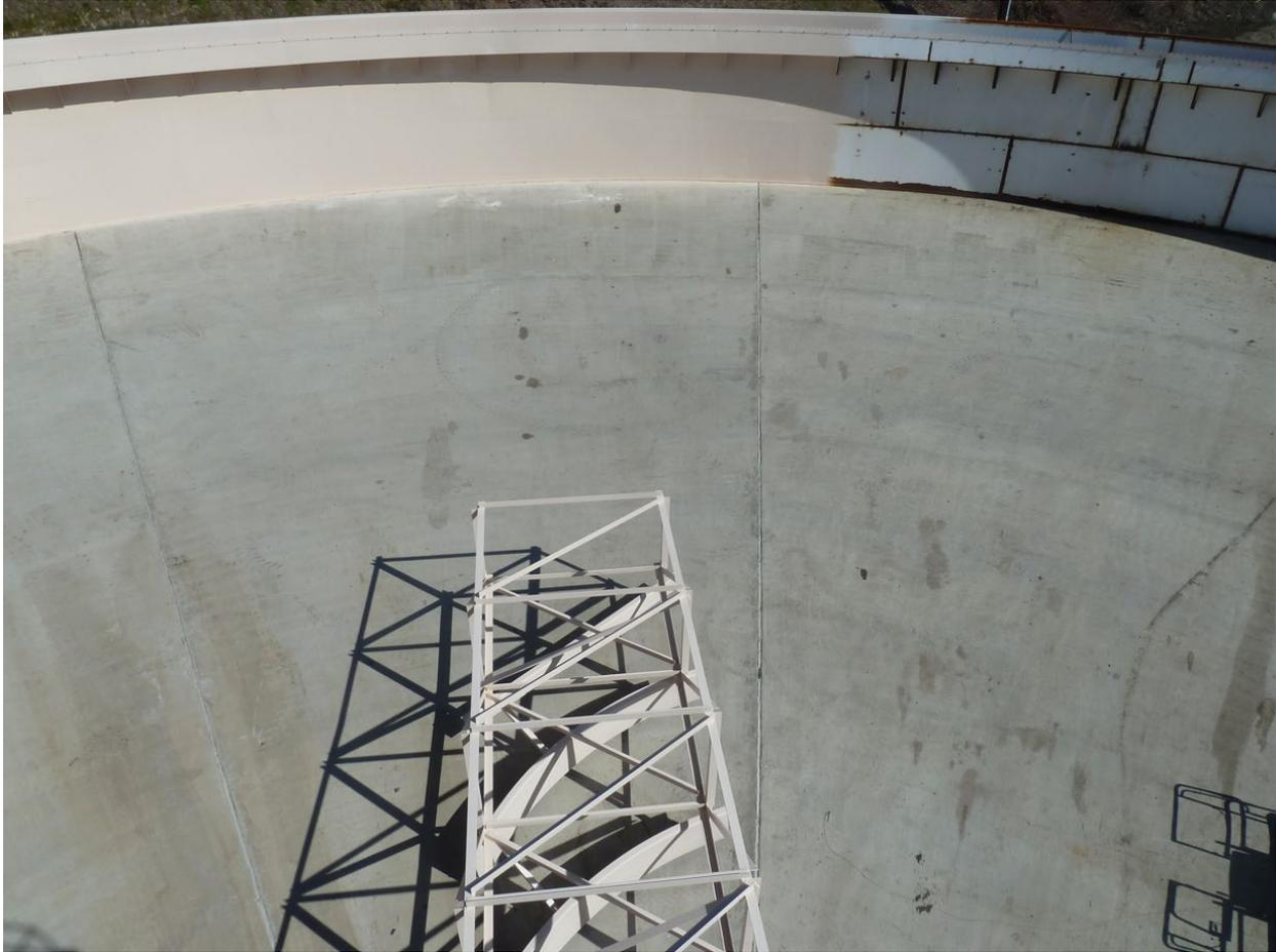
Figure 34: A viewpoint of the inside of the welded steel clarifier shown in Figures 31 & 32. Note the inside wall is in the process of being painted beige. A protective coating was also applied to the steel to retard corrosion. The steel panel weld marks are clearly visible on the unpainted section.
