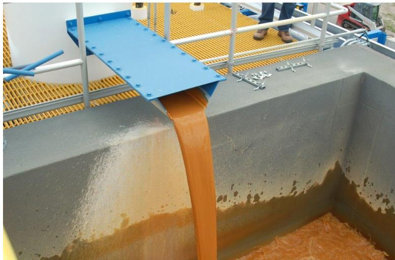
Figure 26: Outfall of sludge conditioning tank showing the sludge/lime slurry mixture being discharged into the reaction tank to react with the untreated influent.
