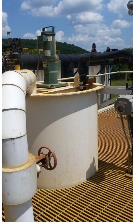
Figure 25: A steel mix tank to condition the recycled sludge with hydrated lime. The white pipe is the sludge recycle line and the smaller diameter black pipe entering the top right of the tank is the lime slurry line. A mechanical mixer is used to flash mix the sludge and lime slurry. The lime/sludge mixture is then discharged to the reaction tank where it reacts with the untreated influent water.
