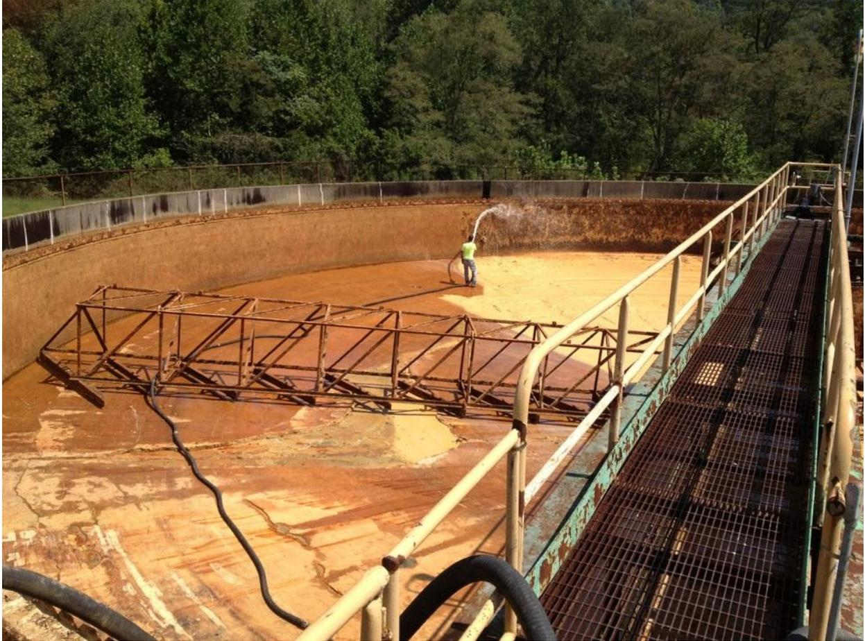
Figure 12: Photo of an operator using a pressurized hose to clean iron hydroxide scale from the walls, floor, and rakes of the clarifier. Notice the lack of scale to the left of the operator compared to the right. Figure 9 shows the empty clarifier after it was cleaned.
