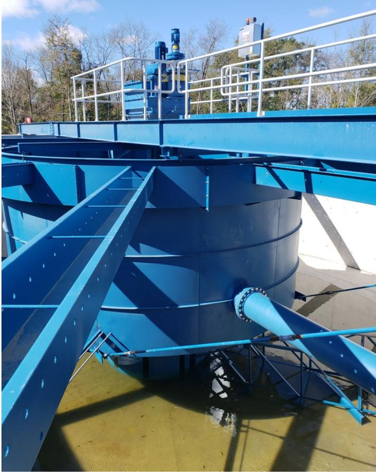
Figure 24: A picture showing the reaction well of a newly constructed solids contact clarifier. The twelve-inch inlet pipe transports the raw mine drainage into the draft tube where it is reacted with hydrated lime and recycled sludge.
