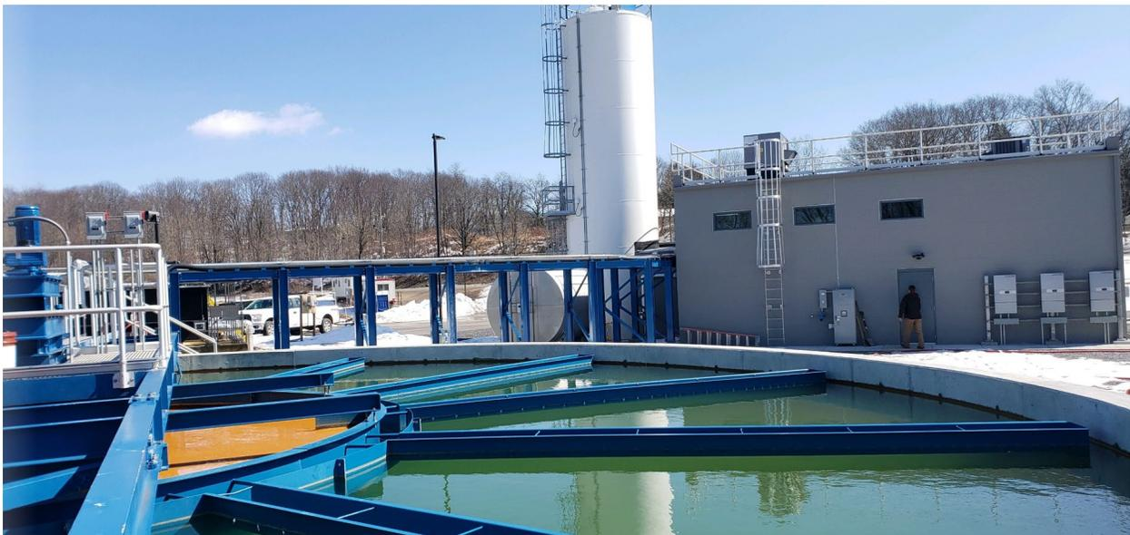
Figure 21: Concrete walled solids contact clarifier. Draft tube and reaction skirt/well are underwater and not visible.
