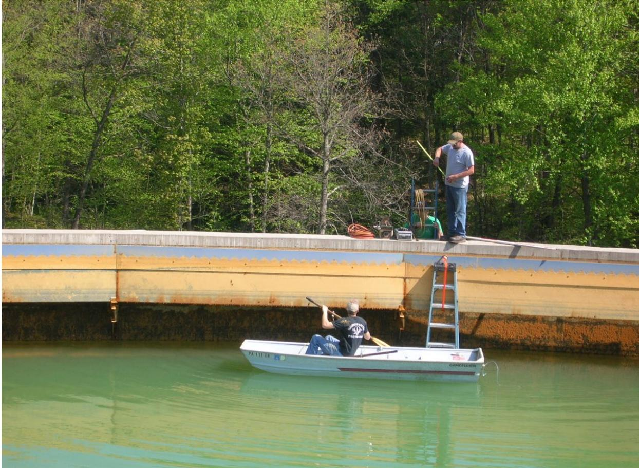
Figure 37: Works replacing the steel bolts that attach the overflow weir to the concrete wall with stainless steel bolts. The corrosion caused some of the bolts to fail causing the weir to fall into the clarifier (Figures 38 and 39). Stainless steel fasteners must be used when treating mine drainage. Note the top of the ladder is resting against the saw-toothed overflow weir and the weir is resting on support beams that secure the weir to the concrete wall.
