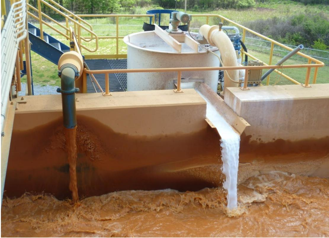
Figure 27: The HDS conditioning tank was retrofitted to separate the lime slurry and sludge due to constant scaling and maintenance issues with the tank. The recirculated sludge is shown discharging from the blue pipe at the left of the photograph and the lime slurry is discharging from the conditioning tank.
