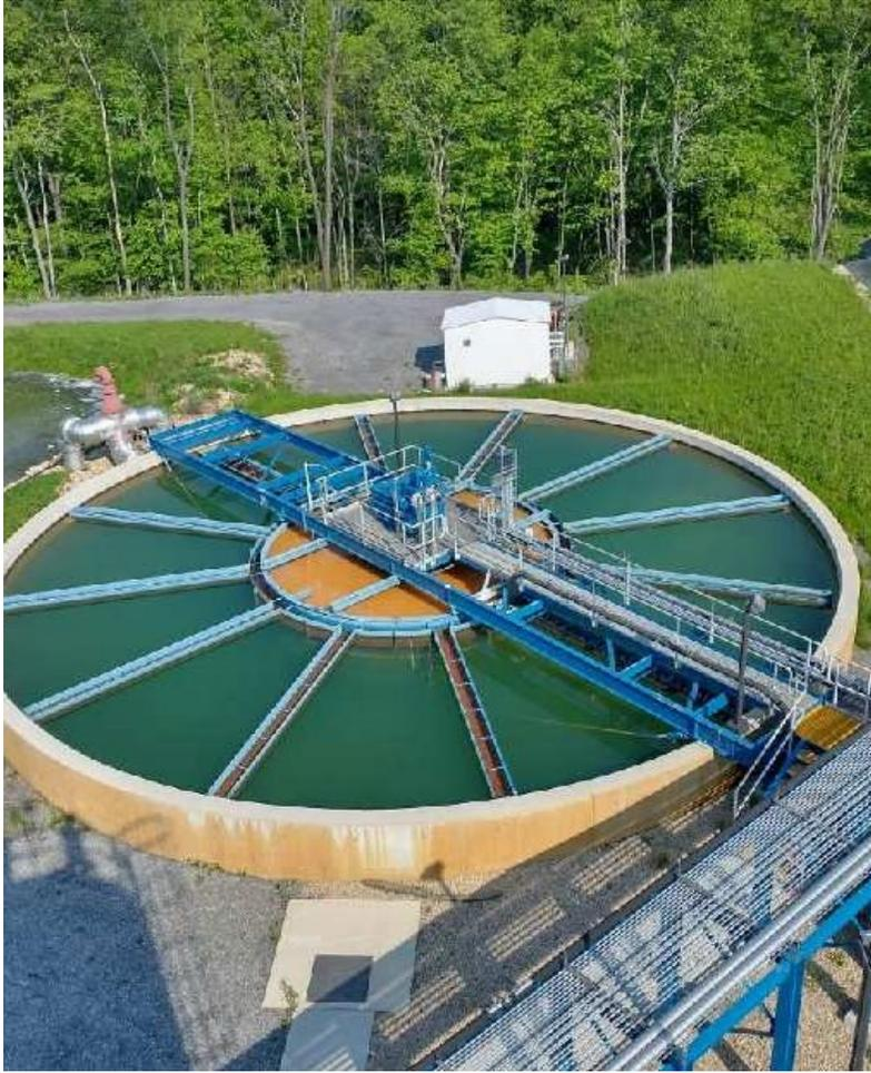
Figure 22: Aerial view of newly constructed concrete-walled Solids Contact Clarifier treating ferruginous mine drainage. Sludge pumps are housed in the white building and the effluent is discharged from silver piping into a wetland where total Fe is reduced from 0.5 to 0.03 mg/L.
