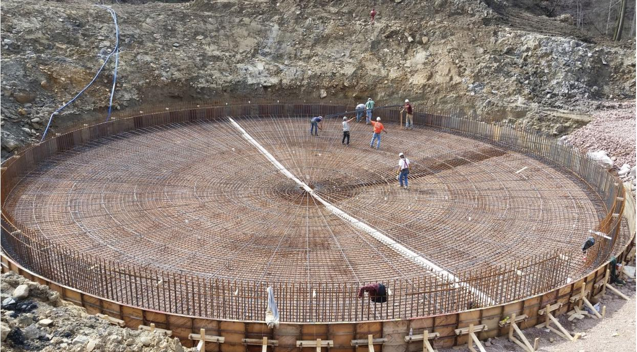
Figure 30: Workers constructing a rebar form to pour a sloped concrete floor of a clarifier. The vertical form is to pour the concrete side walls.
