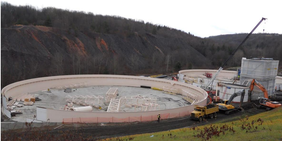
Figure 32: The construction of a 220 ft diameter welded steel clarifier with a concrete floor. Note the missing steel panels that allow for equipment access into the clarifier during construction.
