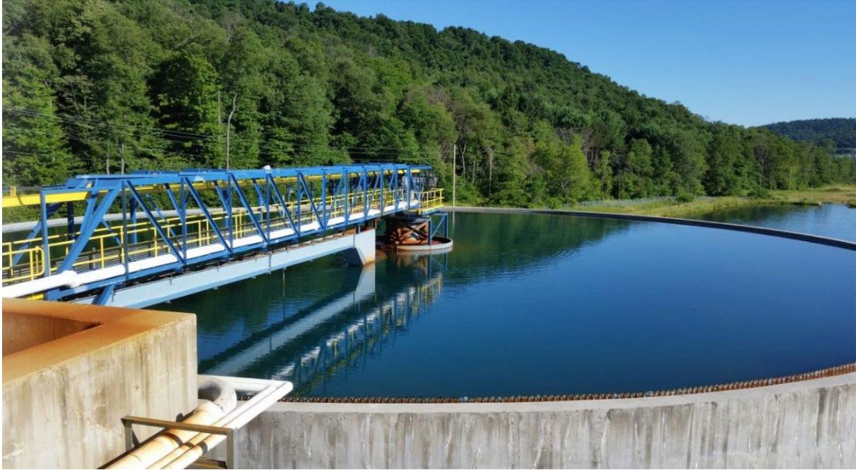
Figure 4: Typical concrete conventional clarifier used to in mine drainage treatment in the eastern U.S.
