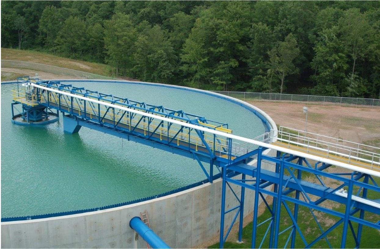
Figure 6: Concrete-walled conventional clarifier. Note the open trough located under the walkway (catwalk) to the center well. Diluted polymer flocculant is added at hydraulic jump in the trough where the water falls by six inches to provide the mixing necessary to disperse the diluted polymer throughout the waste stream. Particle-to-particle interactions occur within the center well to promote agglomeration of particles.
