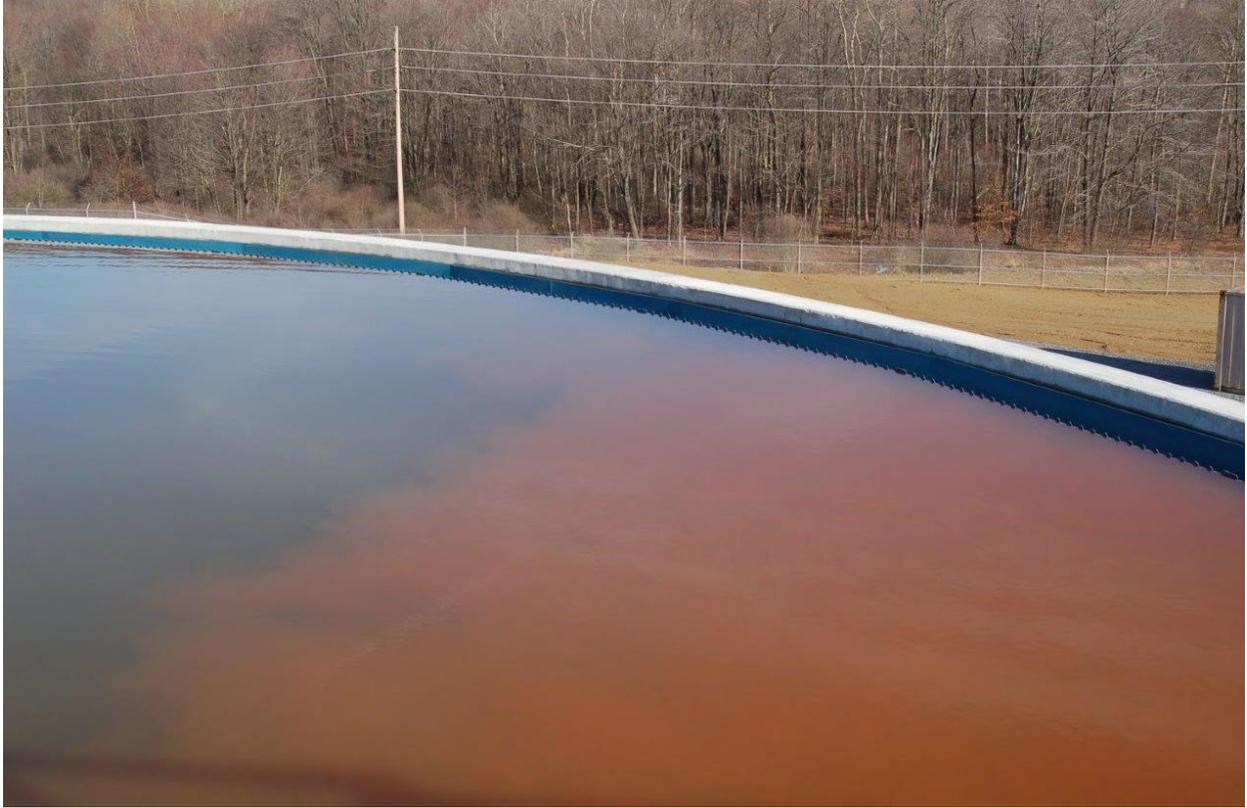
Figure 19: Cloud of suspended iron hydroxide that followed the rake rotation after conversion from hydrated lime to hydrogen peroxide.
