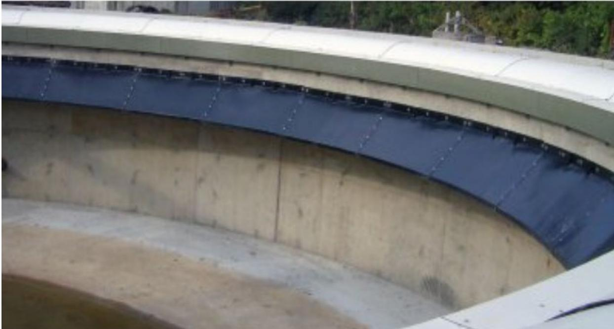
Figure 40: The blue fiberglass Density Current Baffle extends (courtesy of NEFCO) extends along the periphery of the outer wall just below the overflow weir.
