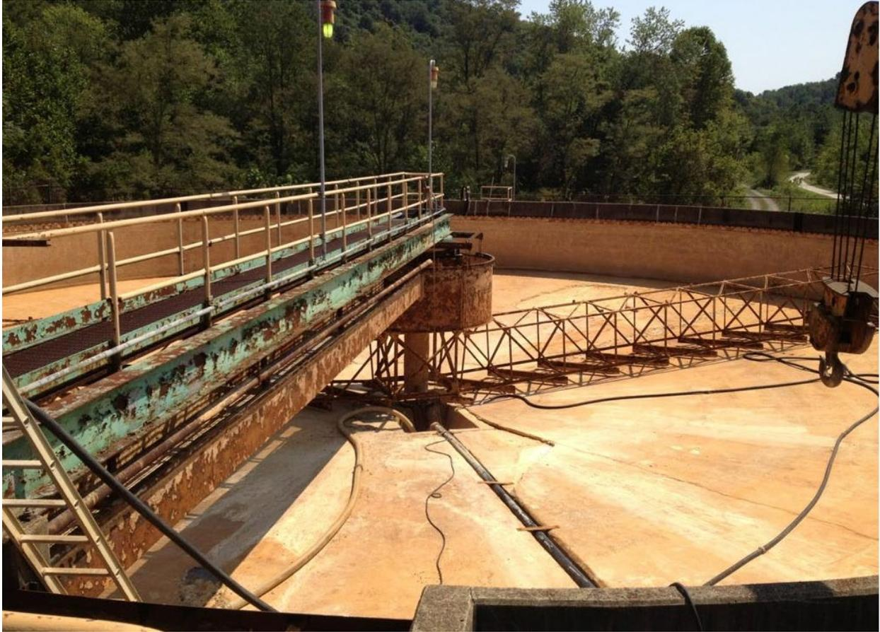
Figure 10: A different angle of the same clarifier shown in Figure 5. Note the rectangular sludge sump located in the bottom center of the clarifier along with the steel sludge line embedded into the concrete floor of the clarifier. A sludge pump housed in the operations building pumps sludge from the sludge sump through the sludge line to an injection borehole that terminates in an underground mine. Also note the corrosion on the steel catwalk and handrailing extending to the center well.
