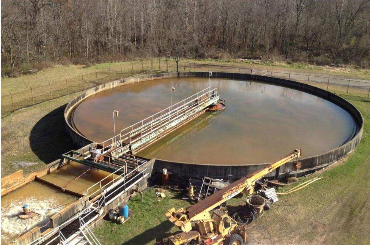
Figure 8: Photo of a 110 ft diameter conventional clarifier. Note red-colored sludge blanket is within five feet of the surface indicating the need to pump sludge. Reducing the volume of the sludge bed allows the sludge blanket to reposition lower in the clarifier.
