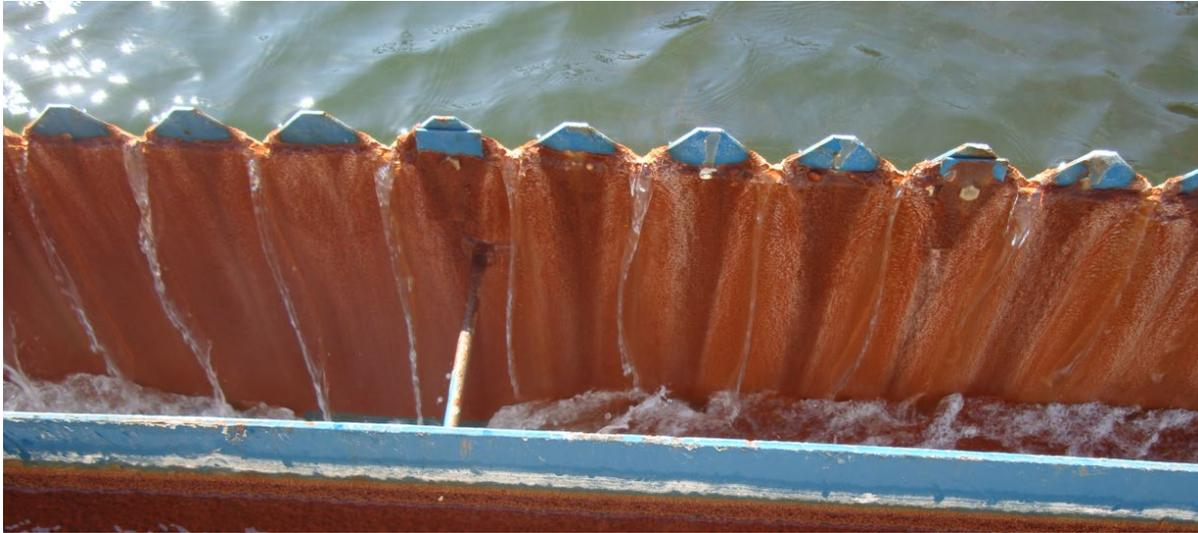
Figure 35: Photo showing a buildup of iron in the valleys of the sawtooth overflow weir.
