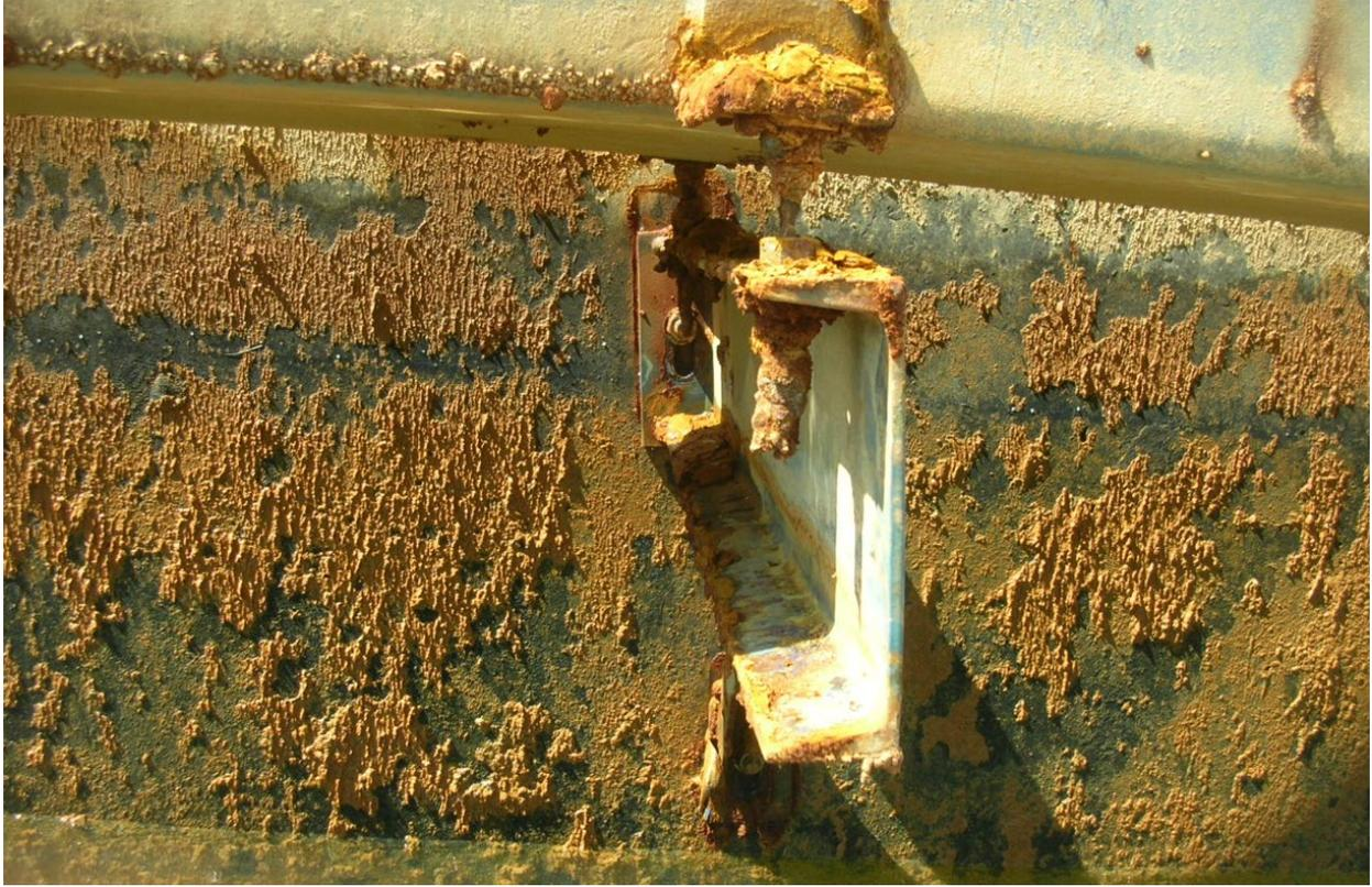
Figure 38. Photo showing the corrosion of the fasteners that connect weir (top of photo) to the steel support beam and that connect the beam to the concrete wall. The steel fasteners were replaced with stainless steel.
