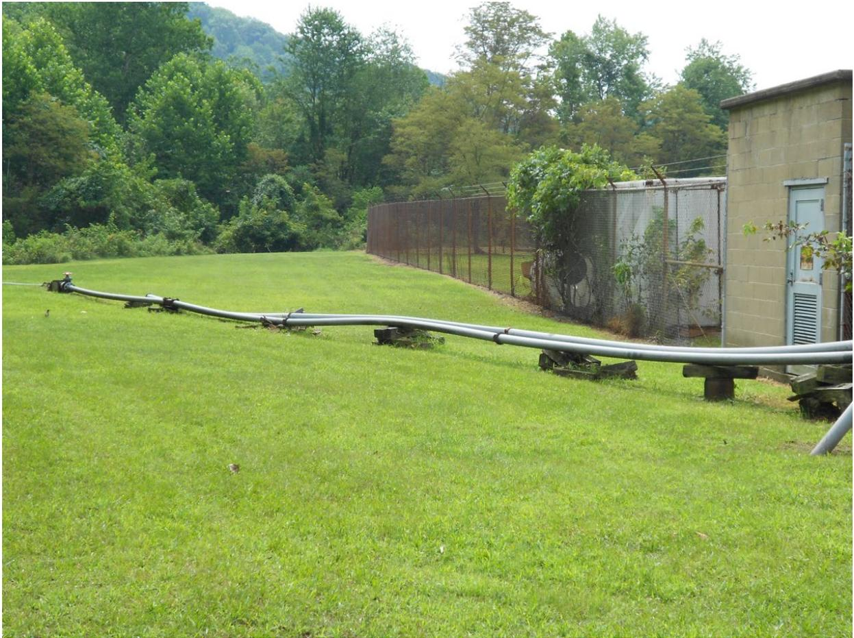
Figure 43: Overland sludge pipeline to injection borehole. Most sludge lines are buried but this one is supported by wooden cribbing.
