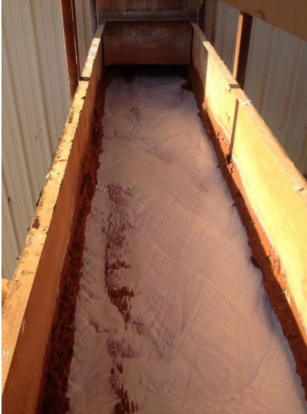
Figure 28: HDS trough system developed by Bethlehem Steel. Lime slurry is dosed into the trough directly inside the building. The sludge/lime slurry mixture travels 30 feet before being discharged into the reaction tank to mix with the untreated influent water. The conditioned sludge in this photo has a higher percentage of lime since the photo was taken during a sludge pumping event. When sludge is pumped from the clarifier to an injection well, the amount of sludge recirculated decreases.
