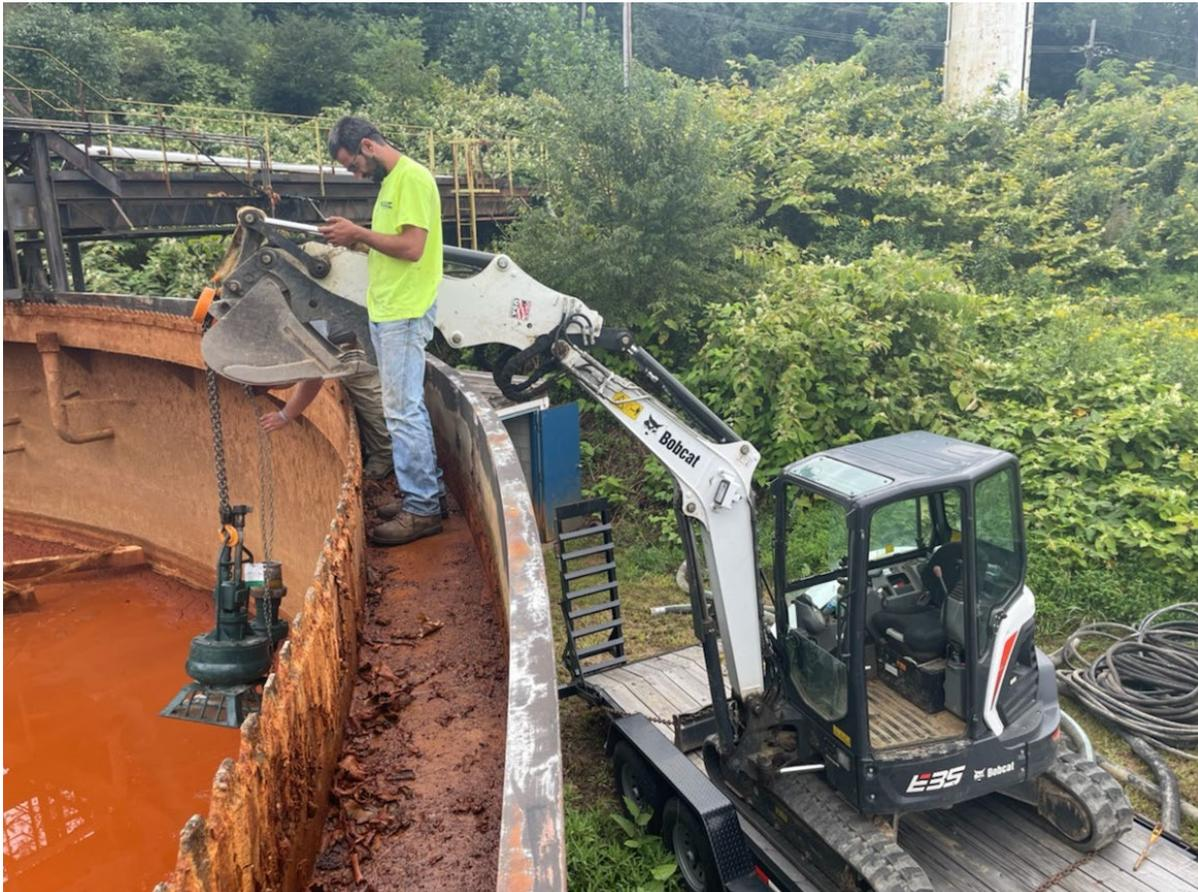
Figure 36: Worker lowering pump to clean inside of clarifier. In addition, the iron-coated overflow weir and transport trough (working standing in trough) will be cleaned to restore an even distributed flow across the weir.
