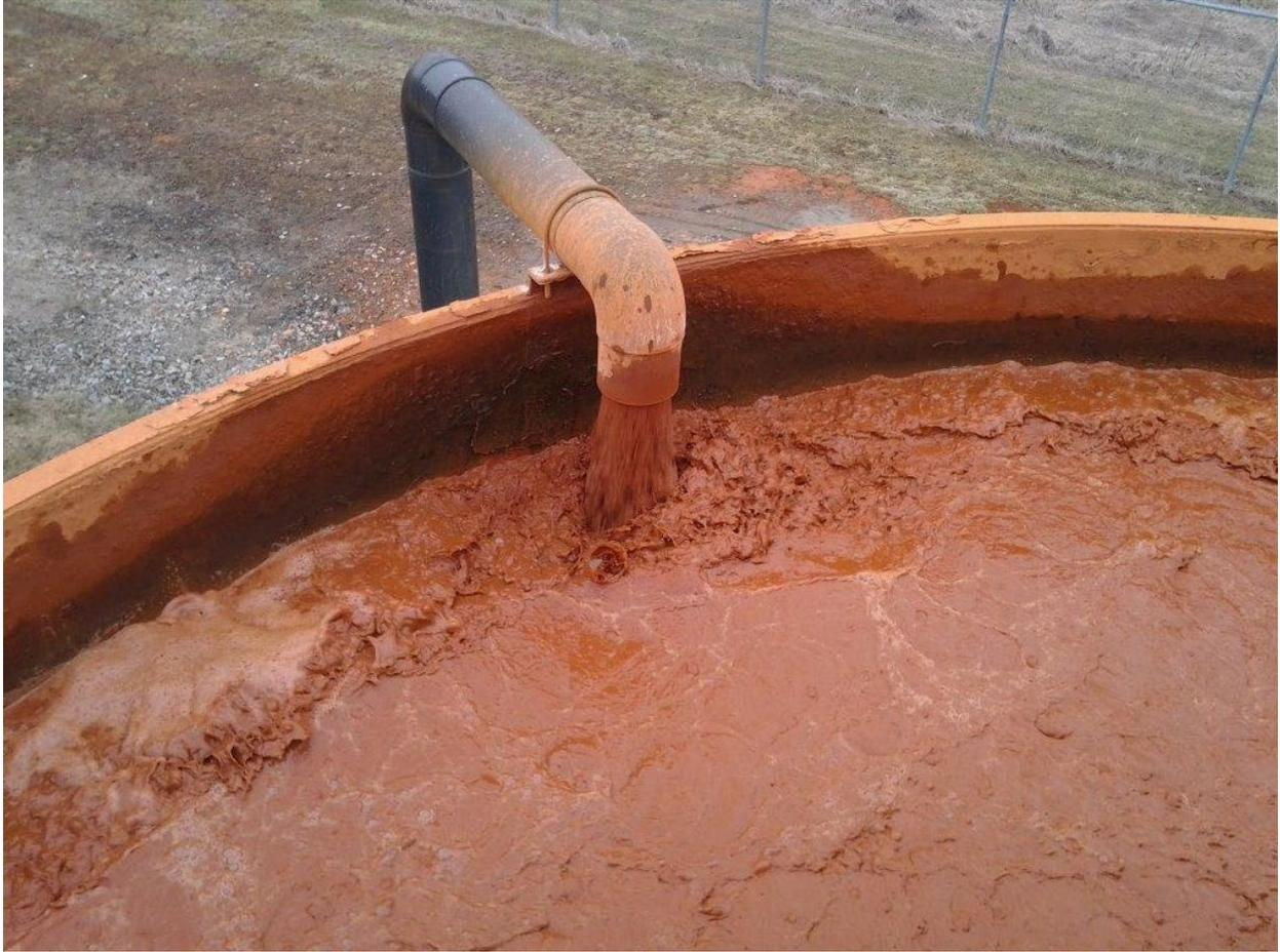
Figure 45: Photo showing sludge injected in the underground mine is being captured by the raw water pump and recirculated with the raw water back to the reaction tank. See caption in Figure 44.
