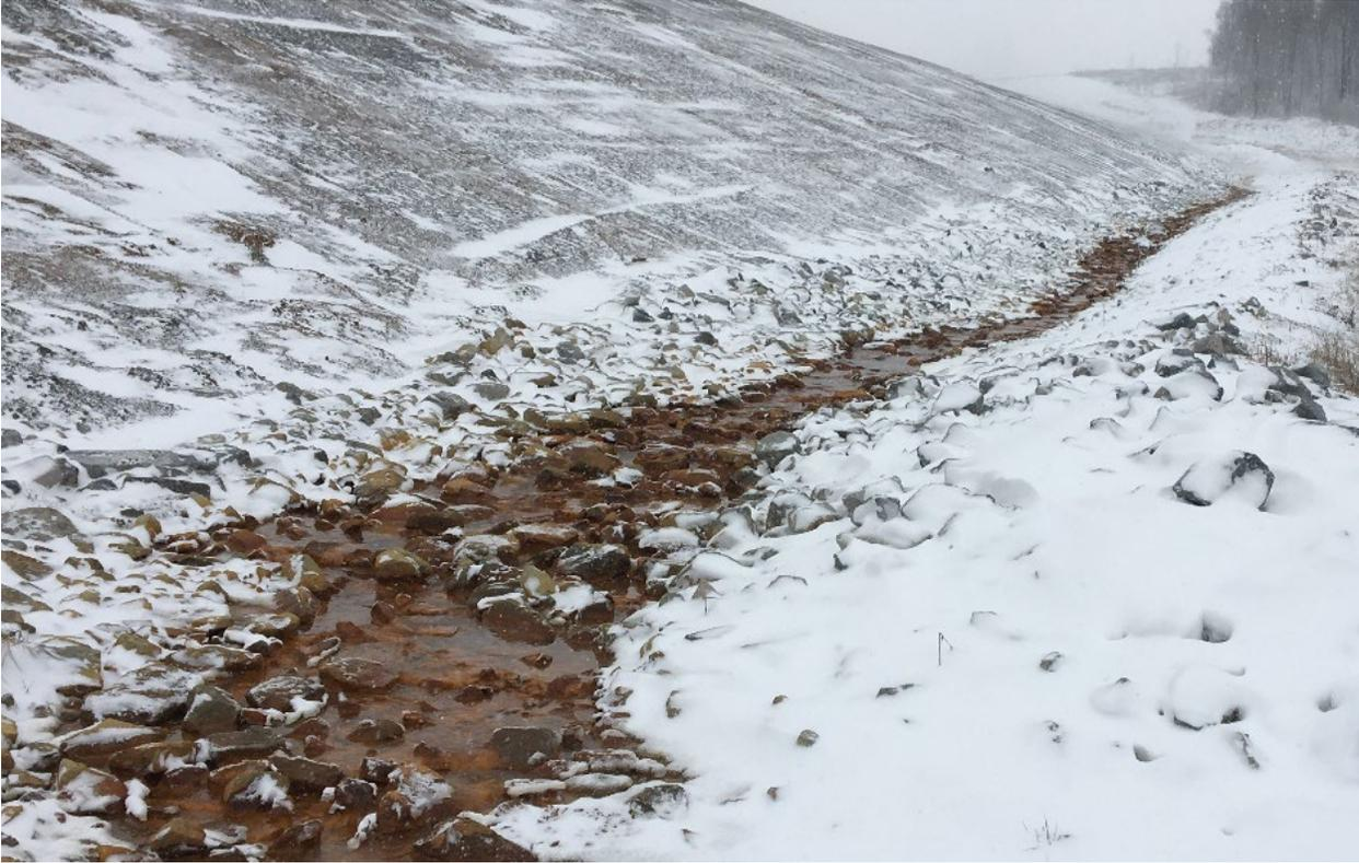
Figure 5: Photograph of Aggregate-lined ditch.
