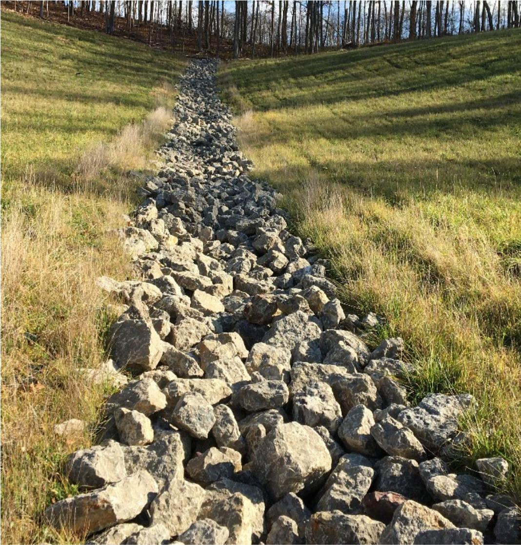
Figure 4: Photograph of Aggregate-lined ditch.
