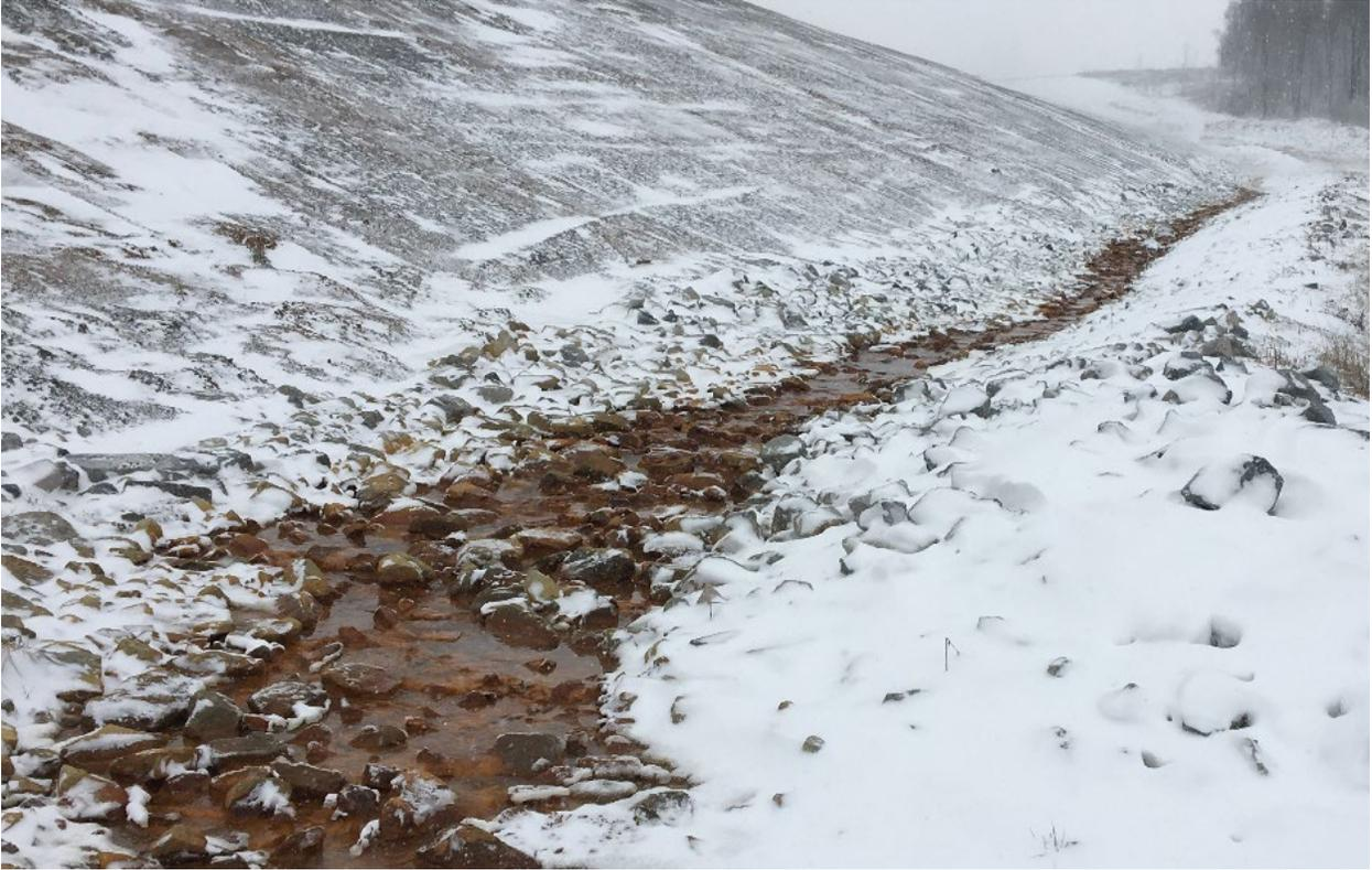
Figure 5: Photograph of Aggregate-lined ditch.
