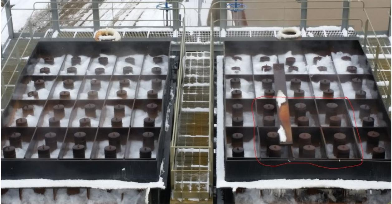
Figure 21: Notice reduced water levels within the red box of the Maelstrom on the right side of the photo. The reduced airflow reduces the water elevation and is a sign the stainless steel air nozzle banks are clogged and require cleaning.
