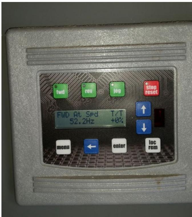
Figure 24: Variable Frequency Drive control panel provides the ability to control the blower output. This provides the ability to alter the decarbonation/horsepower ratio to optimize treatment costs.
