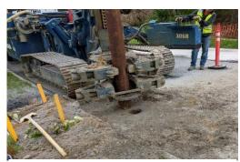
Installation of grout pillars to create a bulkhead underground.
