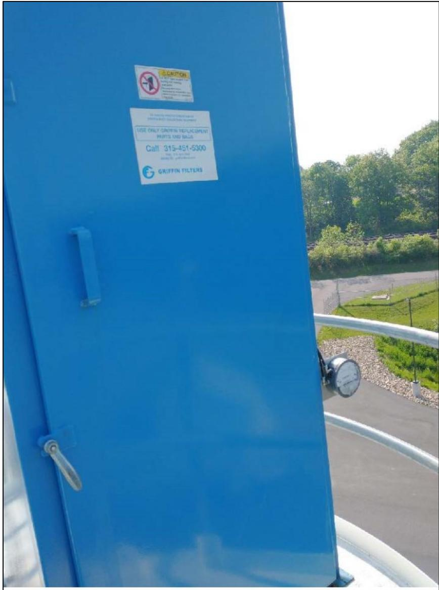
Figure 11: Access to filter bag house to maintenance and replace filters on top of silo
