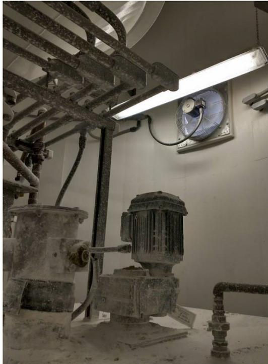
Figure 20: Mixer motor on top of Hydrated Lime slurry tank used to mix the hydrate with water. Note exhaust fan near top of photo to improve air quality within the skirt of the lime silo.
