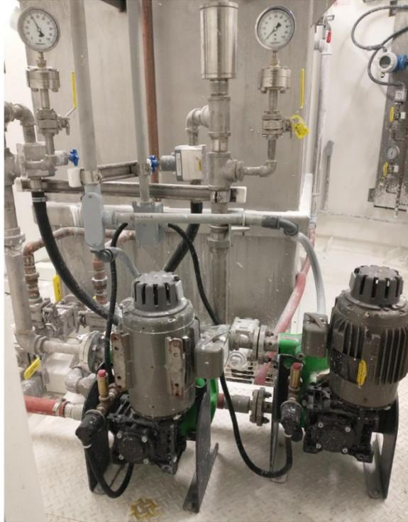
Figure 16: Pumps used to pump Hydrated Lime slurry from the slurry tank, located under silo, through the red hose and to the dose point.
