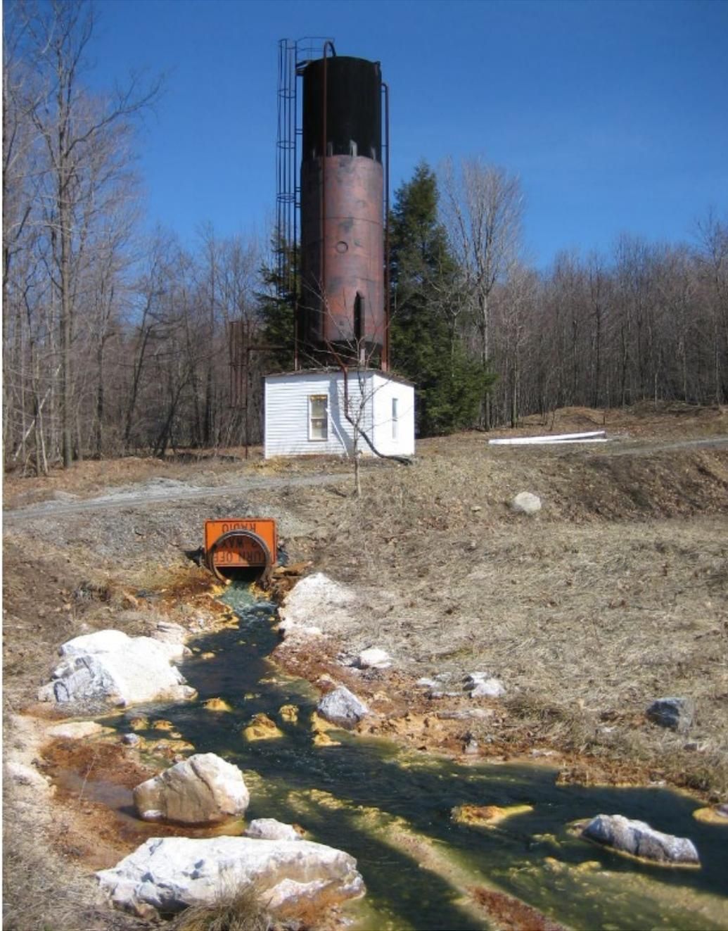
Figure 14: Simple hydrate system positioned overtop of a mine discharge to dry feed lime directly into the drainage flowing under the white building. A rock channel is used to create turbulence to aid in mixing and dissolving the lime into the drainage. Note the green ferrous iron hydroxide indicating the treatment pH is  $> 8.3$ .
