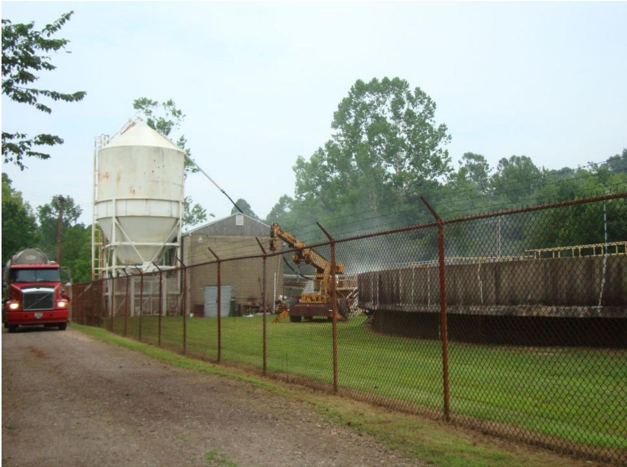
Figure 7: A 23-ton semi-truck pneumatically filling a 50-ton silo with hydrated lime. Note the fill line along the left side of the photo. Also, the fill line can be seen through the fence that connects the truck to the silo. Note the air exhaust line extending from the top of the right-hand side of the photo down to the reaction tank where the line is submerged to during filling to control lime dust. This 1960s-era silo lacks a filter bag air purification system onto of the silo.
