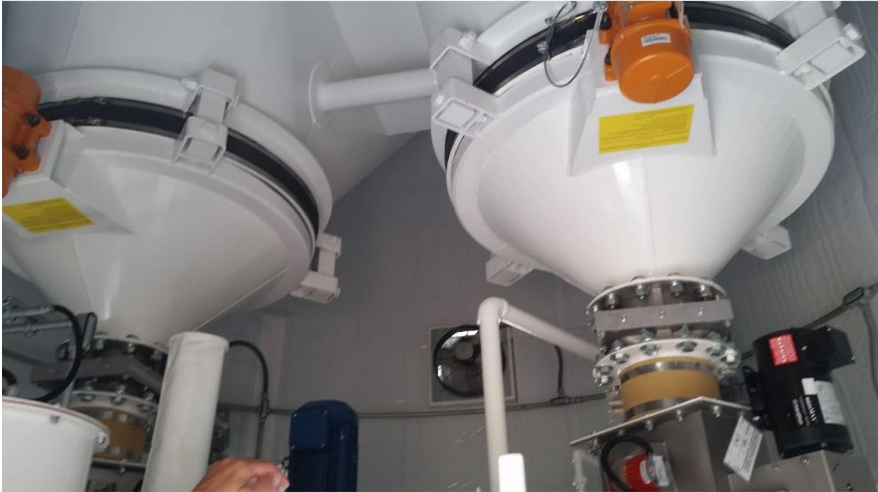
Figure 12: Photo of dual silo cones beneath a 120-ton silo. The dual cones and hydrate feeder system provides redundancy incase the feeder system malfunctions. Note the orange 1-HP bin vibrator motors that vibrate the base of the silo to prevent lime from compacting and “bridging” across the base. The motors are time to vibrate the base of the silo for 30-secs every 5 minutes. The timers are adjustable.
