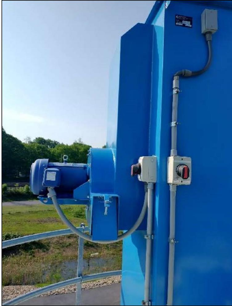
Figure 10: Alternative view of dust collection system on top of the silo. Motor and filter bags in blue housing remove hydrated lime exhaust dust during the filling of the silo.
