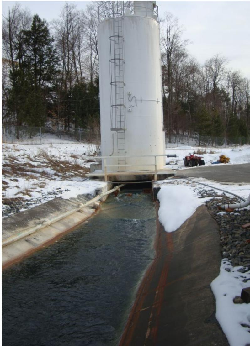
Figure 13: Hydrated Lime silo and dispensing system “dry feeding” hydrate directing into mine drainage flowing underneath the system. This eliminates the need to make a slurry and pump a hydrate slurry to the dose point. Attention is required to ensure moisture from mine drainage doesn’t redecarbonate hydrate and cause feeding issues.
