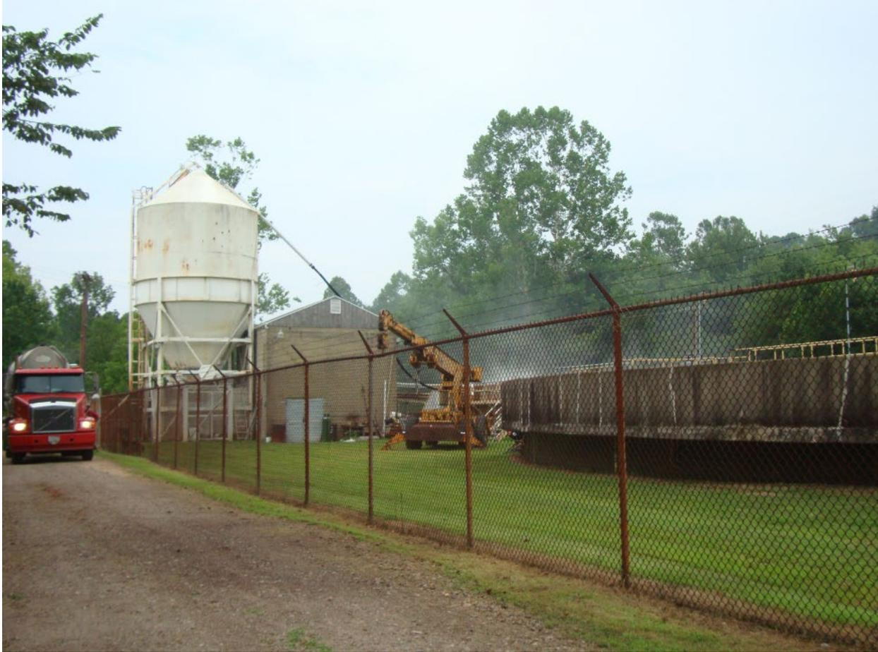
Figure 7: A 23-ton semi-truck pneumatically filling a 50- ton silo with hydrated lime. Note the fill line along the left side of the photo. Also, the fill line can be seen through the fence that connects the truck to the silo. Not the air exhaust line extending from the top of the right-hand side of the photo down to the reaction tank where the line is submerged to during filling to control lime dust. This 1960s-era silo lacks a filter bag air purification system onto of the silo.
