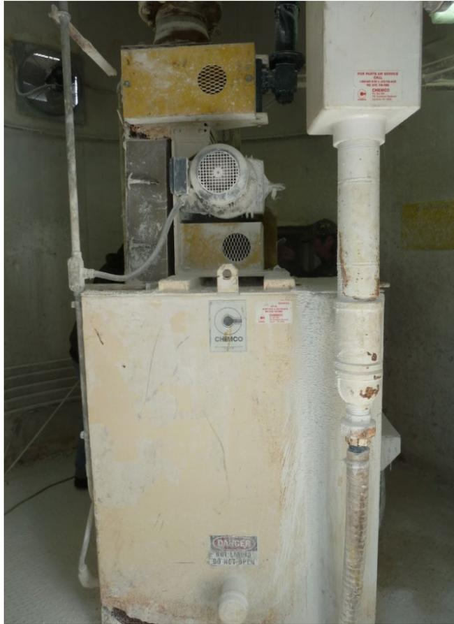
Figure 15: Volumetric screw feed, hydrated lime slurry tank, and mixer positioned under the silo. Hydrated Lime and water are mixed in the slurry tank and pumped to the dose point.
