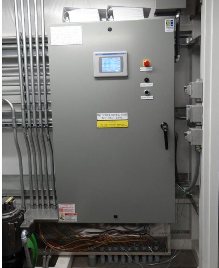
Figure 18: Electrical control panel located inside silo and controls slurry make up and pumping.
