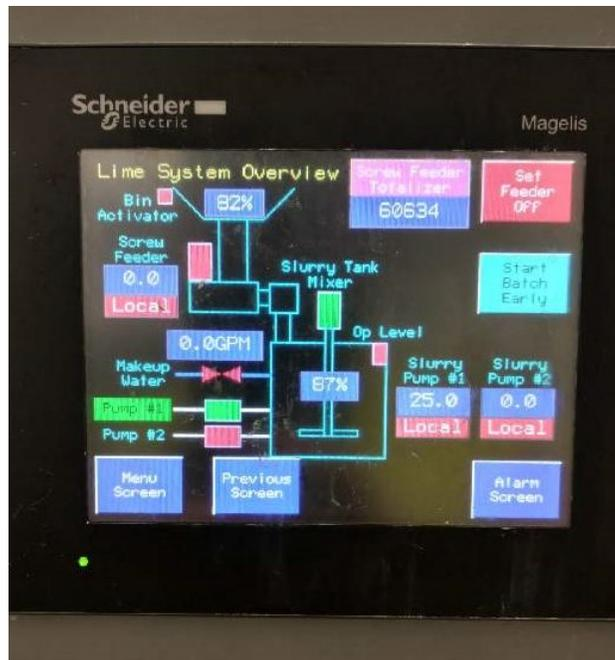
Figure 19: Close up of the touch screen attached to the face of the electrical control panel shown in Figure 18.
