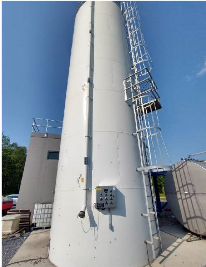
Figure 8: 50-ton turn-key hydrated lime silo with bottom skirt that houses bin vibrators, electrical control panel, slurry tank, slurry mixers, slurry pumps, and electrical control panel (shown on silo). Note the fill line that connects to semi-trucks to pneumatically push 23-tons of hydrated lime up and into the top of the silo.
