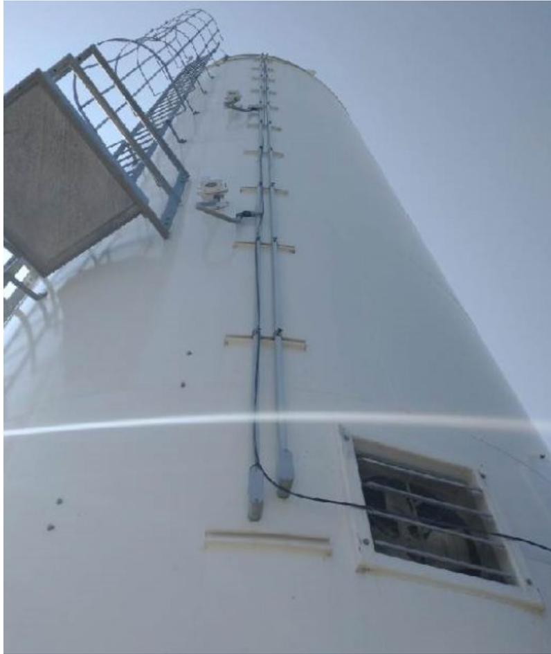
Figure 21: Exhaust fan shown near bottom of silo to remove hydrate dust and improve air quality within the silo skirt.
