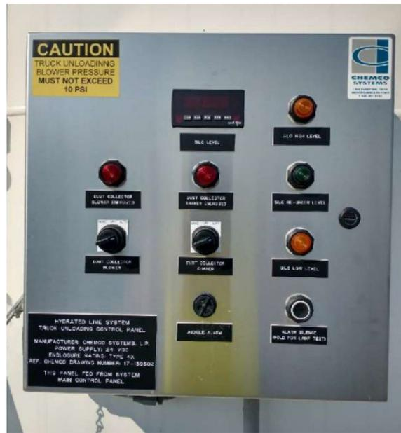
Figure 17: Electric control panel that controls dust collection bag filters that sit on top of silo and low and high silo fill alarms. This control panel is attached to the outside of the silo and operated when the silo is filled.
