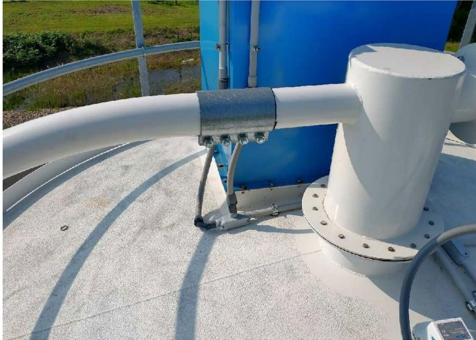
Figure 9: Photo of the fill line entering the top of the silo. Semi-Trucks carry approximately 23 tons of Hydrated Lime attach to the bottom of the fill line and pneumatically push the lime to the top of the silo. Note the blue housing that contains bag filters used to the evacuated exhaust air as lime is pushed into the silo during filling.
