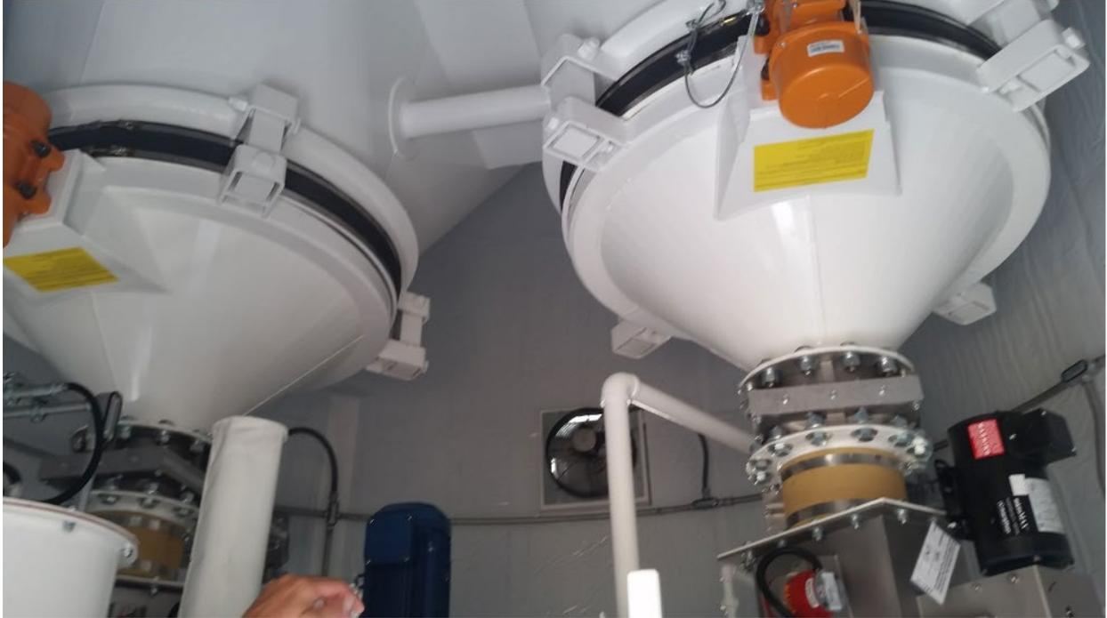
Figure 12: Photo of dual silo cones beneath a 120-ton silo. The dual cones and hydrate feeder system provides redundancy in case the feeder system malfunctions. Note the orange 1-HP bin vibrator motors that vibrate the base of the silo to prevent lime from compacting and “bridging” across the base. The motors are timed to vibrate the base of the silo for 30-secs every 5 minutes. The timers are adjustable.
