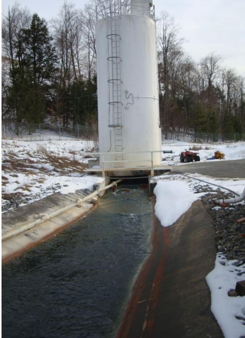
Figure 13: Hydrated Lime silo and dispensing system “dry feeding” hydrate directing into mine drainage flowing underneath the system. This eliminates the need to make a slurry and pump a hydrate slurry to the dose point. Attention is required to ensure moisture from mine drainage doesn’t redecarbonate hydrate and cause feeding issues.
