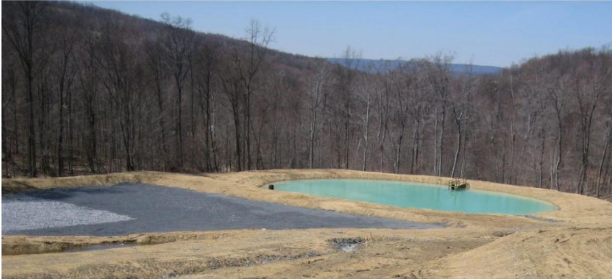
Figure 8: A newly constructed limestone bed (left) constructed with a dosing siphon. The system acts as a batch reactor that fills with mine drainage until a pre-determined elevation is achieved that triggers the dosing siphon to drain the system to a settling pond. The aquamarine color of the settling pond is caused by suspended aluminum flushing to the pond.
