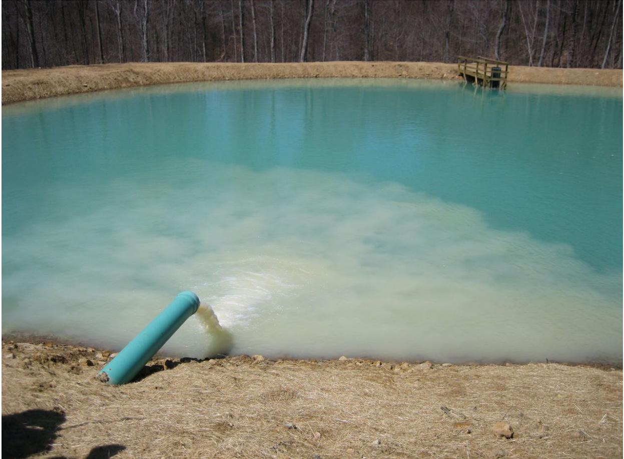
Figure 10: Aluminum Hydroxide being flushed from a Limestone Bed to a settling pond after the water level tripped the dosing siphon
