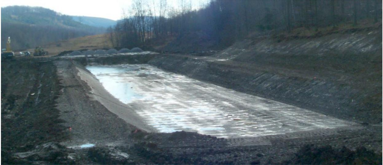
Figure 5: Graded footprint of limestone bed. Piles of limestone seen in the background.
