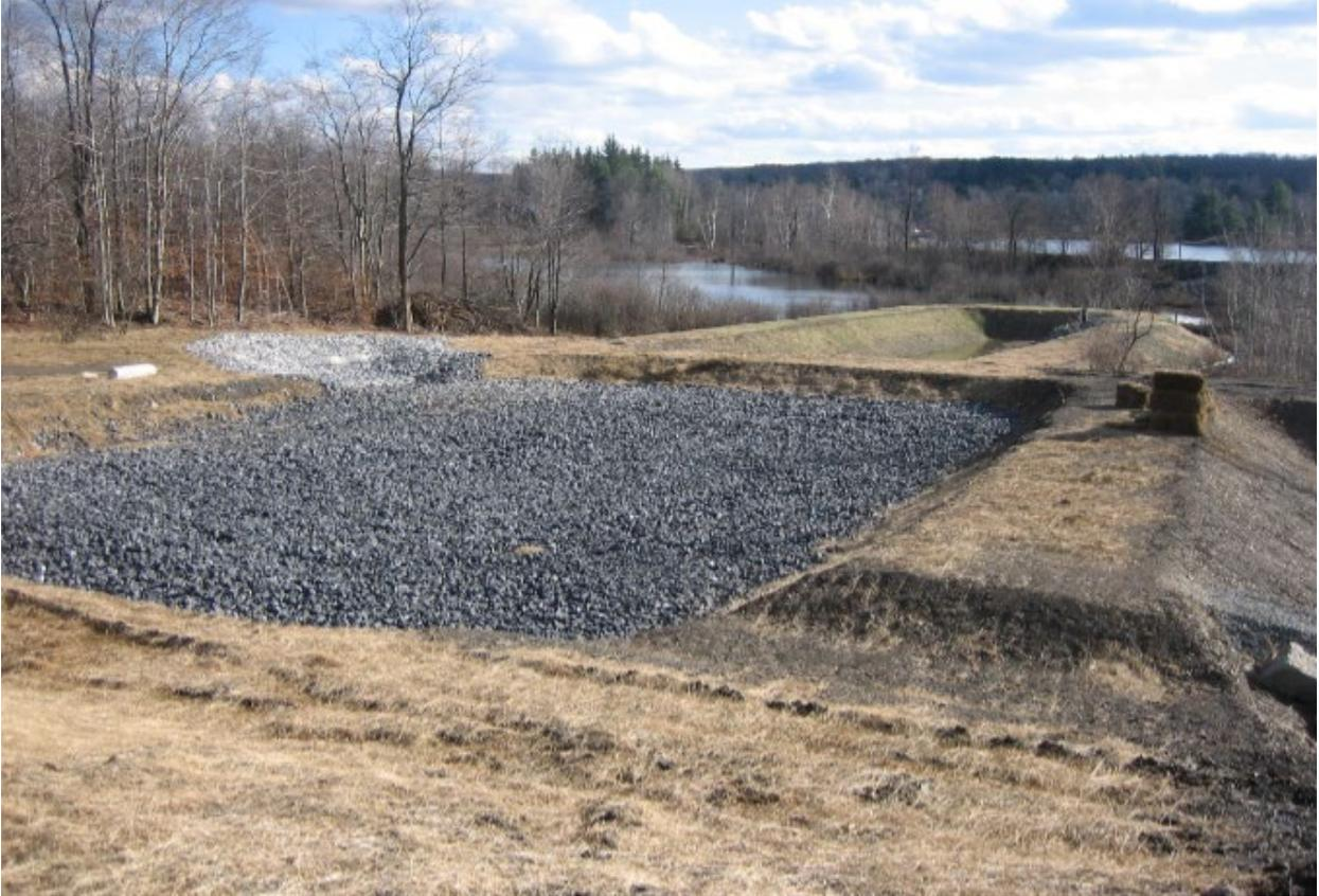
Figure 6: Newly constructed Limestone bed before being filled with mine drainage.
