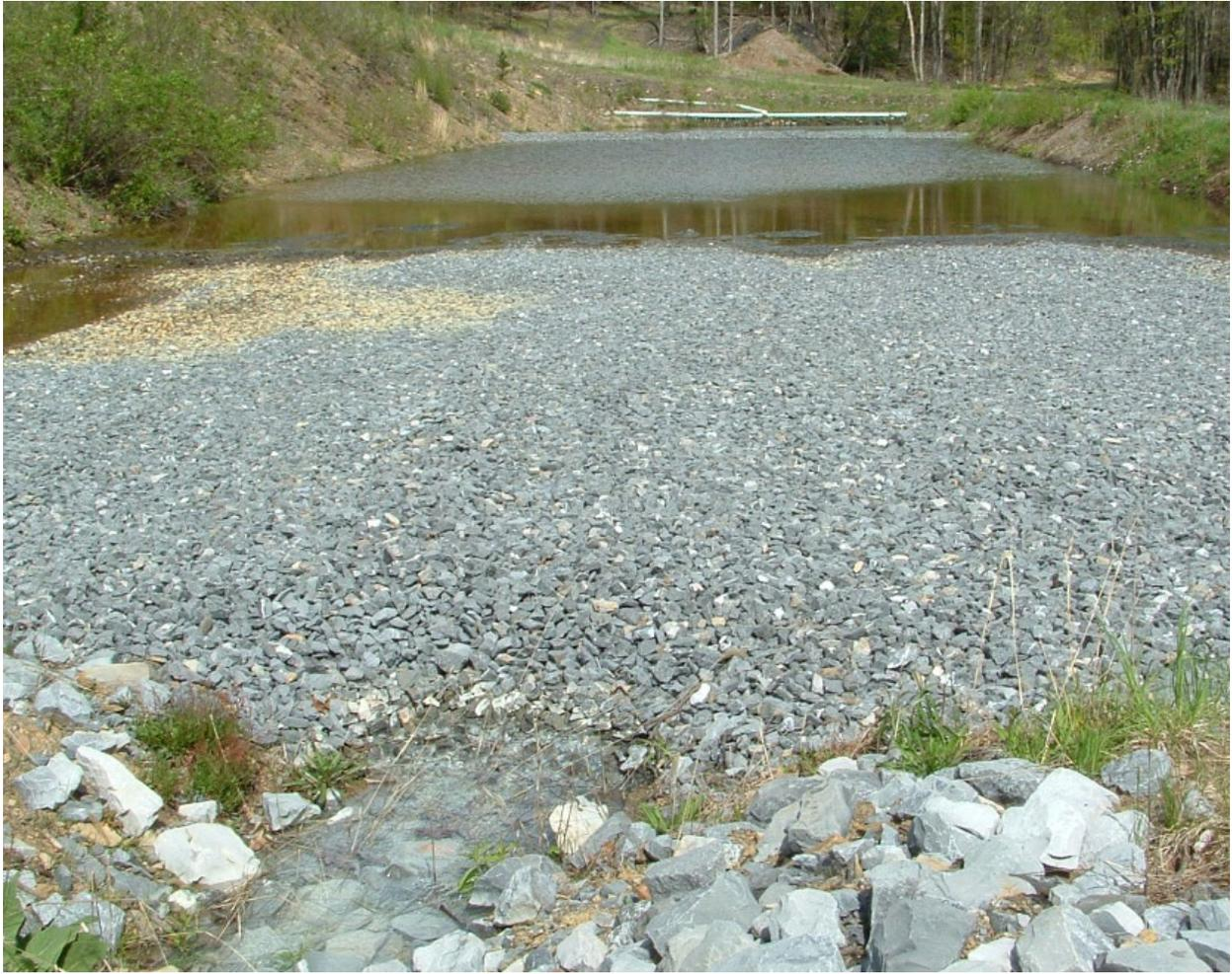
Figure 7: A limestone bed constructed with a focus on easy maintenance and not using a piping network to continuously flush the system to remove precipitates. Water flows into the system from the piping manifold seen in the background and water exits in the foreground.
