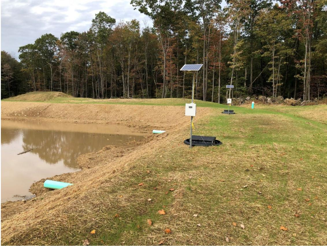
Figure 9: An “Agri Drain Smart” water control structure is shown enclosed by the black corrugated pipe. The solar-powered system can be set using the programmable logic controller (PLC) contained within the white box on the post to drain the limestone bed once a week and for a specified duration. The control box powers an actuator that opens and closes a gate valve to drain (flush) the system contained within the water level control structure in the embankment.
