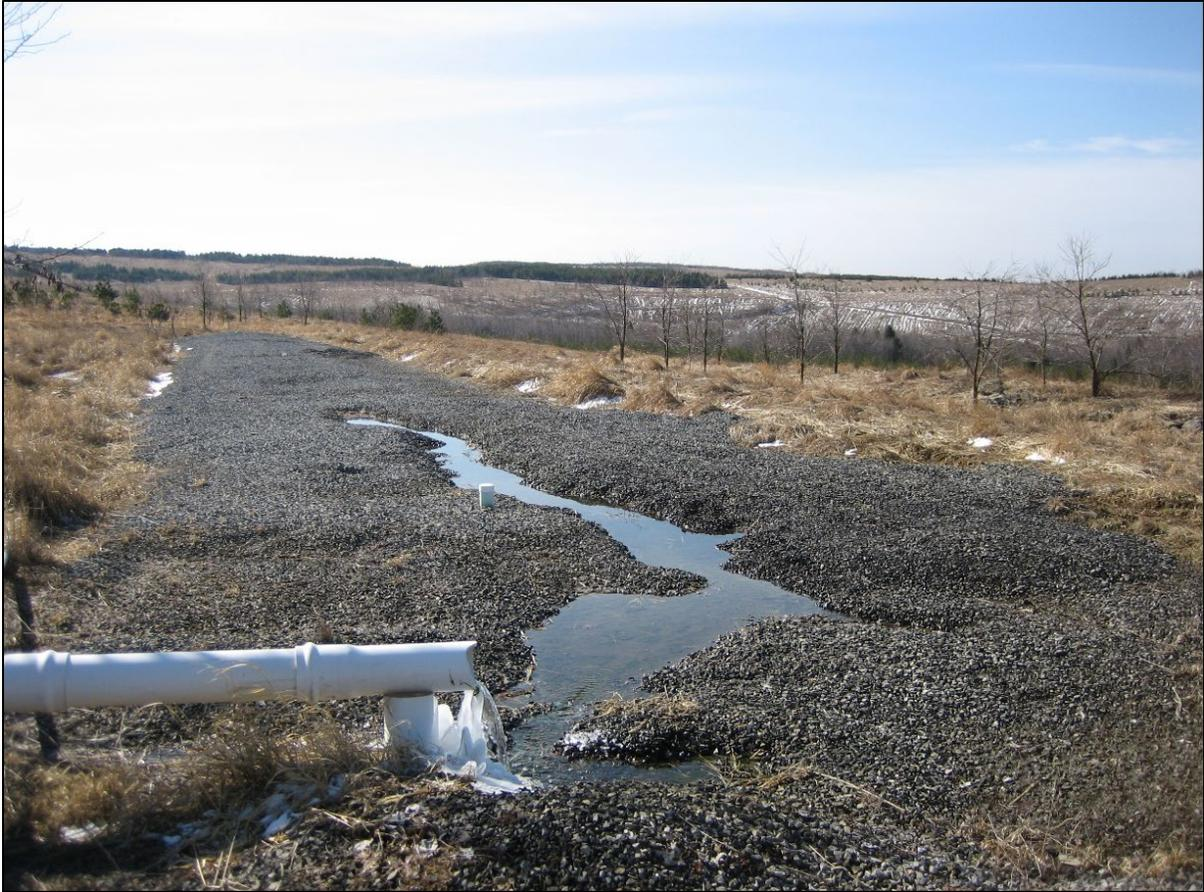
Figure 5: A manganese removal bed that has achieved less than 0.1 mg/L for over 20 years with minimal maintenance. Most of the maintenance involves using a mechanical excavator to break up the manganese scale at the beginning of the bed. A small depression trench was installed here to permit the build up of hydraulic head to force the water into the stone. This bed treats 20 gpm and a raw manganese concentration of 30 mg/L using a uniform sized  $\frac{3}{4}$ " limestone.
