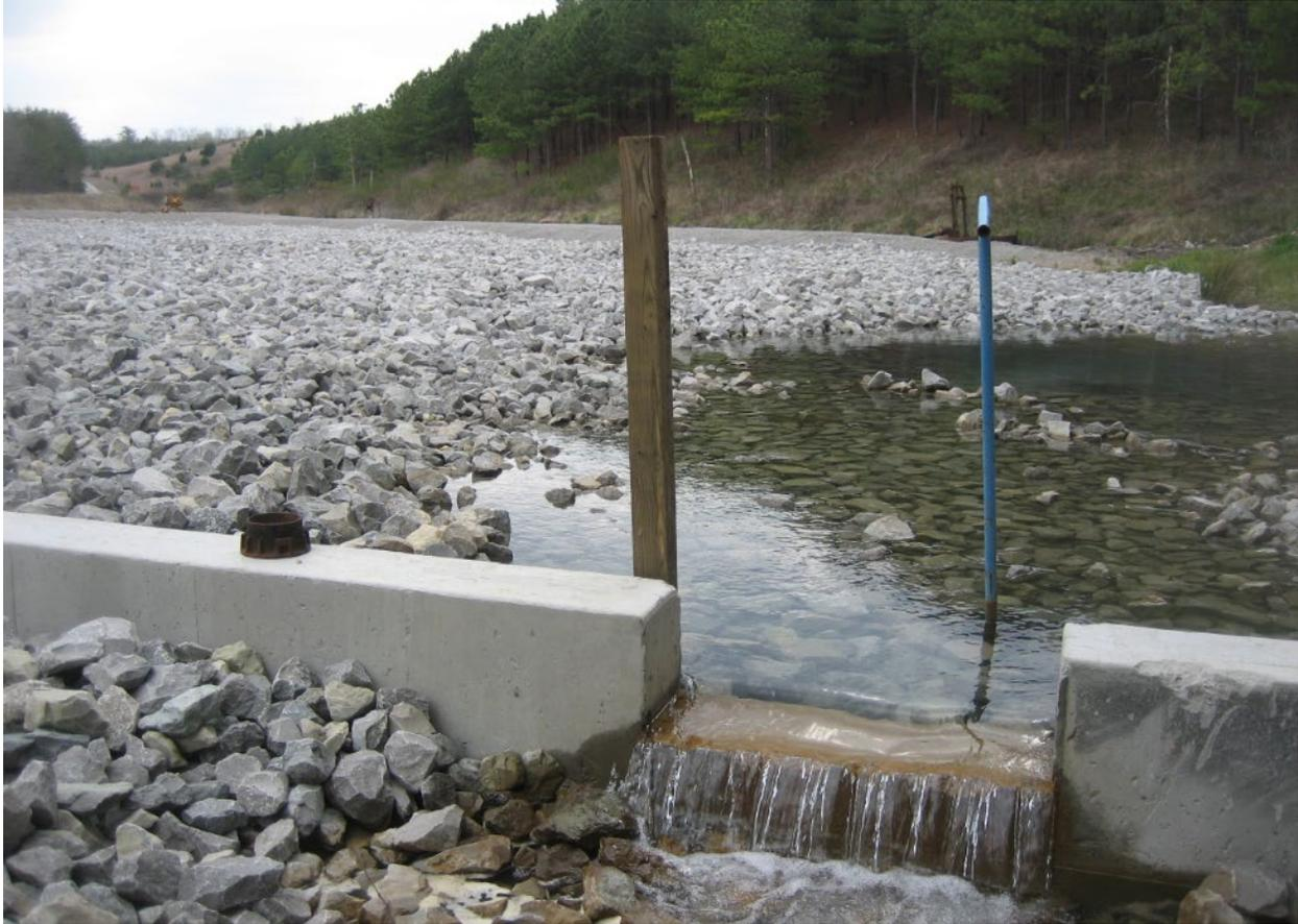
Figure 6: This large MRB was used to treat a flow of 600 gpm containing a manganese concentration of 8 mg/L. The bed contained more than ten thousand tons of limestone ranging in size from 4 to 6 inches.
