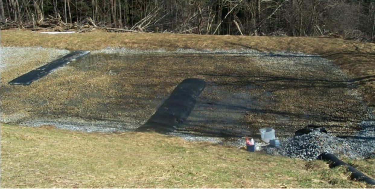
Figure 7: MRB showing blackish-brown manganese coated limestone. Influent pipe shown at bottom right and large baffle used to prevent short circuiting.
