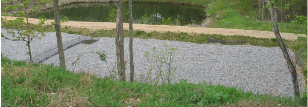
Figure 4: Manganese removal bed treating 60 gpm flow on the Flight 93 Memorial grounds near Somerset, Pa. The open-water trench is used to reoxygenate the water to facilitate manganese removal.
