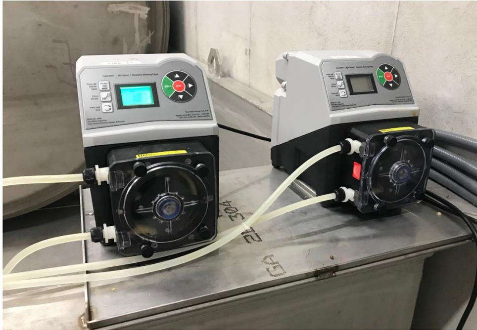
Figure 7. Photo of a Dosing Skid with Two Pumps.
