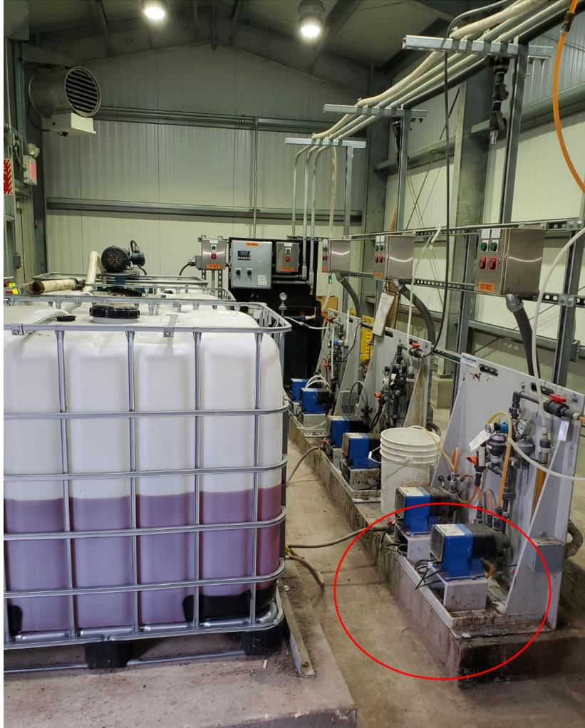
Figure 6. Photo of a Dosing Skid with Two Pumps in Red Circle. The chemical storage containers (tote) would represent the Non-Bulk Container for Sodium Permanganate.
