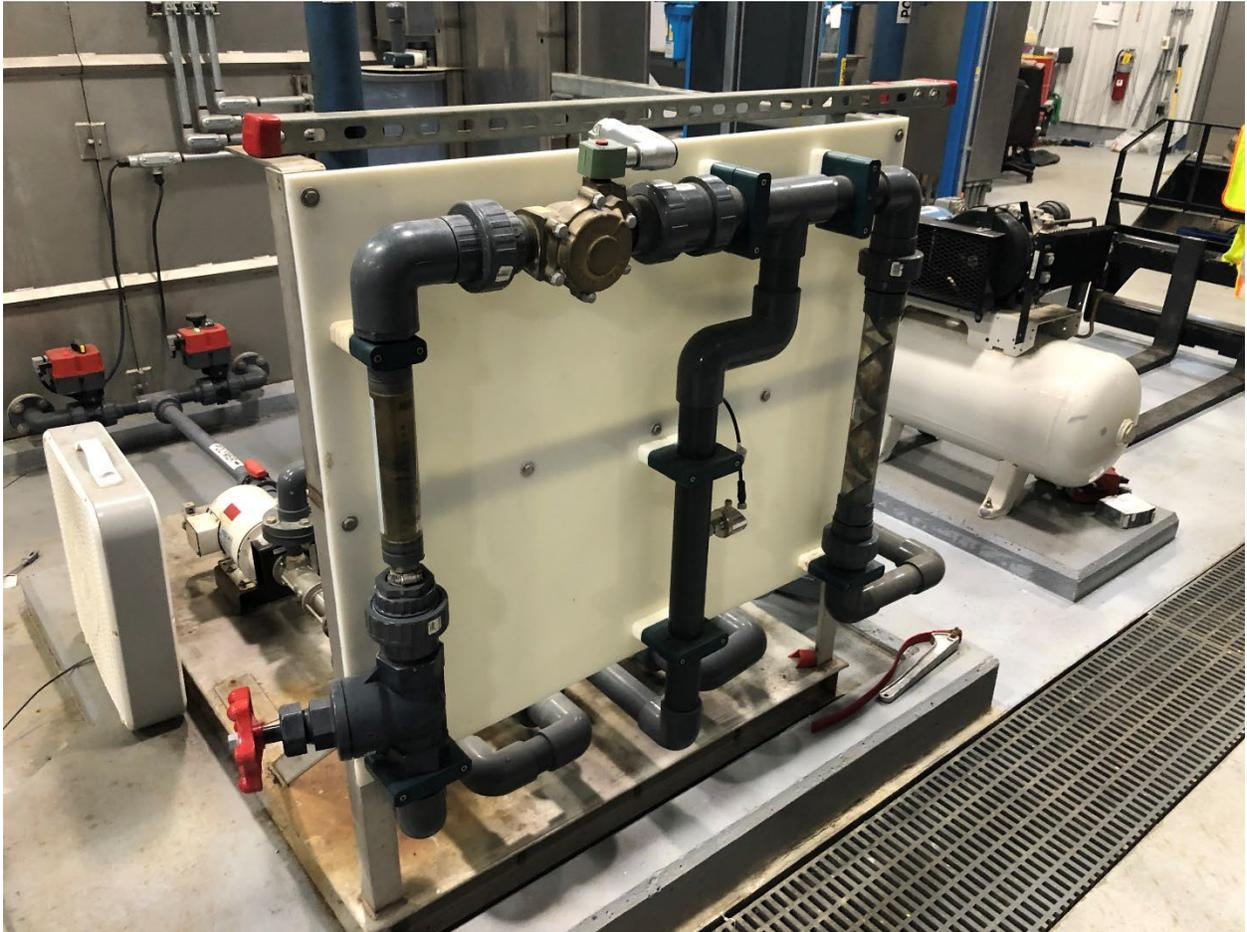
Figure 6. Pumps and inline static mixers for mixing the made down polymer solution with push (dilution) water prior to addition to the mine drainage source.
