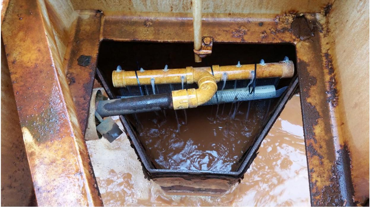
Figure 8. Application point of polymer into the mine drainage at a treatment facility.
