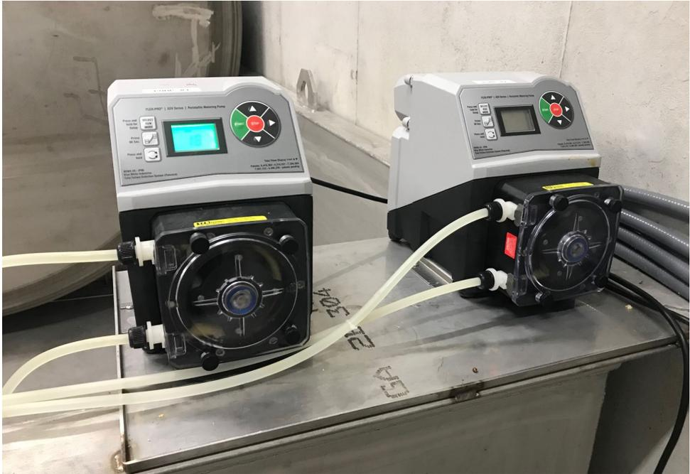
Figure 7. Photo of two pumps as part of the dosing skid component of a dry polymer automatic system.
