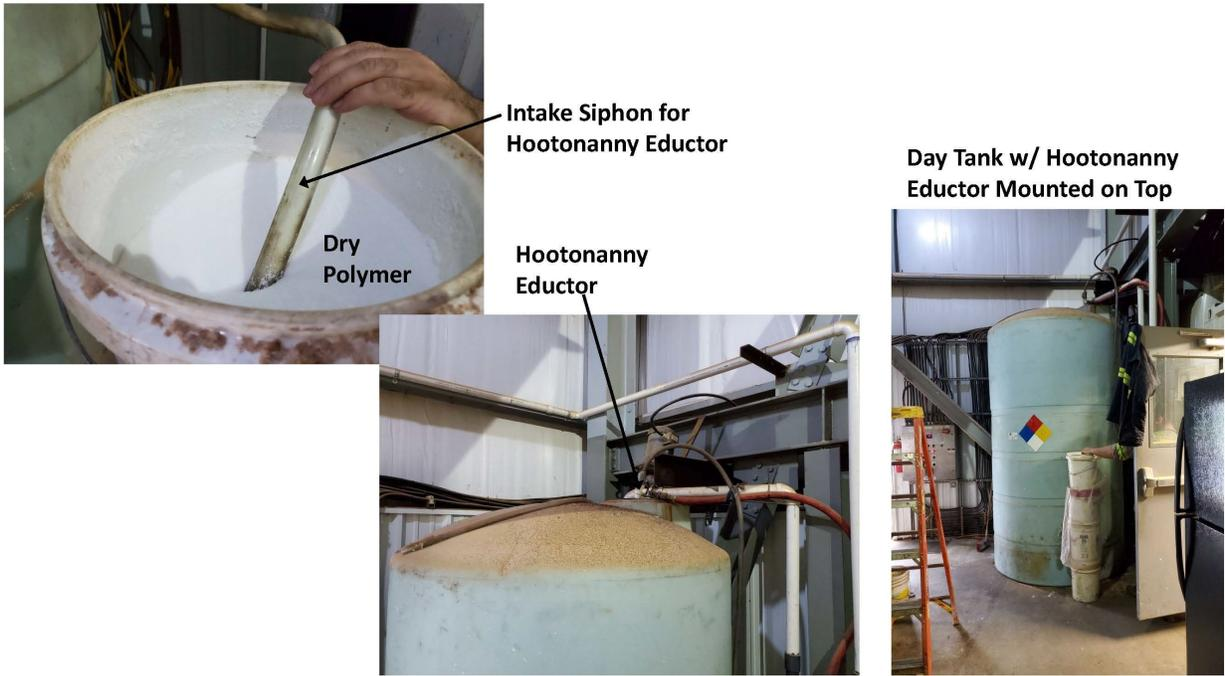
Figure 4. Manual make down of dry polymer into day tank using Hootonanny Eductor system on top of tank at a mine drainage treatment facility.
