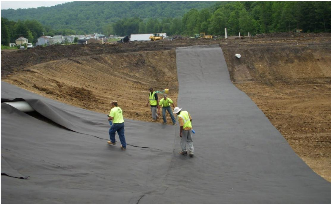
Figure 9. Photo of liner being installed on inside embankments and bottom of pond.
