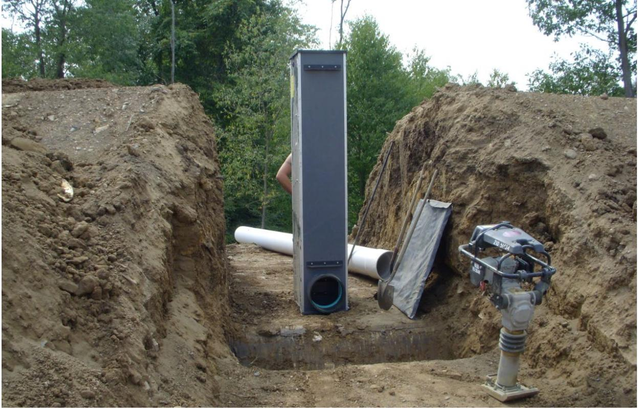
Figure 11. Agri Drain water level control structure being installed during construction of a passive treatment system.
