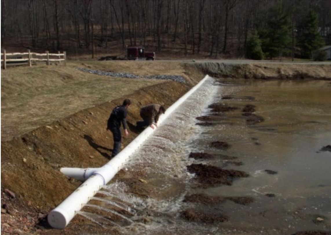
Figure 4: Influent piping configuration commonly used to distribute flow across the width of the pond to promote uniform flow distribution.
