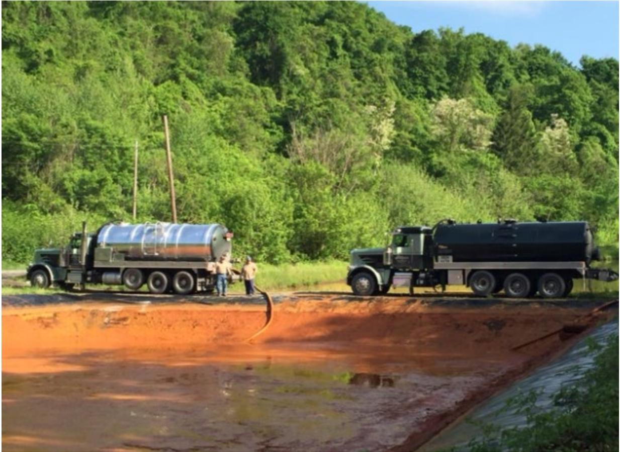
Figure 15: Vacuum trucks removing sludge from a pond.
