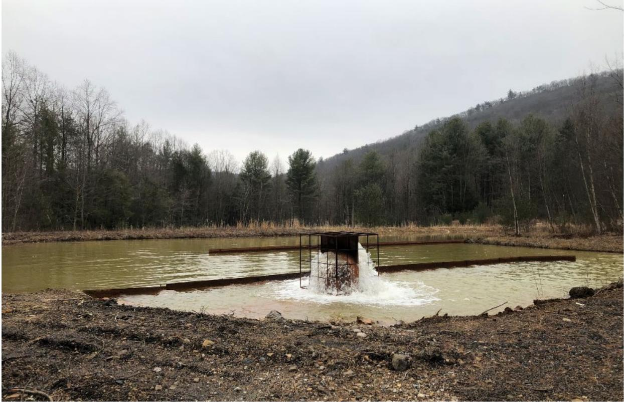
Figure 6: Pond with raised standpipe promoting the aeration at the inlet of the pond.
