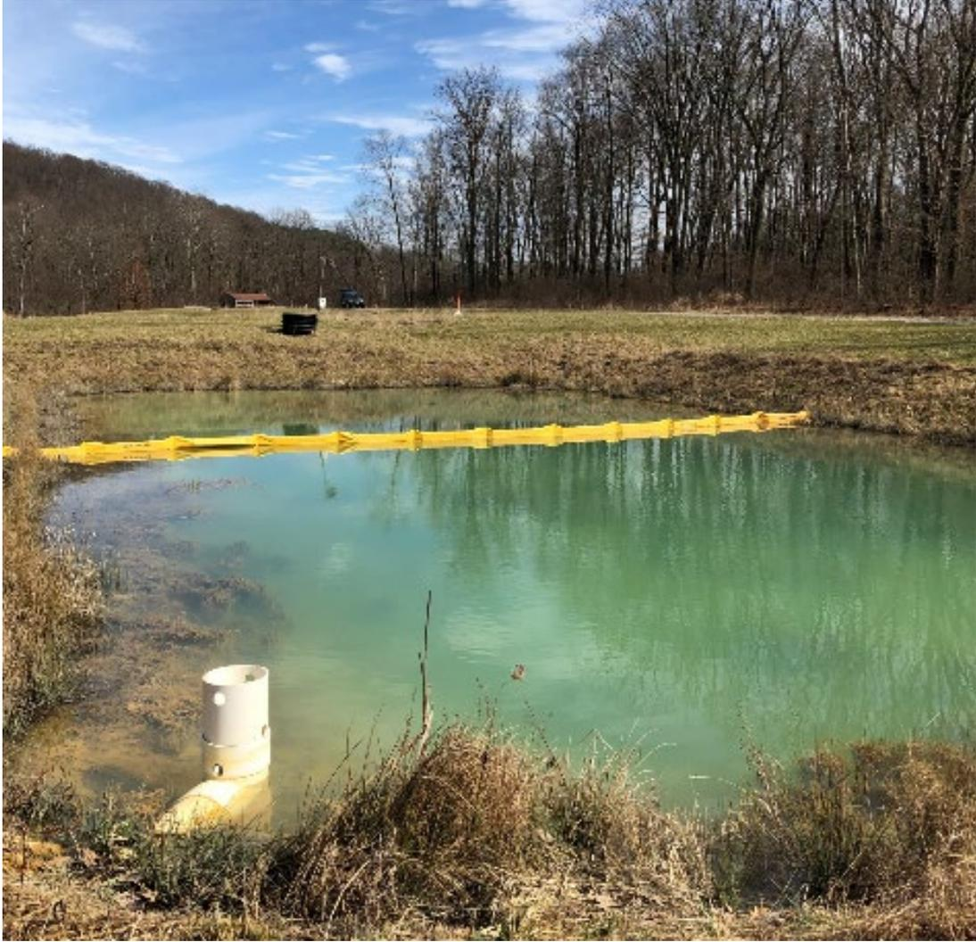
Figure 7: Pond with a floating baffle across the width of the pond.
