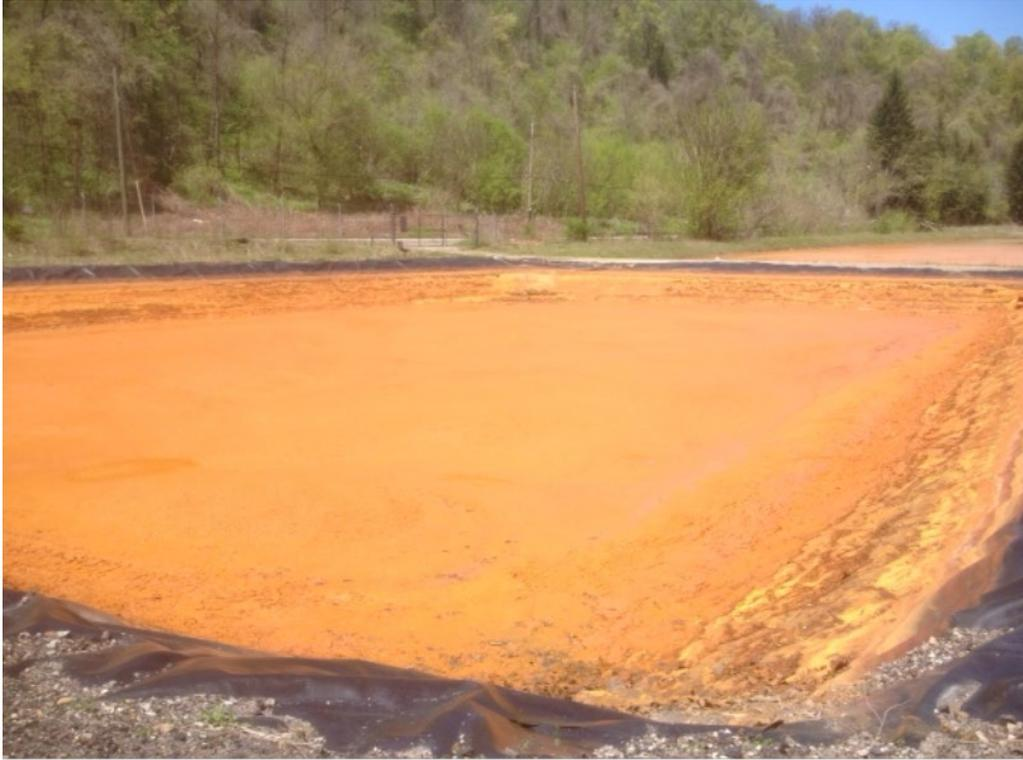
Figure 12: Photo of pond with liner with oxidized iron settled out in pond.
