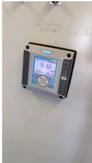
Figure 8: pH Controller (Hach 200) for lime slurry metering/dosing pumps
