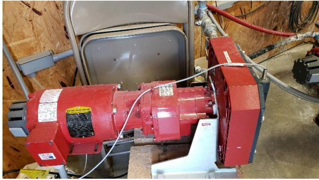
Figure 6: Two examples of lime slurry metering/dosing pumps
