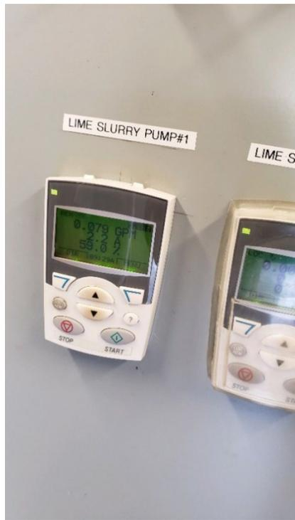
Figure 7: VFD Control units for lime slurry metering/dosing pumps
