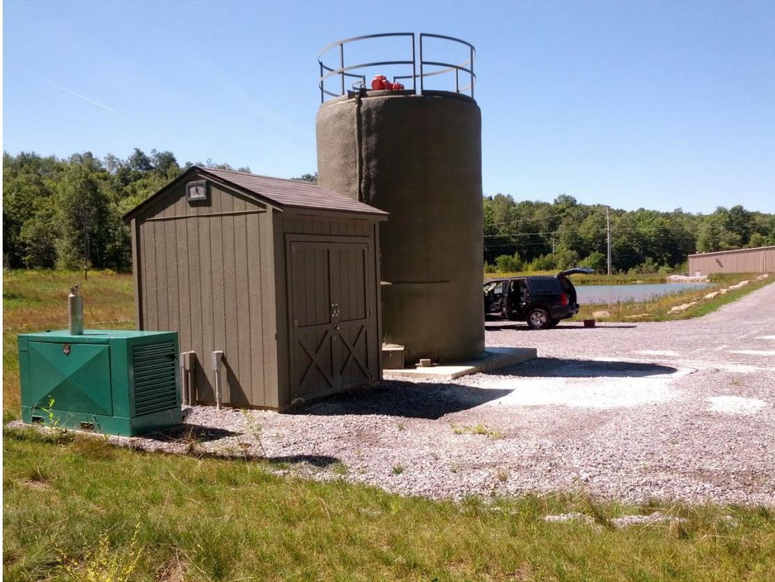
Figure 4: Pre-manufactured Lime slurry system in use at a PA Bituminous Mine Site. 8800 gallon insulated storage tank, shed for dosing pump and electrical controls and a standby diesel generator.
