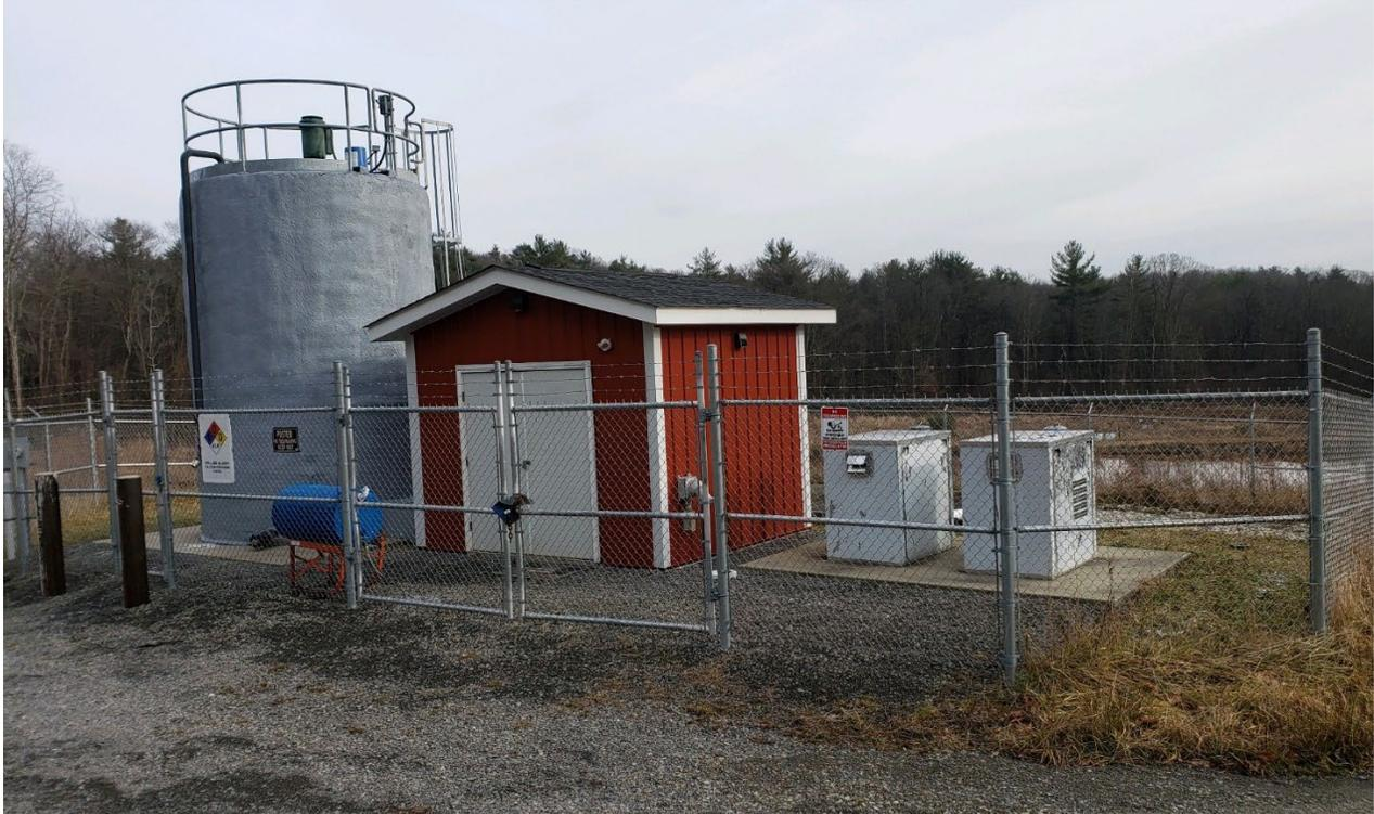
Figure 5: Pre-manufactured Lime slurry system in use at a Northern PA Bituminous Mine Site. 8800-gallon insulated storage tank, shed for dosing pump and electrical controls. Blower units shown on the right-side concrete pad are used for a reaction tank.
