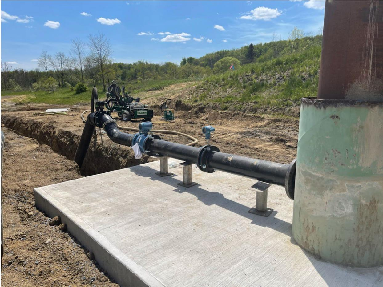
Figure 3. New installation for a Vertical Turbine Pump showing concrete pad, surface borehole casing, inner borehole casing and conveyance piping connection fittings at a mine site in Pennsylvania used to pump water from an underground mine pool to the surface for treatment at an active chemical treatment facility.
