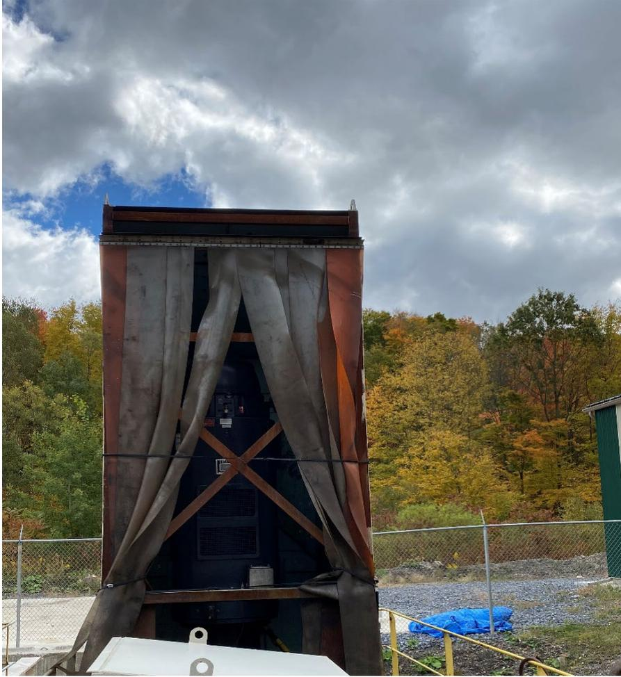
Figure 2. Vertical Turbine Pump housed in an enclosure for noise suppression and to reduce weathering at a mine site in Pennsylvania used to pump water from an underground mine pool to the surface for treatment at an active chemical treatment facility.
