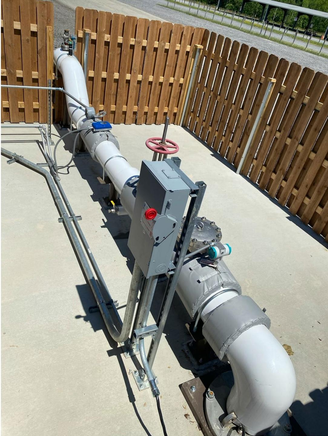
Figure 5. Concrete pad showing conveyance pipeline connection, electrical service and monitoring and telemetric equipment for a submersible turbine pump at a mine site in Pennsylvania used to pump water from an underground mine pool to the surface for treatment at an active chemical treatment facility.
