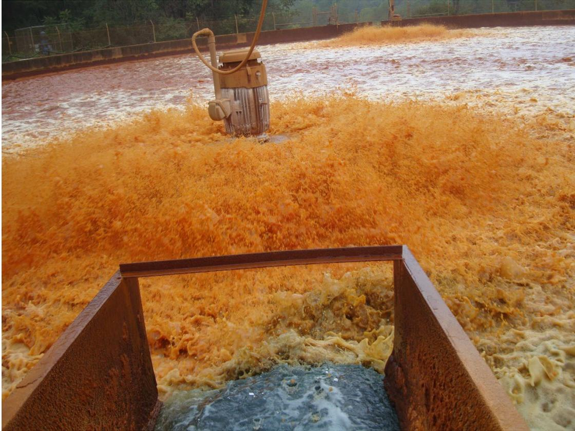
Figure 5: Surface Aerator in a large concrete CSTR Reaction Tank.
