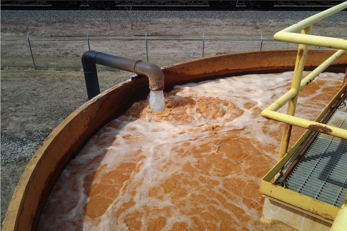
Figure 1: Steel CSTR Round Baffled Reaction Tank with a mechanical mixer.
