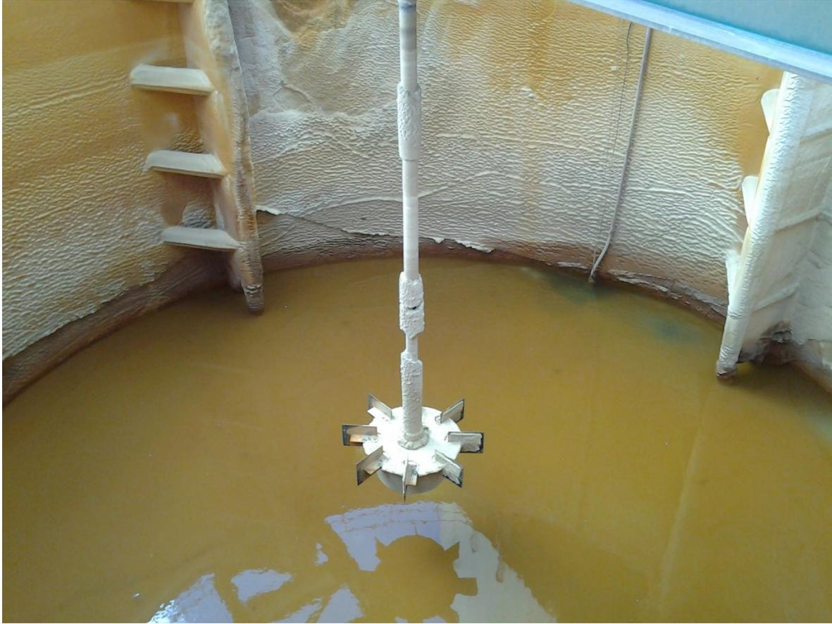
Figure 2: Concrete Reaction Tank showing baffles and mechanical mixer impeller. This is a western US hard rock mine site (Butte, Montana) Note - Calcite and Gypsum scaling issues.
