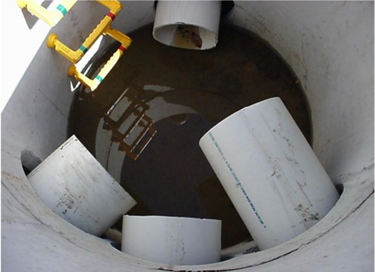
Figure 18. Inside view of Flow distribution structure. The untreated discharge enters through the bottom pipe and is distributed between the top three pipes that feed three VFPs in parallel.
