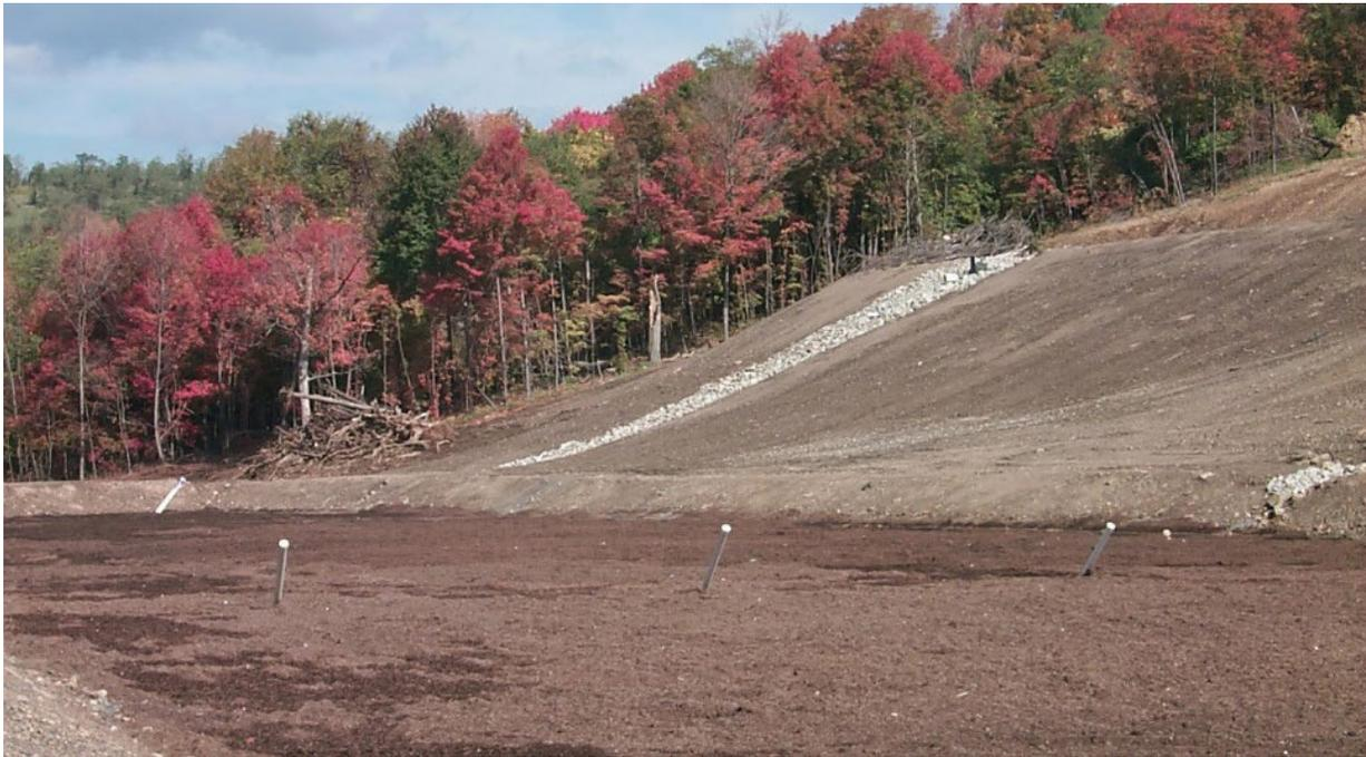
Figure 6: Constructed VFP after installation of compost layer. Vertical pipes are connected to underdrain system and used to maintenance underdrain pipes if clogging occurs. Clean out pipes are no longer typically used.
