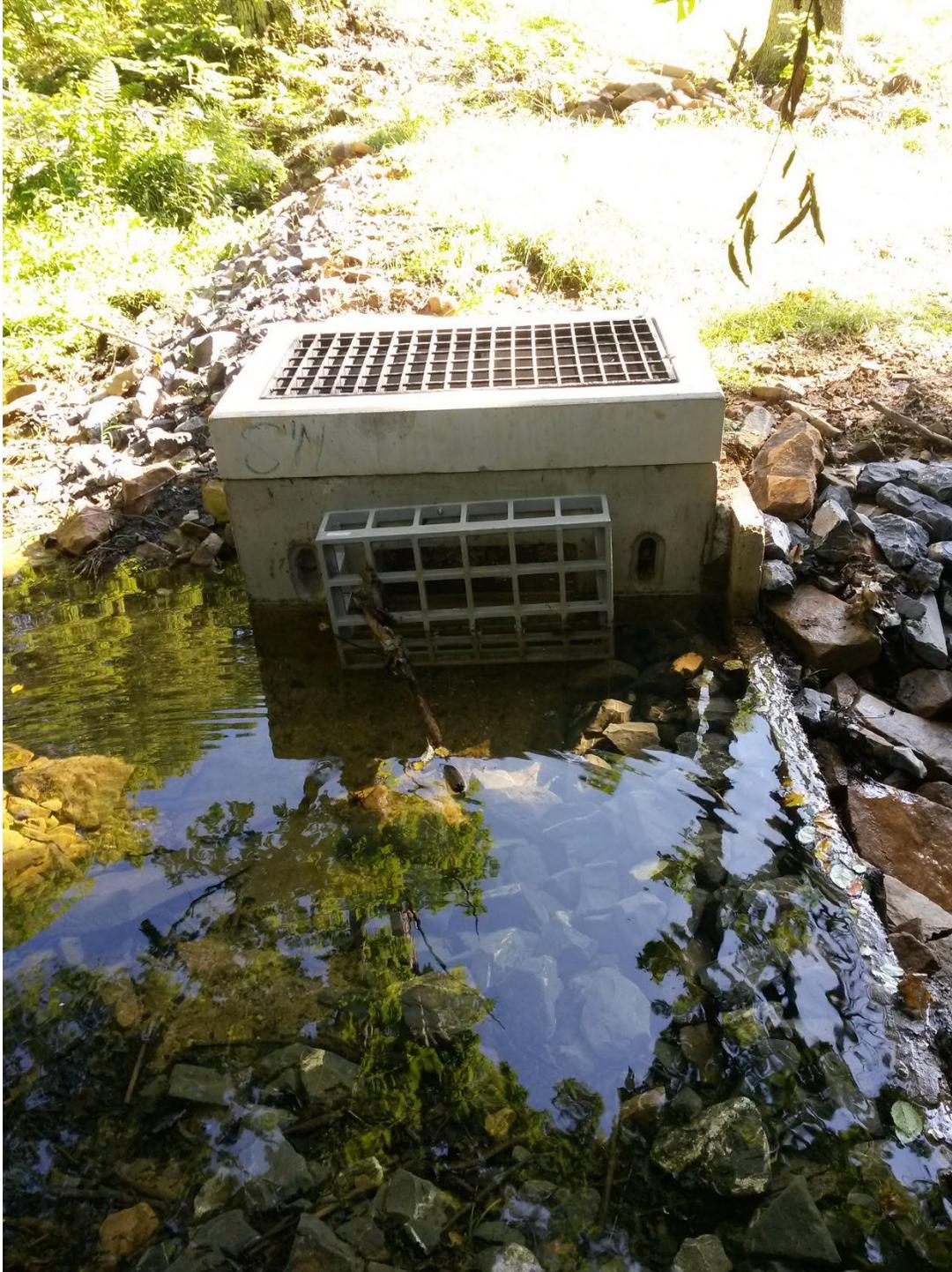
Figure 19 – Open Top Intake Structure with Weir. Water level is controlled by weir and baseflow is forced to flow through trashrack and into the intake structure.
