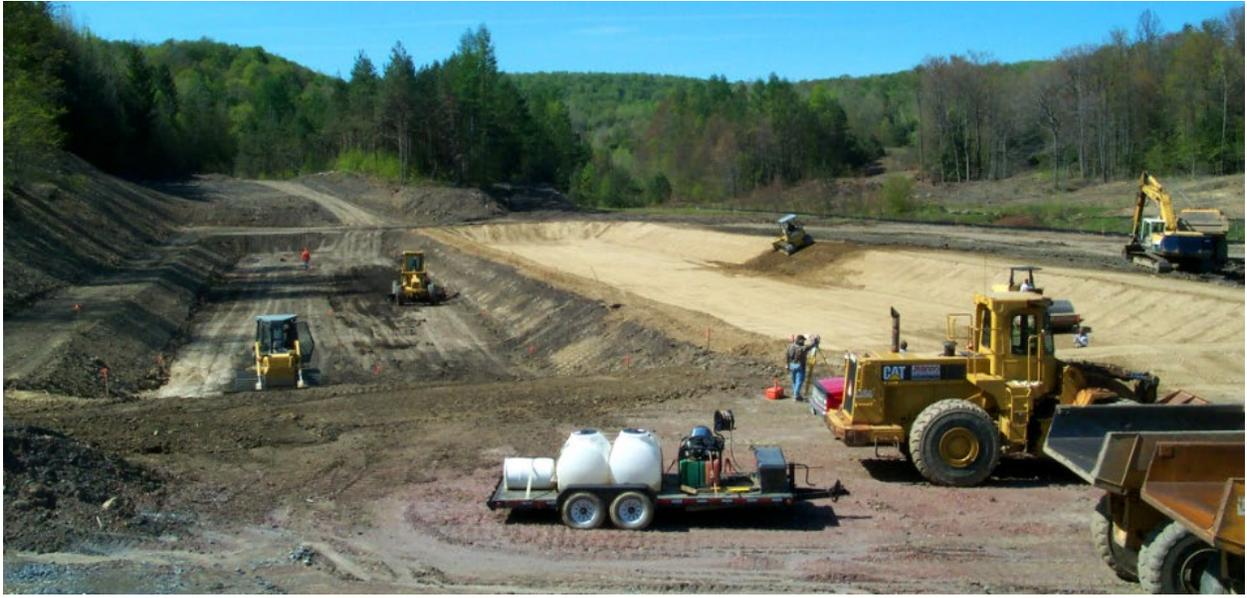
Figure 4: Installation of a clay liner during the construction of a VFP.
