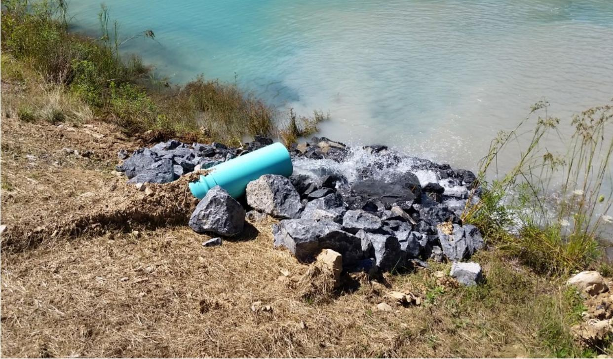
Figure 24 – Outlet protection structure designed to prevent channel erosion
