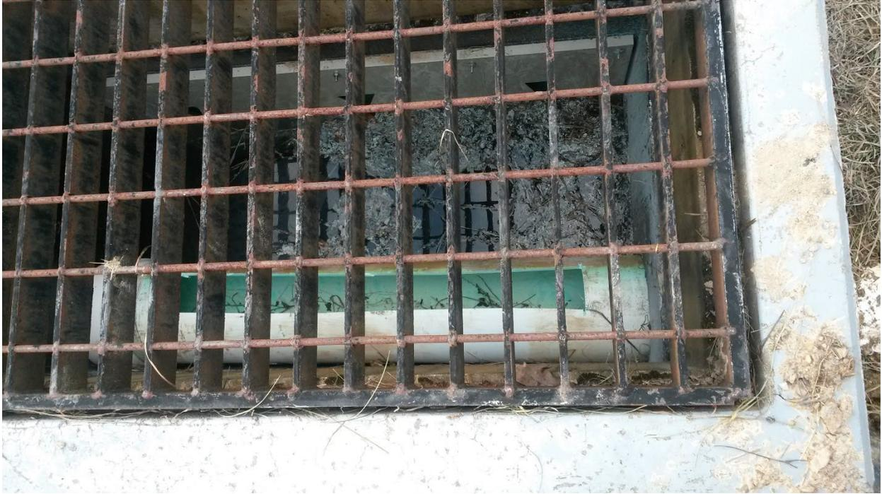
Figure 21 – Flow Splitter Box Installed with Orifice Plate to regulate Flow and Bypass Pipe to prevent Hydraulic Overloading of Treatment Cell
