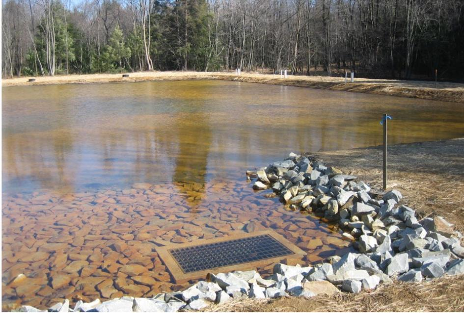
Figure 7: Newly constructed vertical flow pond. Inlet water control structure is shown. The reddish tint to the water in the background is due to low pH iron oxidation occurring on the top of the compost layer. Raw water pH is 2.8.
