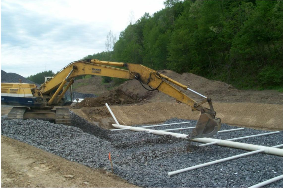
Figure 5: Excavator carefully covering the underdrain piping network (used for discharge and flushing) with limestone in preparation to construct a 3.0 ft thick limestone layer. A 1.5 ft thick compost layer will follow to finish the VFP. The excavator is covering a “spur” pipe. The spur pipes are connected to the larger “trunk” pipe oriented parallel to the bed. This is the type of piping configuration modeled in AMDTreat.
