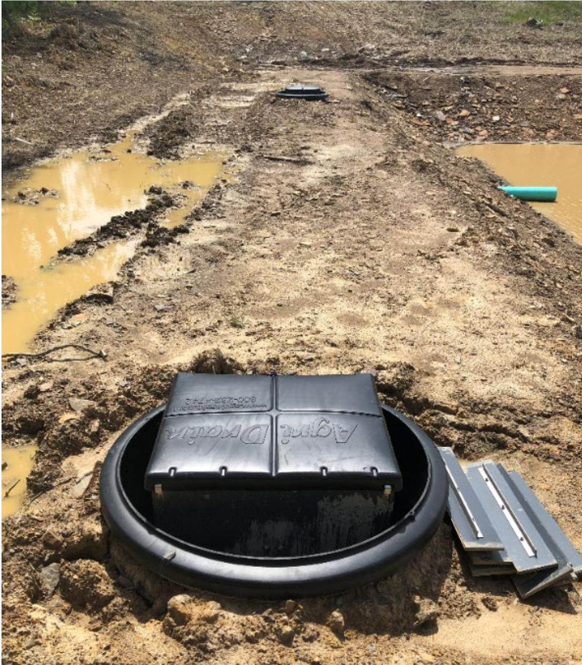
Figure 22 – Photo of Water Control Structure (Agri Drain brand) being installed into an embankment. The water control structure is placed inside a corrugated pipe to protect against soil pressure. Without protection, the box could deform and prevent operators from being able to adjust stop logs to control water level. Stop logs are removed and shown to the right of the corrugated pipe.
