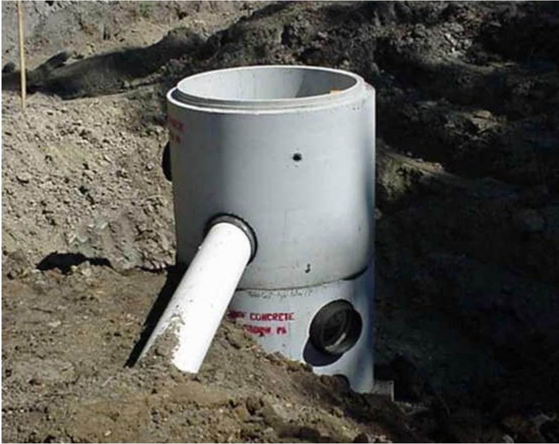
Figure 17. Flow distribution structure. A discharge is piped to the structure and the flow is distributed between three pipes that flow to three VFPs arranged in parallel.
