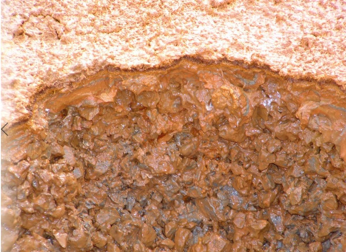
Figure 11. Close up photo of the 1.5 ft cross section of the Limestone Layer after removal of a thin and ineffective Compost Layer. Note the ½” layer of iron hydroxide on top of the Limestone Layer that caused hydraulic failure. In addition, iron hydroxide precipitate filled the void space within the 1 to 2” limestone fragments.
