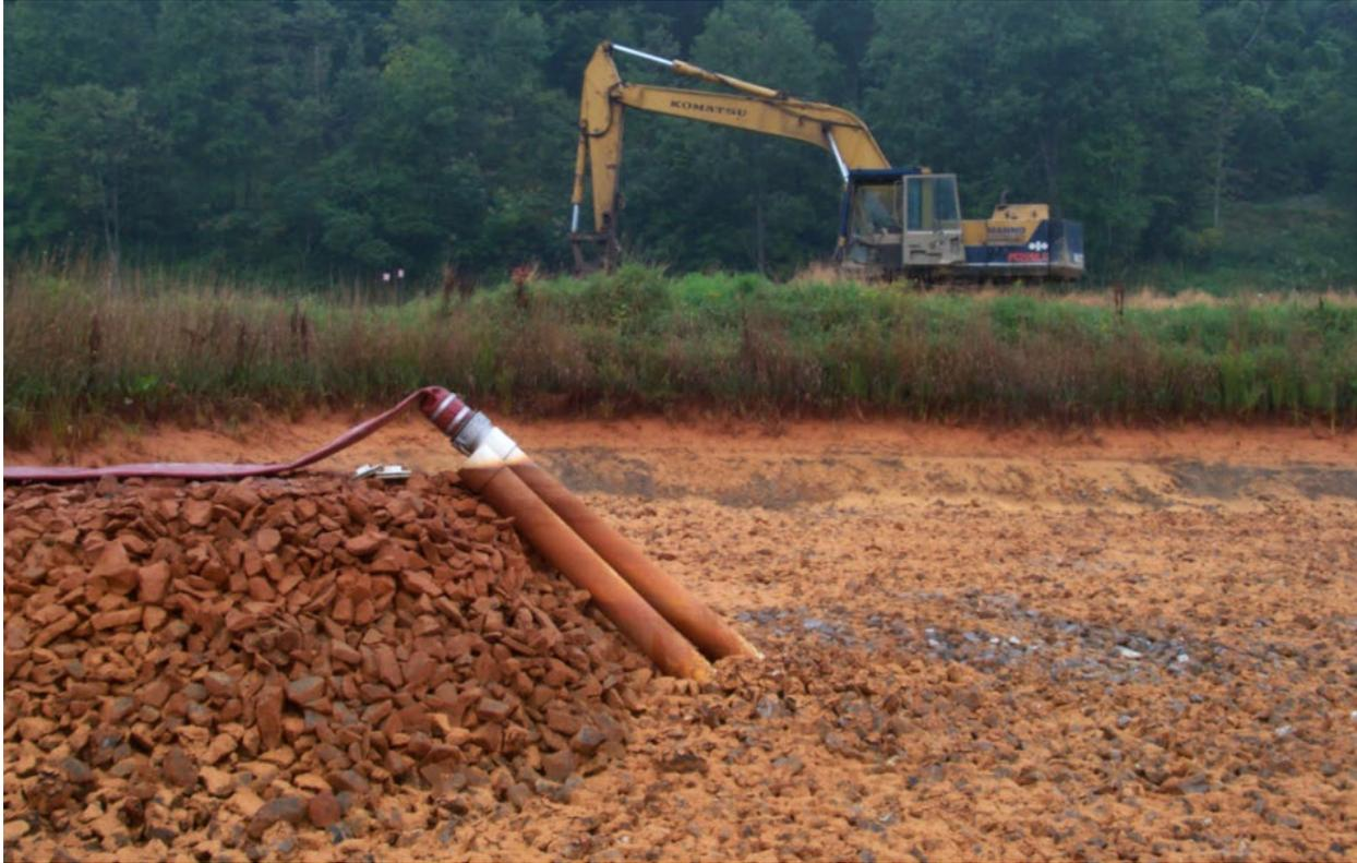
Figure 10. Photo showing the top of the Limestone Layer in a VFP after the compost layer was removed to perform an autopsy to identify the cause of failure. The 6 inch thick compost was insufficient to provide the retention time required to fully reduce the large ferric iron load to ferrous iron. Thus, the ferric iron oxidized and precipitated within the porosity of the limestone layer causing hydraulic failure. After this event, VFPs were designed with 12 to 18” of compost.
