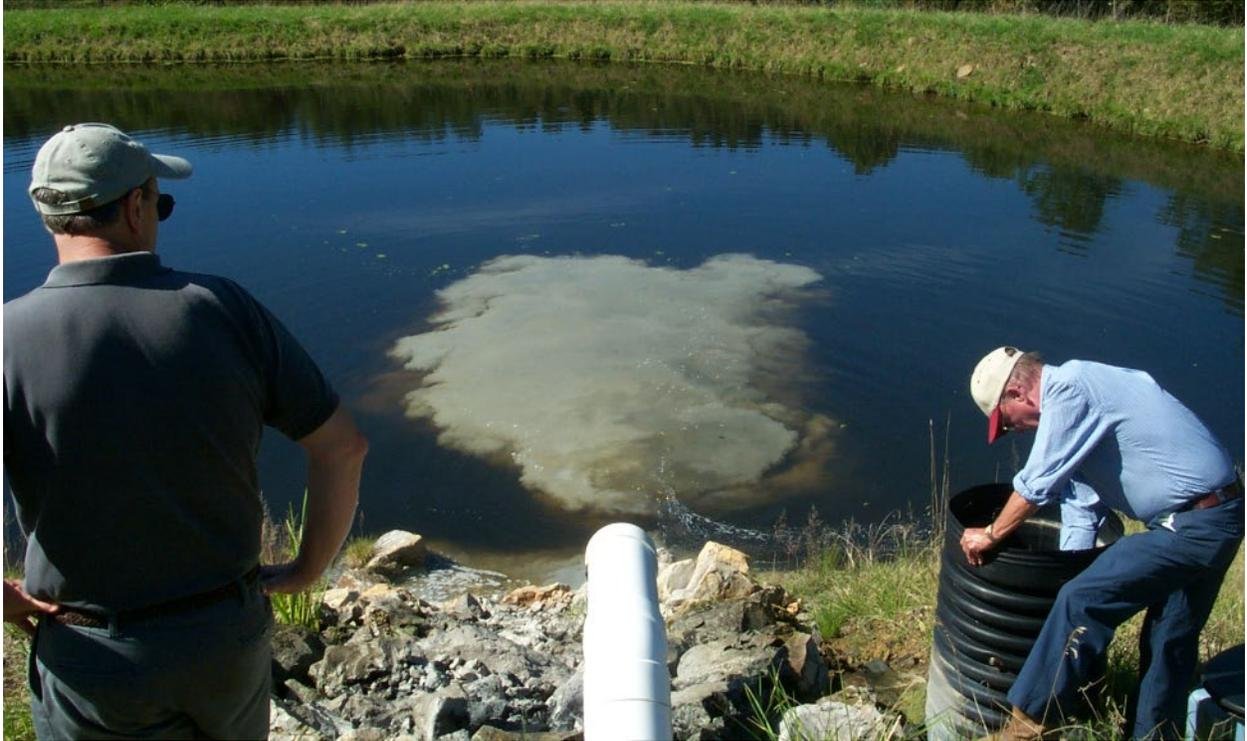
Figure 15. Gentleman on right turning a flush valve to flush a VFP. Note the flushing of the whiteish aluminum hydroxide precipitate.
