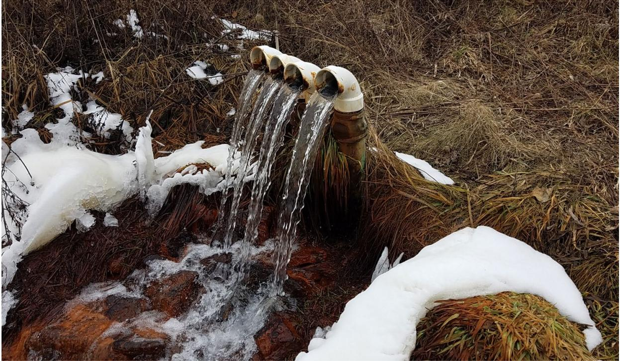
Figure 20: Several discharge pipes with Fernco Couplers to control discharge elevation (photo credit Tim Danehy of Biomost)
