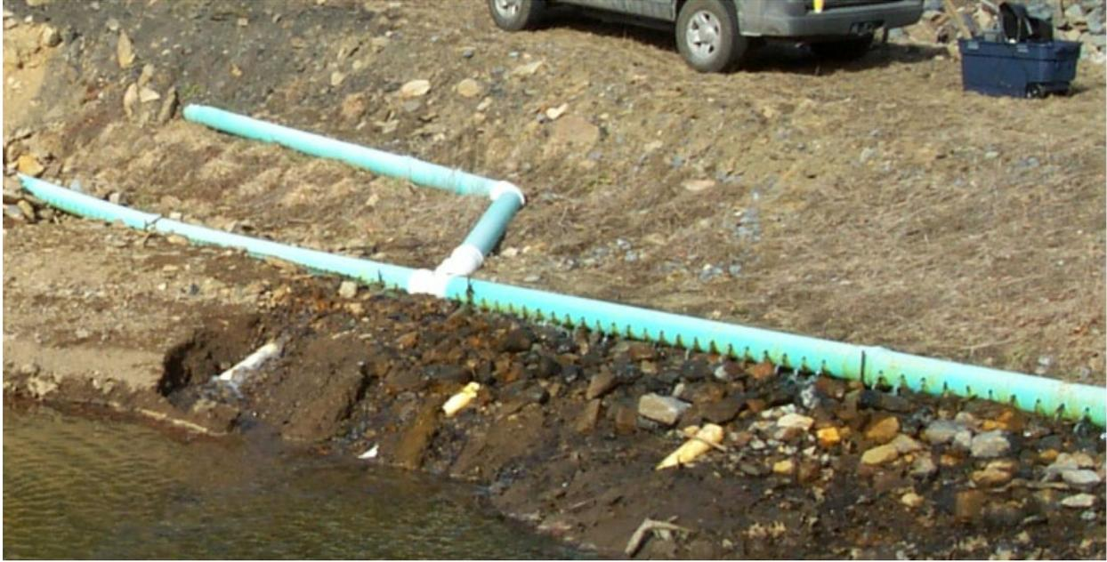
Figure 6: Influent piping configuration commonly used to distribute flow across the width of the wetland. A single pipe conveys mine drainage to the site and is connected to a perforated header pipe that extends the width of the wetland to promote uniform flow distribution.
