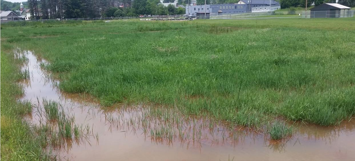
Figure 7: Wetland containing a short circuit (right hand side of photo) void of vegetation due to increased flow velocity. Water bypasses the interaction with wetland plants required for enhanced sedimentation. A sedimentation filter sock and a few bales of straw were used to block and divert water to the vegetated section of the wetland to allow wetland plants to establish in the channel. After a few months, the channel was fully vegetated.
