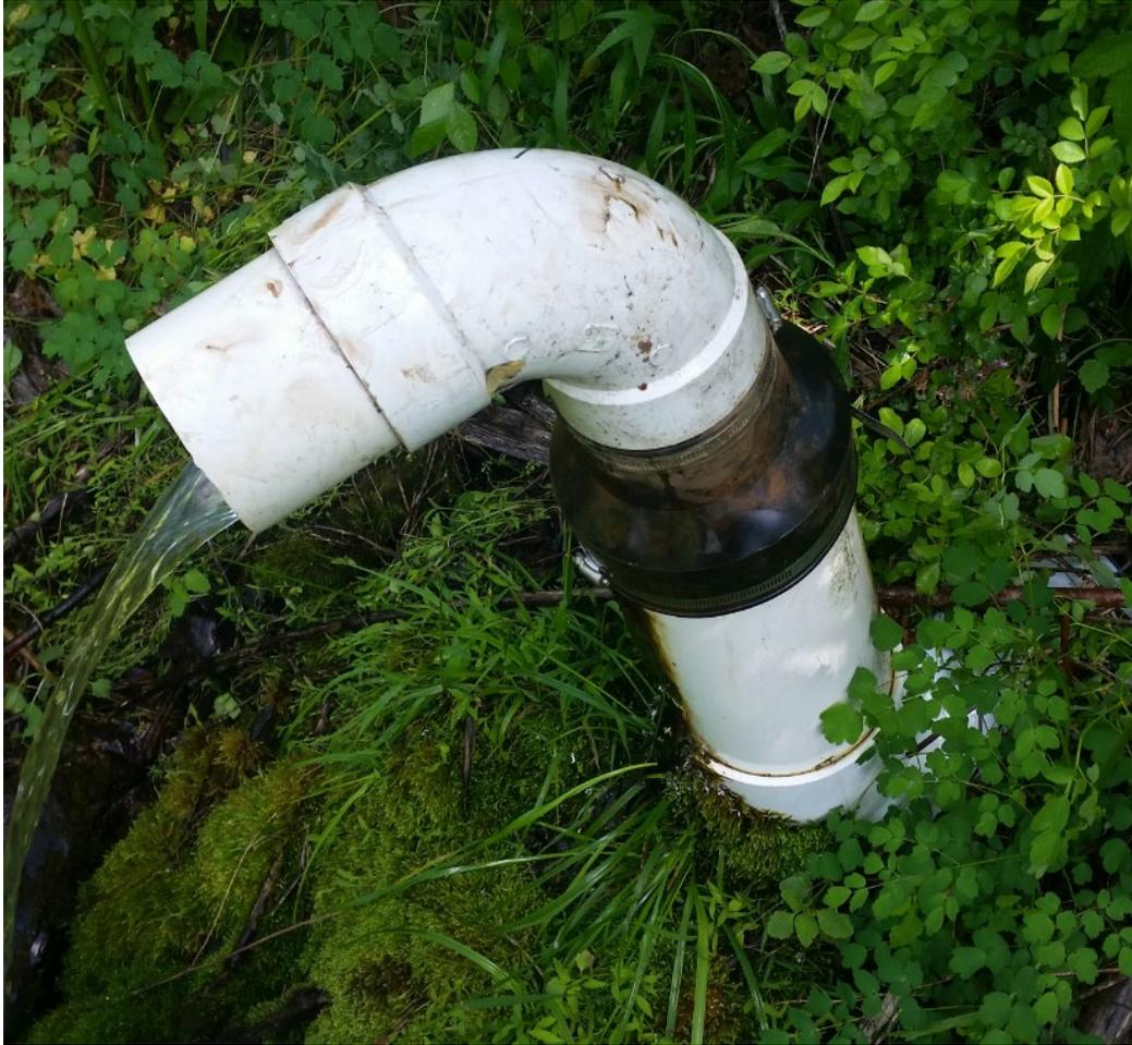
Figure 19: Discharge pipe from treatment system with Fernco Coupler. The Fernco coupler is the black rubber boot with two stainless steel bands used to tighten against PVC pipe to prevent leakage. The coupler has enough space that the upper elbow can be raised or lowered to change the discharge elevation (photo credit Tim Danehy of Biomost).
