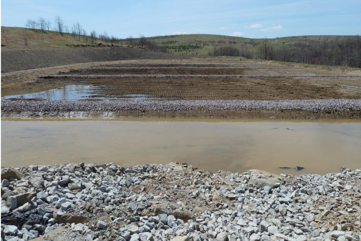
Figure 10: Installation of rock baffles with 80 ft spacing during construction of a 2.0-acre Wetland. Note darker colored soil layer in 2<sup>nd</sup>, 3<sup>rd</sup>, and 4<sup>th</sup> wetland cells.
