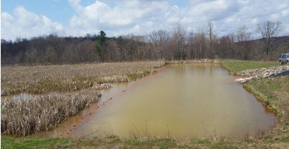
Figure 8: Water flows from the conveyance channel (right side of photo) into the inlet pool to promote flow distribution. The inlet pool is typically 3.0 ft deep to prevent the growth of wetland plants, capture suspended solids to protect vegetation, and to dissipate the energy of the water entering the wetland. Note the slightly submerged iron-coated rock apron that separates the inlet pool from the vegetation. The top of the rock apron level to promote even distribution of flow.
