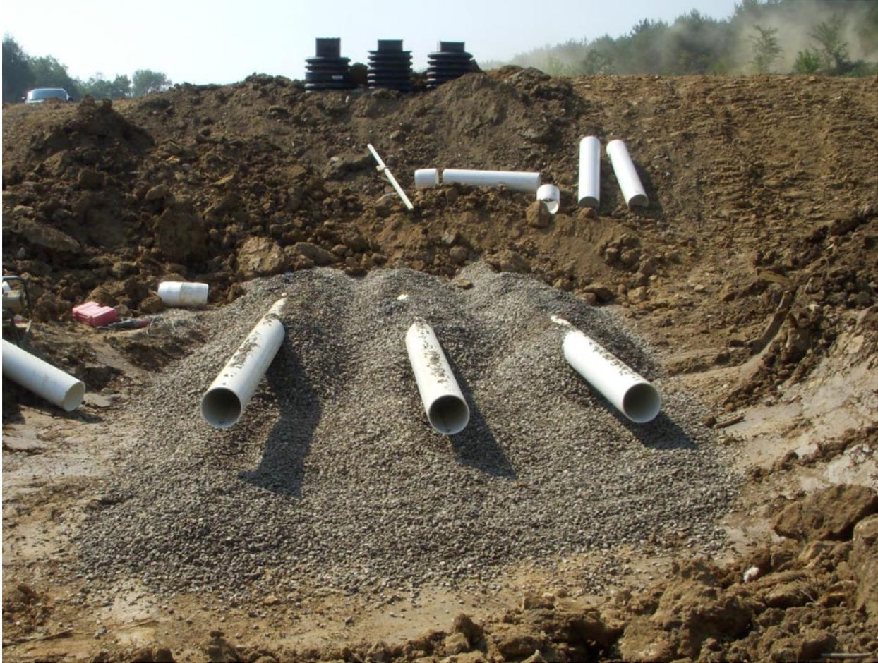
Figure 18: Three Agri Drain water control structures protected by black corrugated pipe. This is not installed into a Wetland. The photo is being used to show how Agri Drain boxes are protected by corrugated pipe.
