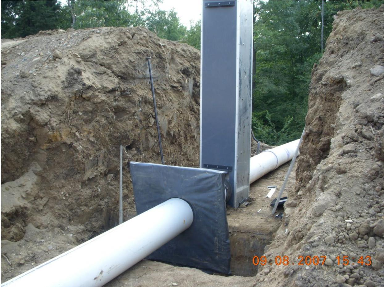
Figure 17: Agri Drain water control structure and anti-seep collar to prevent leakage around pipe that extends through embankment. Note the collar is “keyed” into the base of the embankment.
