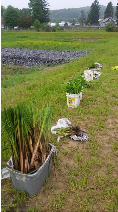
Figure 24: A variety of wetland plant plugs for manual planting.
