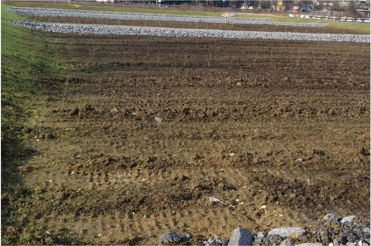
Figure 25: Wetland just after seeding and manually planting wetland plant plugs. A small amount of water (no more than 0.5 ft) will be added to wetland to promote seed germination and plug growth.
