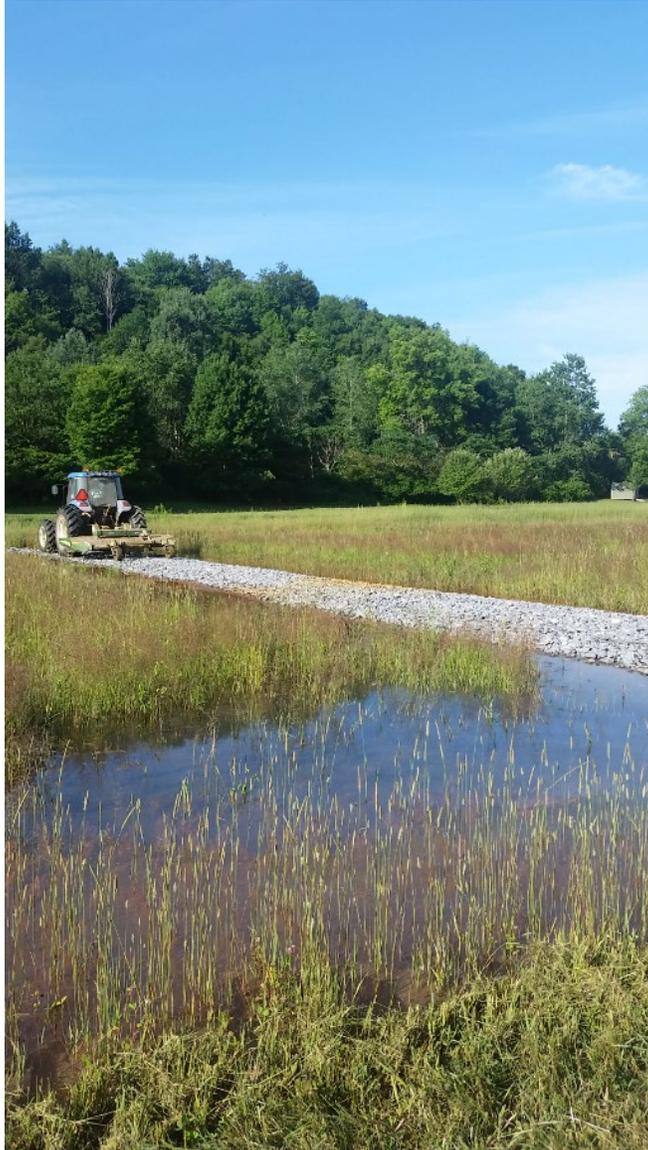
Figure 11: Wetland rock baffle used to transport tractor mower across Wetland
